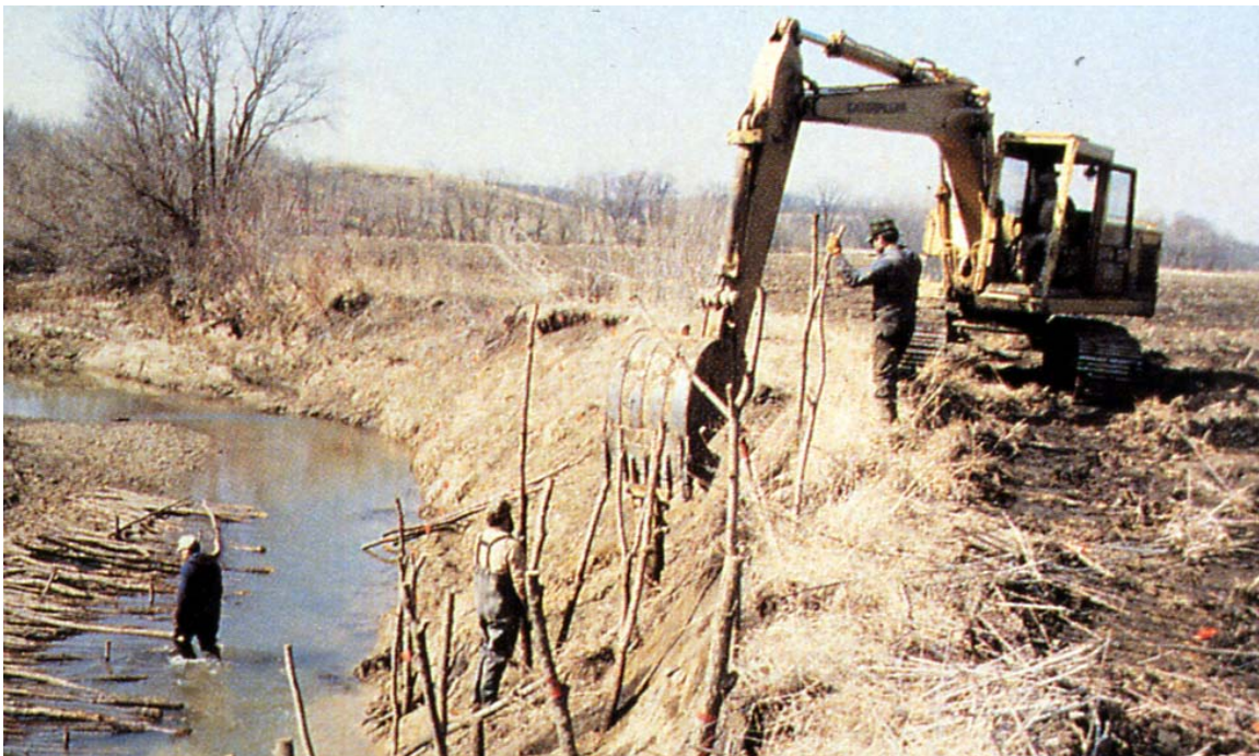
12 D Photo: Mechanical installation of willow or cottonwood posts. Illinois Water Survey
