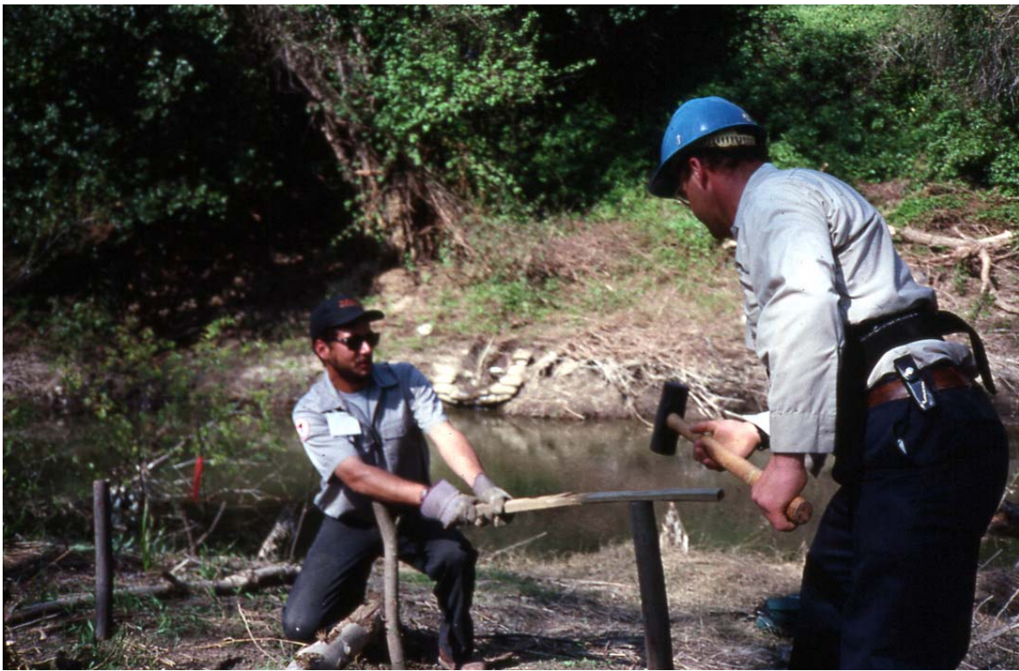
12 C Photo: Installing a willow or cottonwood post by hand.
