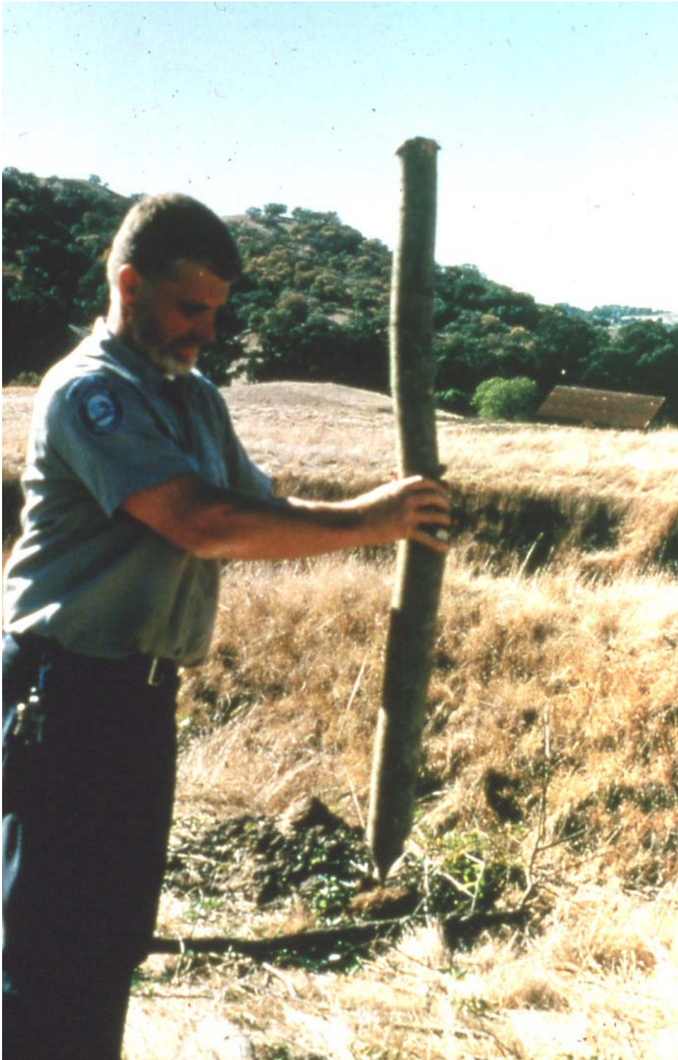
12 B Photo: Willow Post. Note planting end has been pointed for easy installation.
