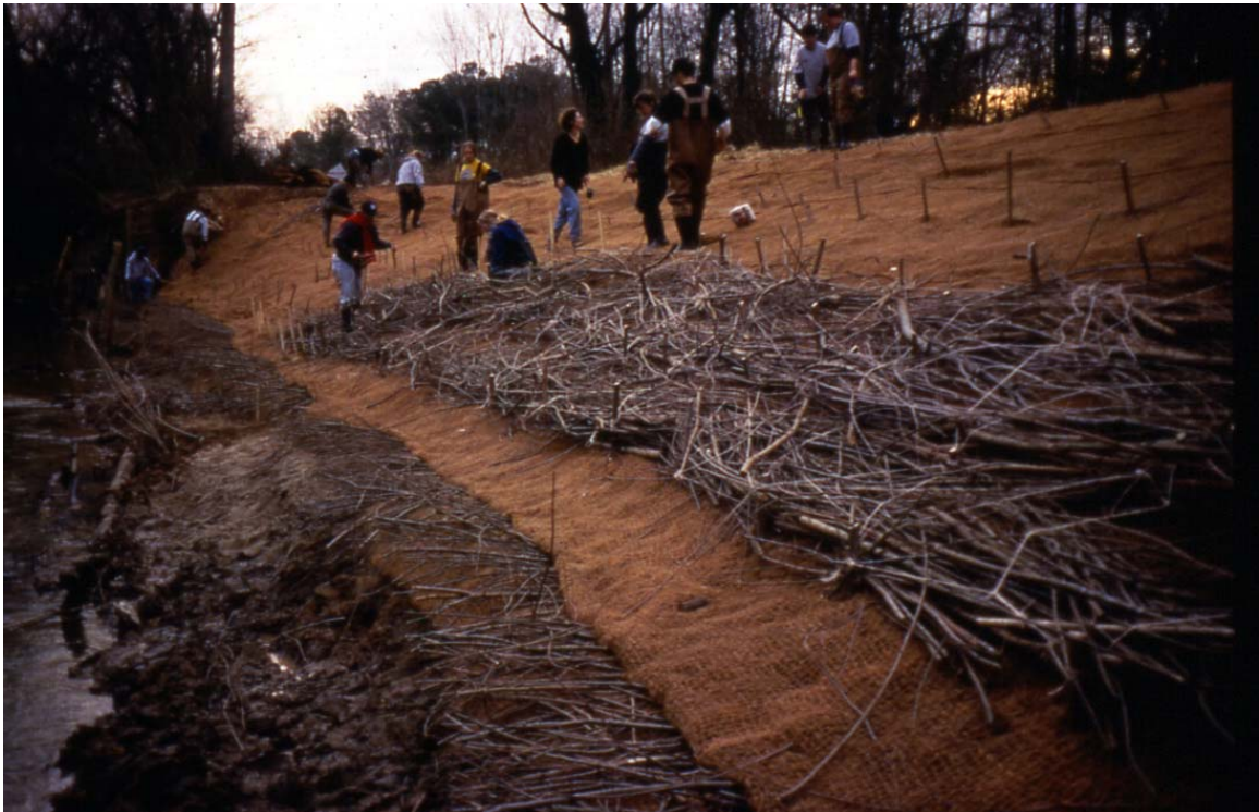
Figure 14C. Brush and Post Installation
