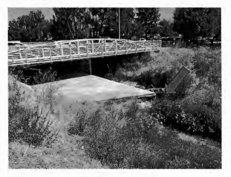
Figure 6B: View of erosion upstream of Los Coches Street
