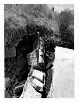
Figure 6A: Erosion upstream of Los Coches Street
