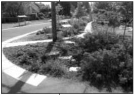
Seattle SEA Streets Project. Graded swales with amended soils reduced stormwater volume by 97 percent for two consecutive years. Utilities (SPU) staff are developing prototype "Natural Drainage System" projects to meet multiple goals within street rightof-ways. These goals include infiltrating and slowing stormwater flow, filtering pollutants by soils
