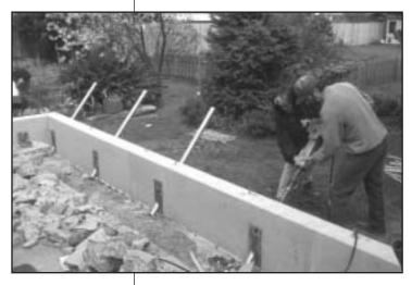
Homeowners in Olympia install a Low Impact Foundation Technology (L.I.F.T.) system as an alternative to a conventional foundation.
