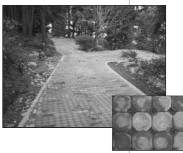
The pervious paver system replicates natural stormwater infiltration, provides treatment and eliminates the need for conventional detention/ treatment systems.
