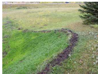
Blanket Installation and Result
