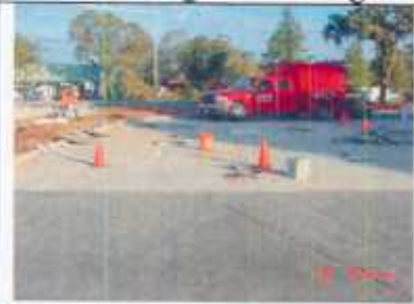
South looking North at Tank Pit
