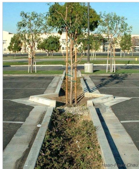
A vegetated swale with curb cuts in the parking lot of a shopping center at 8500 Firestone Blvd., Downey, CA.
