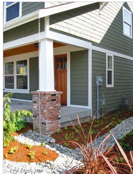
Rain chains guide water into rocky infiltration swales in Seattle's High Point neighborhood.
