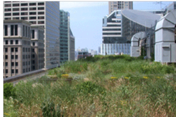
Chicago's green roof on City Hall
