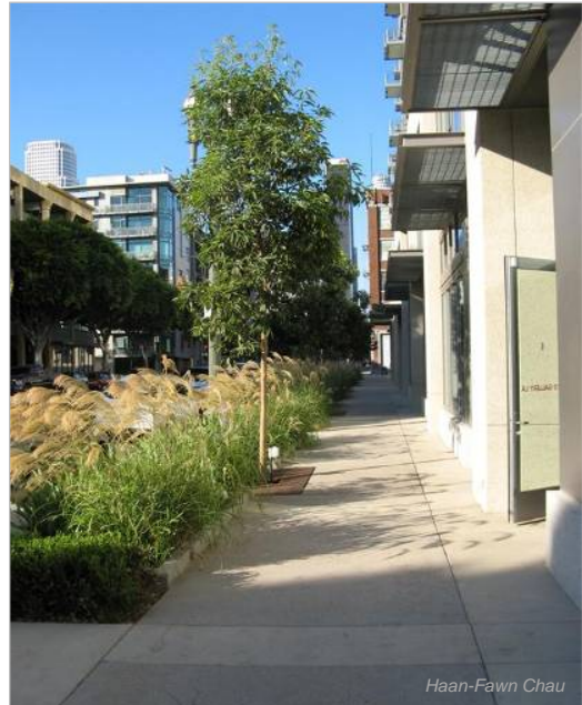
Bioswales and tree wells along 1100 S. Hope Street in downtown Los Angeles
