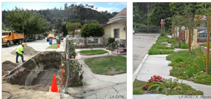
Oros Street during and after “green street” reconstruction.
