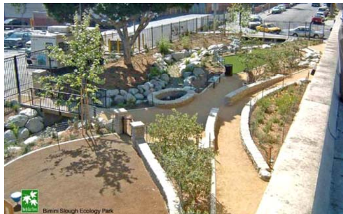
Bimini Slough Ecological Park, created by North East Trees in East Hollywood, daylights an existing storm drain and provides on-site stormwater management. Credit: North East Trees
