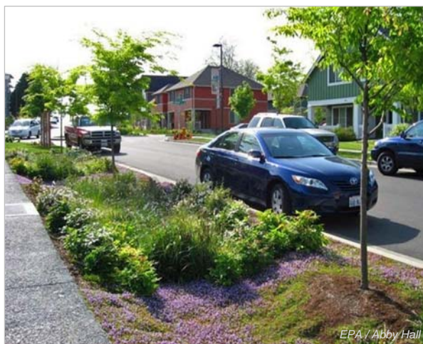
Seattle’s SEA Street (Street Edge Alternatives) project includes bioswales and permeable pavement.
