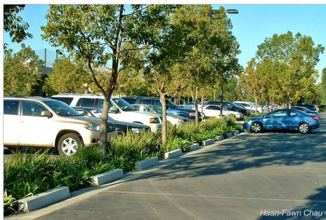
A vegetated swale with curb cuts collects runoff at the RioHondo Golf Course in Downey, CA.
