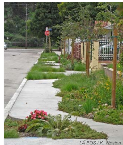
Oros Street after its "green street" reconstruction (Los Angeles)
