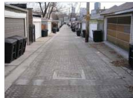
Permeable alley during construction and after completion in Chicago.
