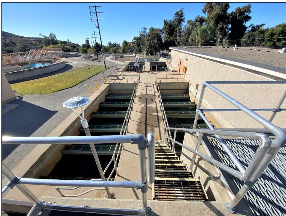
Photograph 18: Overview of filter structure, showing four filter bed; camera facing west, November 16, 2022.
