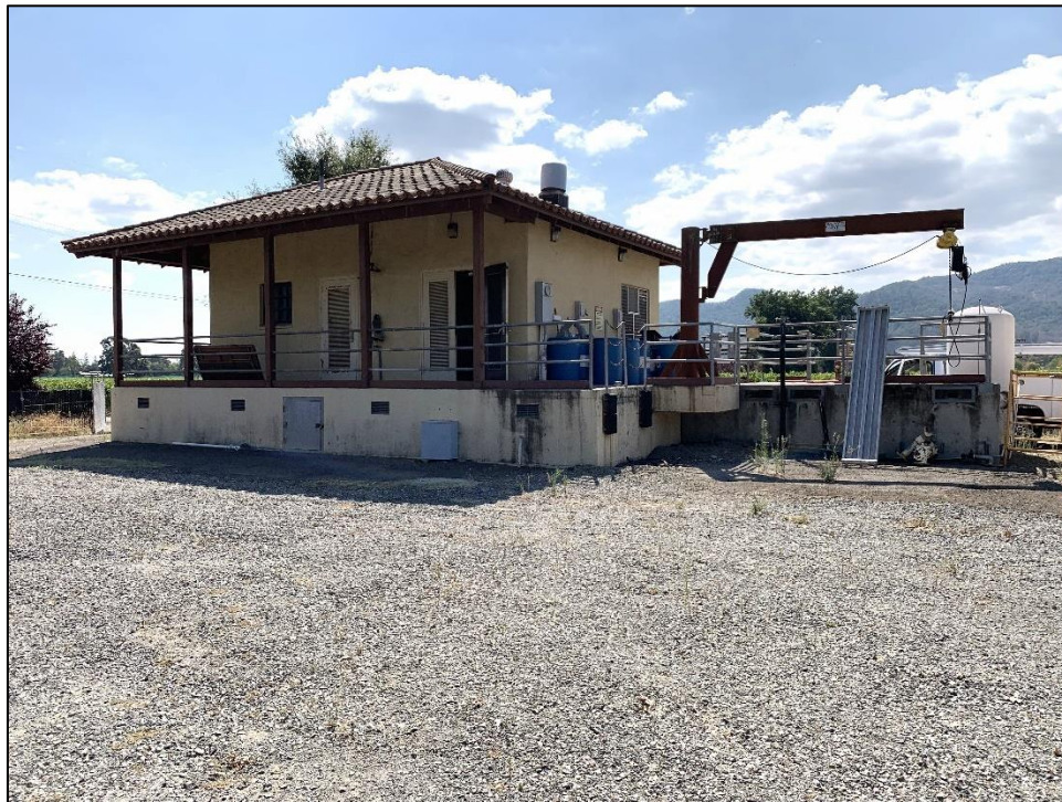
Photograph 29: East side of control building with pump station to right, camera facing west, September 15, 2022.
