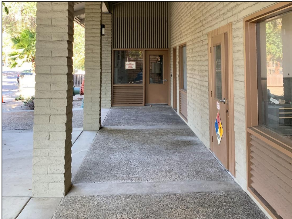
Photograph 7: West side fenestration; facing north, October 13, 2022.
