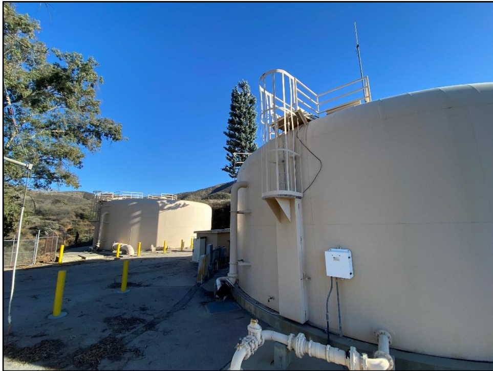
Photograph 24: Storage reservoirs, camera facing southeast; November 16, 2022.
