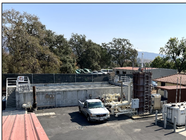
Figure 102: Raised chlorine contact basin (JRP photograph, September 15, 2022).
