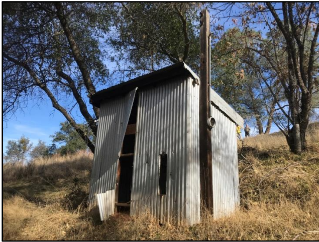
Photograph 14. Electrical shed, west and south elevations. View northeast.
