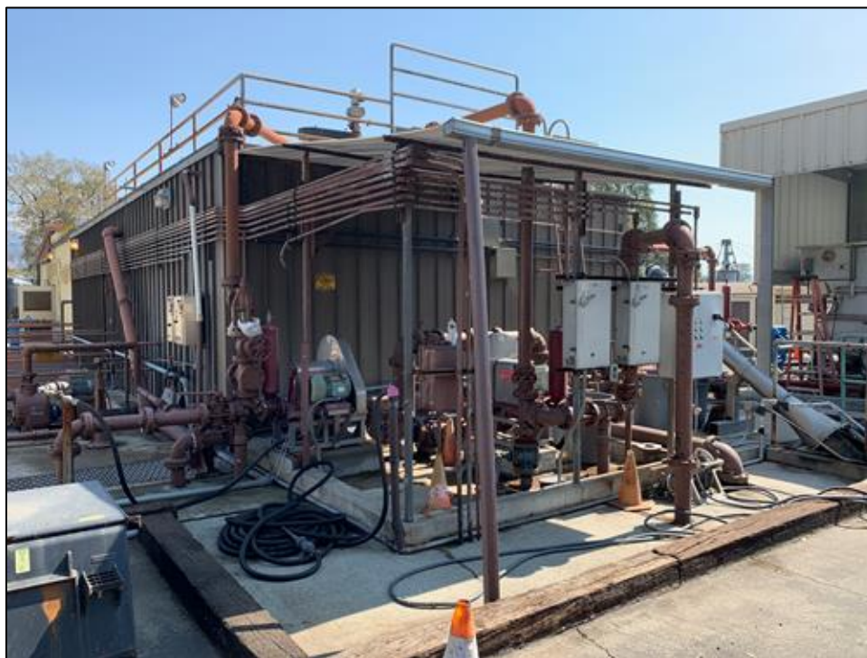
Photograph 22: Rear of sludge digester, camera facing east, September 15, 2022.
