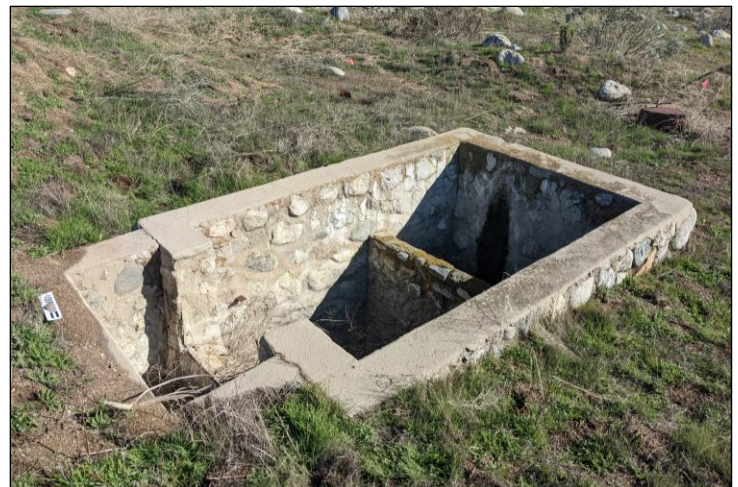
Photograph 11. Concrete and cobble rectangular vault (Feature 14), camera facing northeast (12/13/2022).
