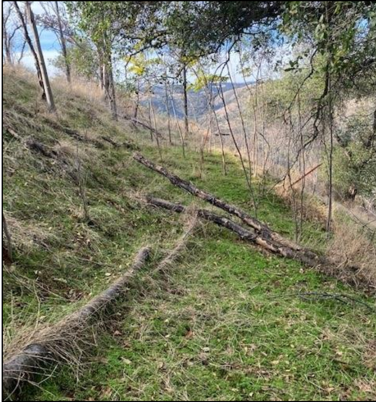
Photograph 19. Leach Field #5 with overgrown supply pipe looking similar to the nearby fallen trees. View northwest.
