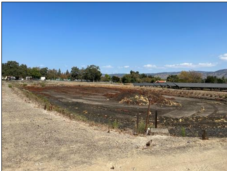
Photograph 25: Sludge drying beds, camera facing north, September 15, 2022.
