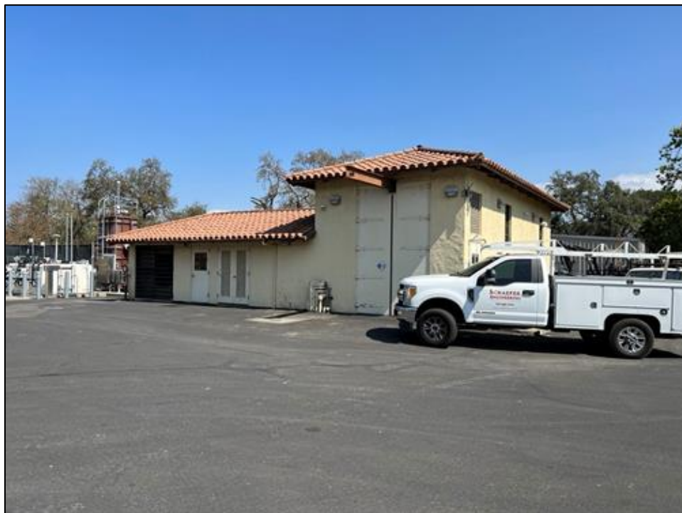
Photograph 3: Control building, southwest corner, camera facing north, September 15, 2022.
