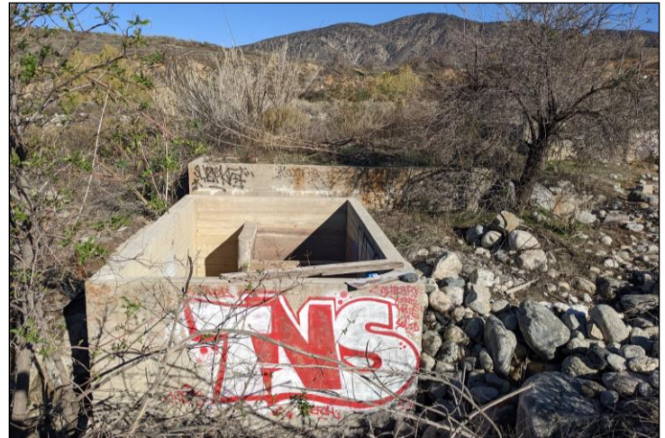
Photograph 10. Weir box (Feature 1), camera facing north (12/8/2022).
