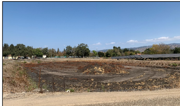
Figure 107: Sludge bed scraped and prepared for disposal (JRP photograph, September 15, 2022).
