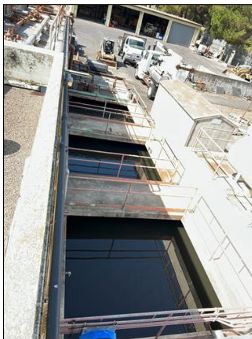
Photograph 11: View from above clarifier tanks, camera facing west, September 15, 2022.
