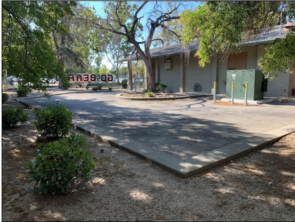
Photograph 14: Landscaping at rear of building; facing southwest, October 13, 2022.
