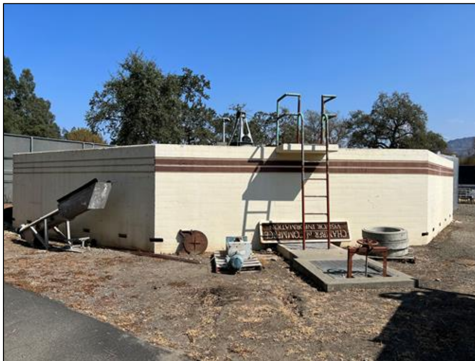
Photograph 13: Trickling filter, camera facing north, September 15, 2022.
