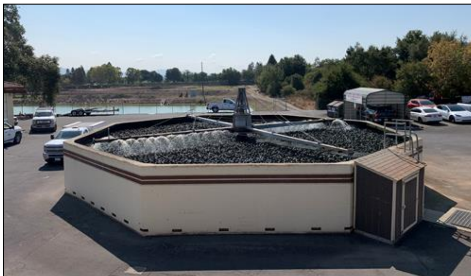
Photograph 12: Trickling filter, camera facing south, September 15, 2022.
