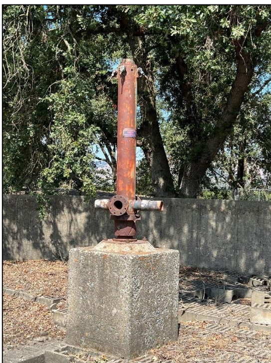
Photograph 27: Central hub and inlet pipe for trickling filter, showing Pacific Flush-Tank Company brand; camera facing east, September 15, 2022.
