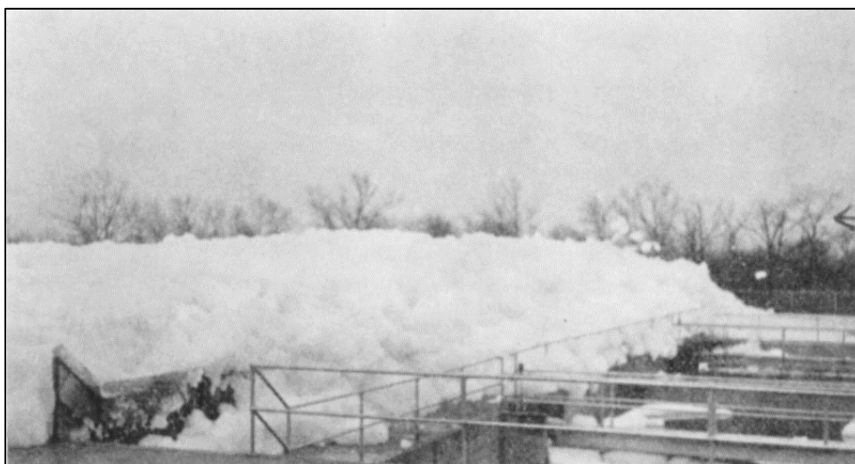
Figure 57: Foaming at an activated sludge plant attributed to synthetic detergents. 276
