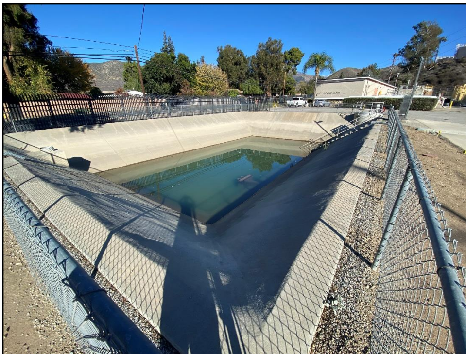
Photograph 23: Washwater recovery basin, camera facing northeast; November 16, 2022.
