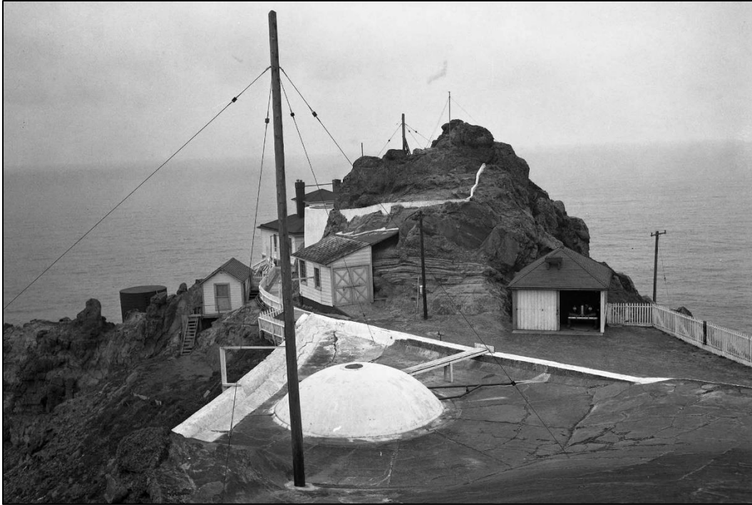
Figure 84: Cistern and 6,000-square-foot concrete watershed at Point Reyes Light Station. 343
