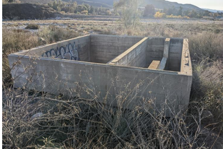
Photograph 2. Weir box (Feature 31), camera facing southwest (12/13/2022).
