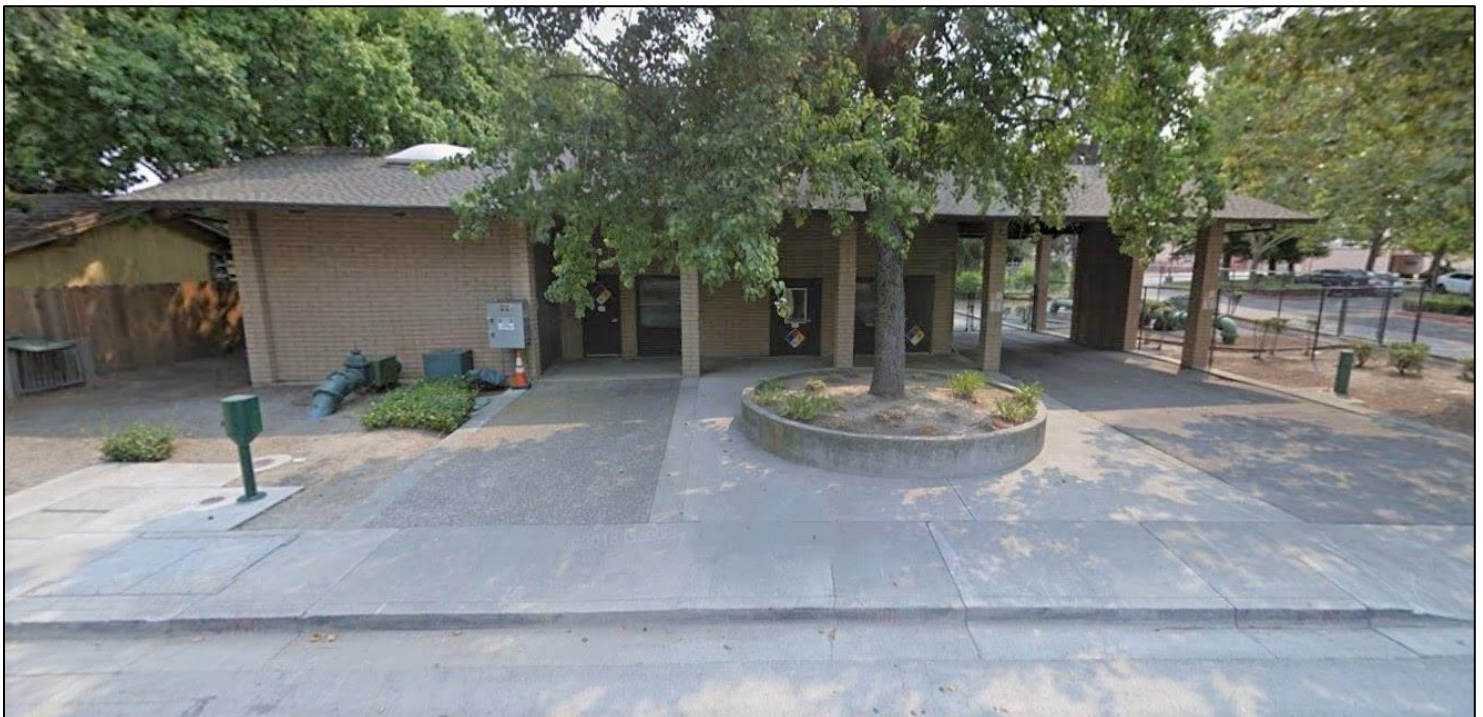
Photograph 3: An August 2018 Google Streetview image shows the treatment building and porte-cochère; facing east. Foliage on the front tree prevented an unobstructed full view of the building at the time of recordation in 2022.
