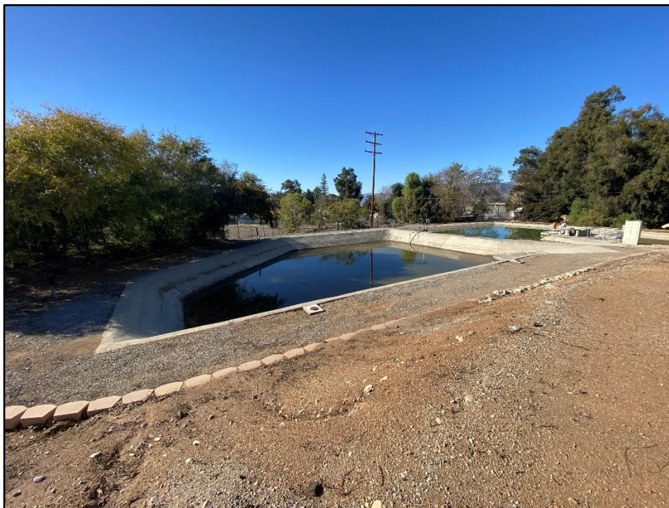
Photograph 22: Sludge pond; camera facing northwest; November 16, 2022.
