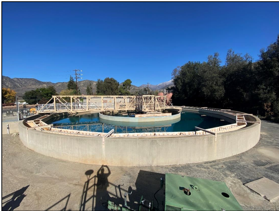
Photograph 15: Clarifier, camera facing northeast; November 16, 2022.
