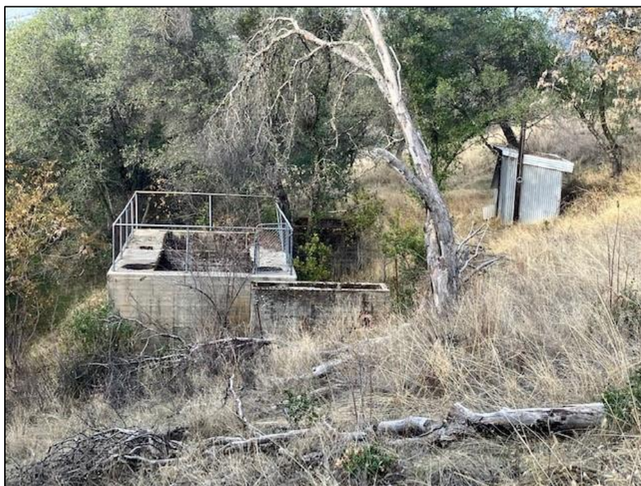
Figure 110. Overview of the 1947 Mokelumne Hill Sanitary District Treatment Plant.
