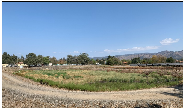
Figure 106: A sludge bed with material from prior year (JRP photograph, September 15, 2022).
