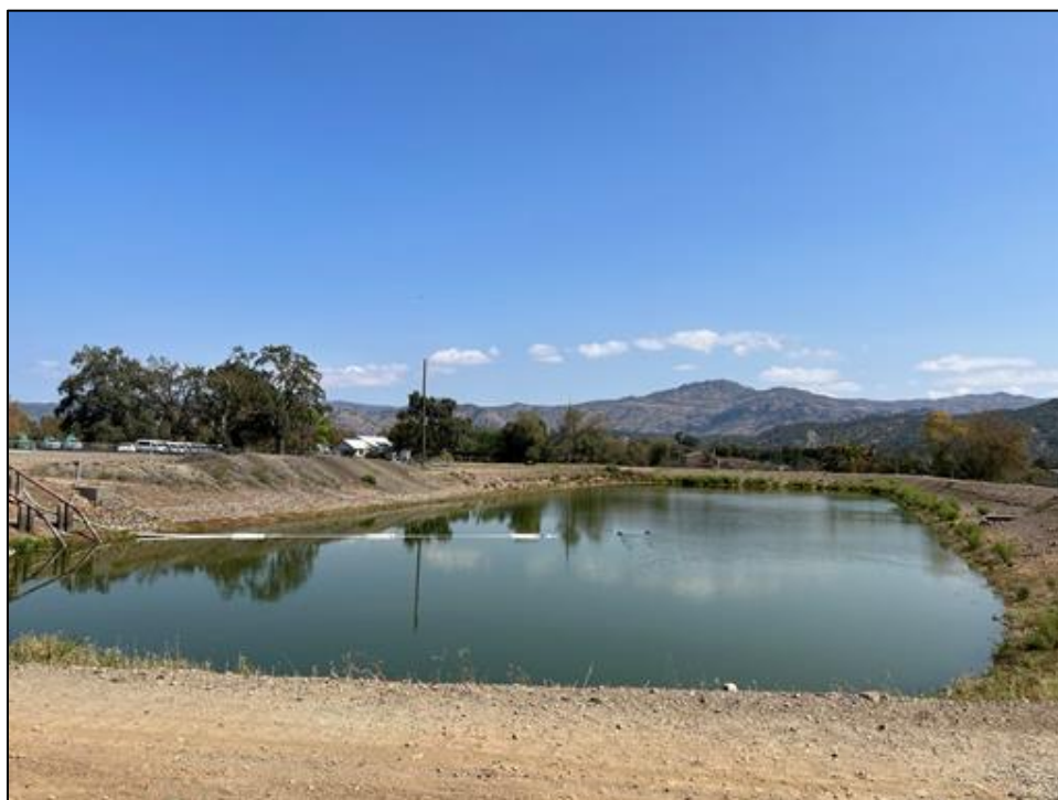
Photograph 21: Flow equalization pond, camera facing northwest, September 15, 2022.
