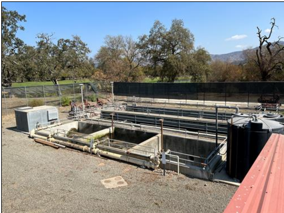
Photograph 15: Activated sludge tanks with final clarifier behind, camera facing northeast, September 15, 2022.
