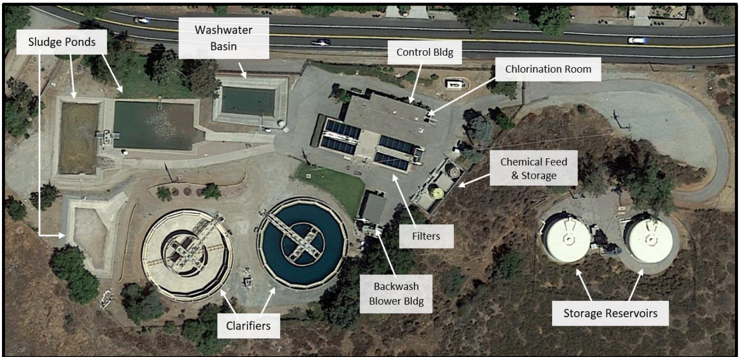
Henry Tate Water Treatment Plant Google Earth imagery, August 5, 2021 Annotated by JRP
