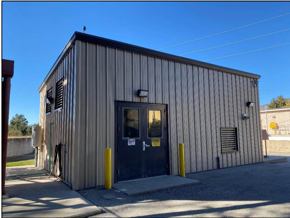
Photograph 20: Southeast corner of modern blower building, camera facing northwest; November 16, 2022.
