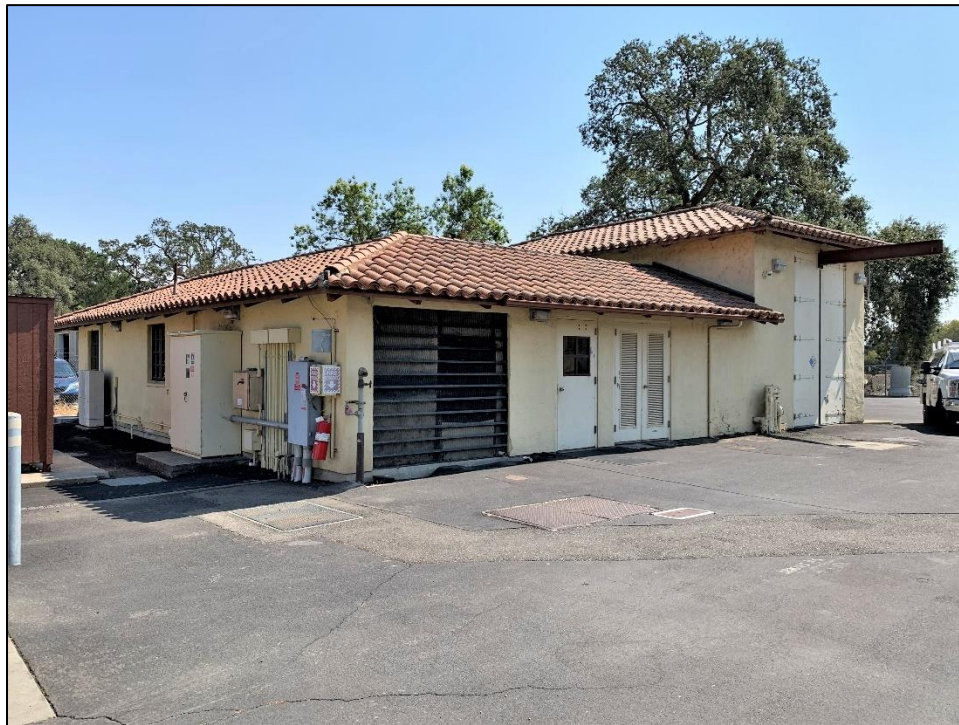
Photograph 2: Control Building, northwest corner, camera facing east, September 15, 2022.
