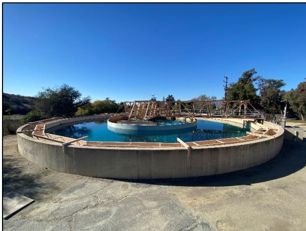
Figure 73: A circular clarifier (JRP photograph, November 17, 2022).
