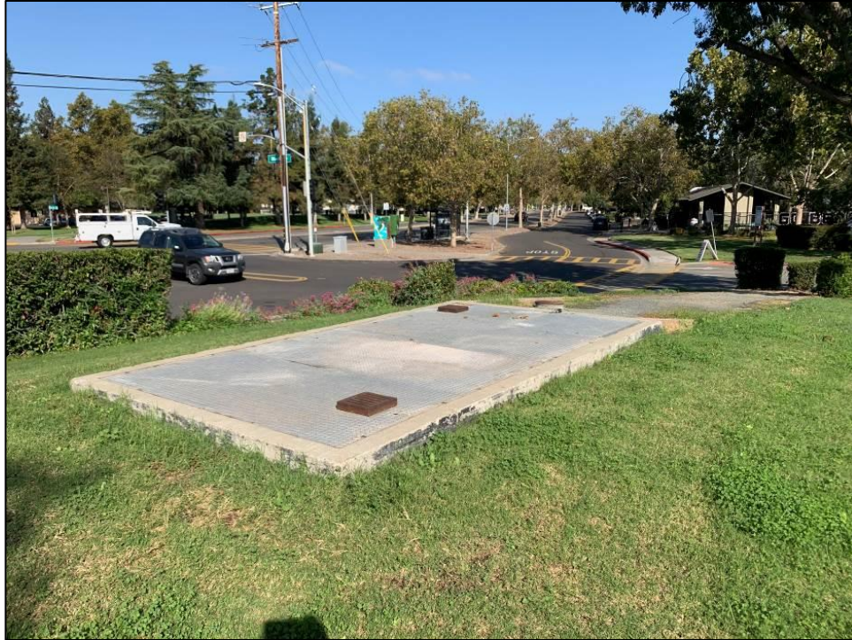
Photograph 2: Well 5 vault; facing north by northwest, October 13, 2022.
