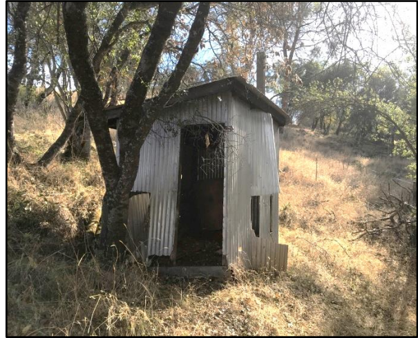
Photograph 15. Electrical shed, north elevation.
