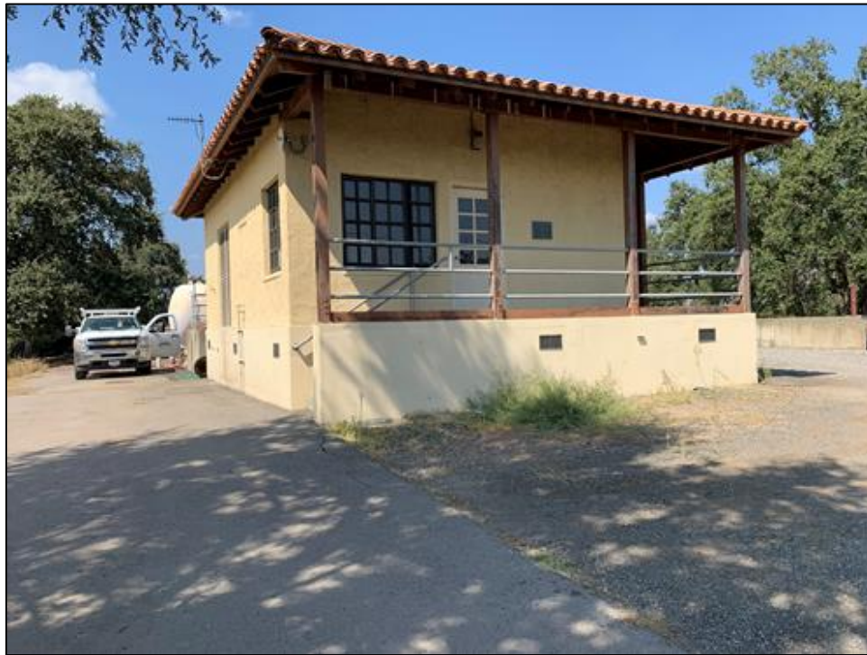
Photograph 28: Pumping station control building, camera facing north, September 15, 2022.
