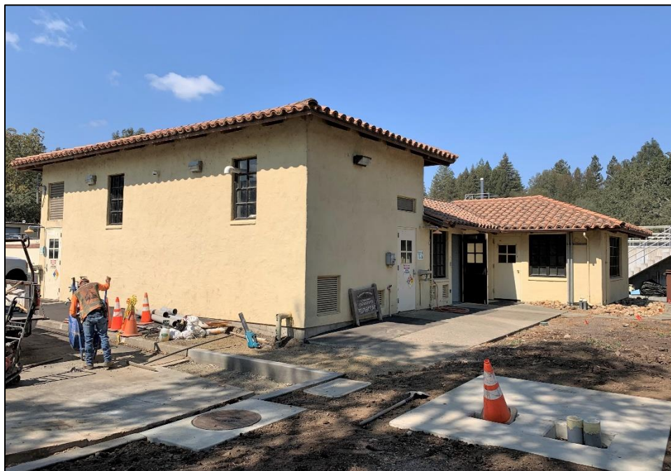
Photograph 4: Control building, south and rear east side, camera facing northwest, September 15, 2022.
