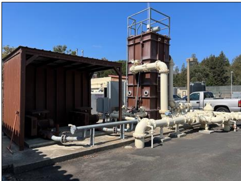
Photograph 18: Fuzzy filter, camera facing northwest, September 15, 2022.
