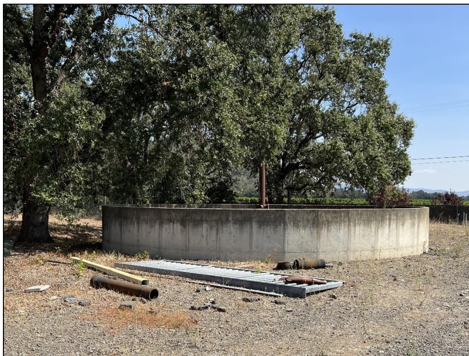
Photograph 26: Trickling filter shell at pump station; camera facing east, September 15, 2022.
