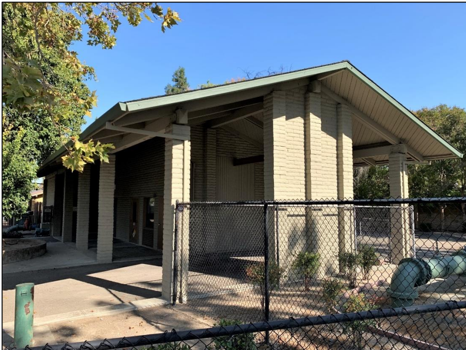
Photograph 5: Partial wall and columns supporting the porte-cochère roof; facing north, October 13, 2022.
