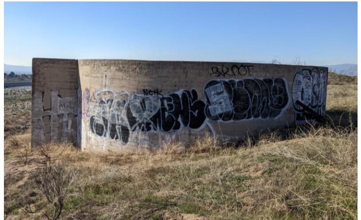
Photograph 5. Surge tank (Feature 8), camera facing west (12/8/2022).
