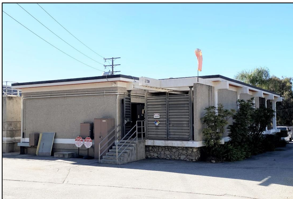
Photograph 3: Northeast corner of control building showing chlorine room entrance; camera facing southwest; November 16, 2022.
