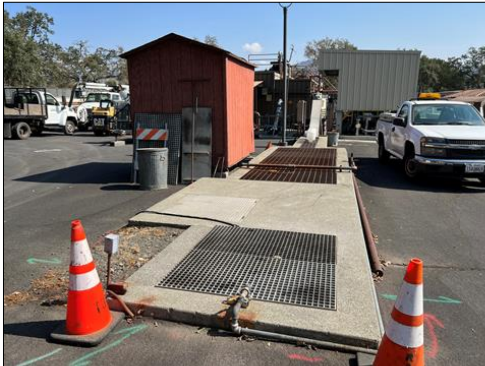
Photograph 6: Grit chamber with shed for aeration equipment, camera facing east; September 15, 2022.
