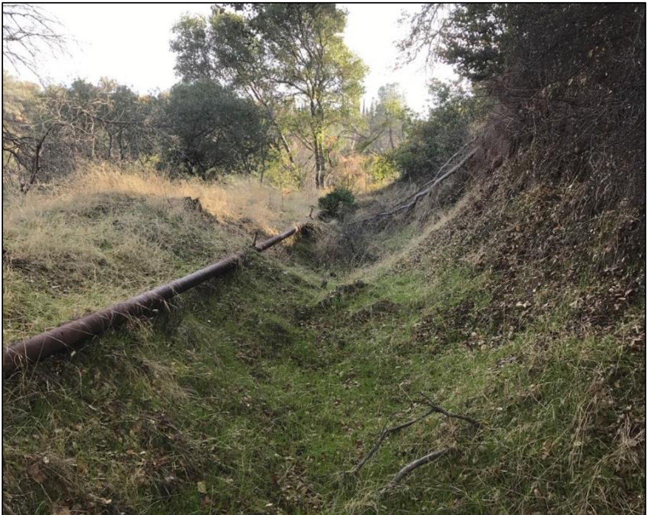
Photograph 18. Leach Field #2 with supply line pipe and distribution heads. View northeast
