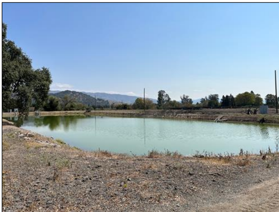
Photograph 20: Effluent storage pond, camera facing east, September 15, 2022.
