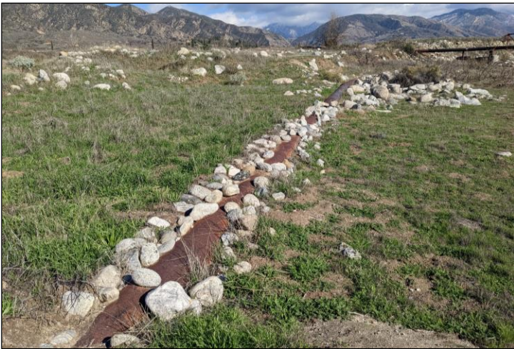
Photograph 13. Metal pipeline with concrete lining (Feature 18), camera facing northeast (12/13/2022).
