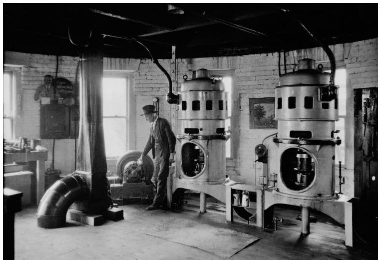
Figure 32: Interior of Los Angeles sewer pump station showing two electric motors. The pumps were housed in a lower, below-ground level. 206
