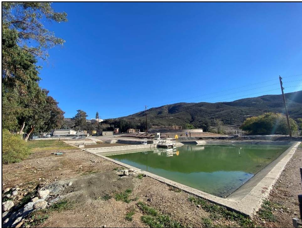
Photograph 21: View of sludge pond basins, camera facing southeast; November 16, 2022.
