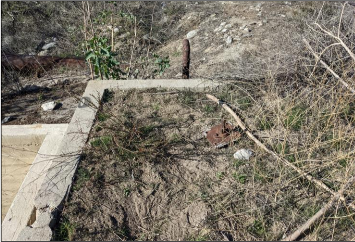
Photograph 8. Cinderblock-topped structure (Feature 4), camera facing west (12/8/2022).
