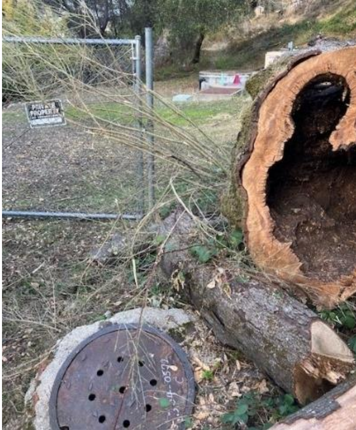
Photograph 3. Access cover to western intake main located at 8514 Center Street, east of the Protestant Cemetery. chamber ( Photographs 1 and 10 ).
