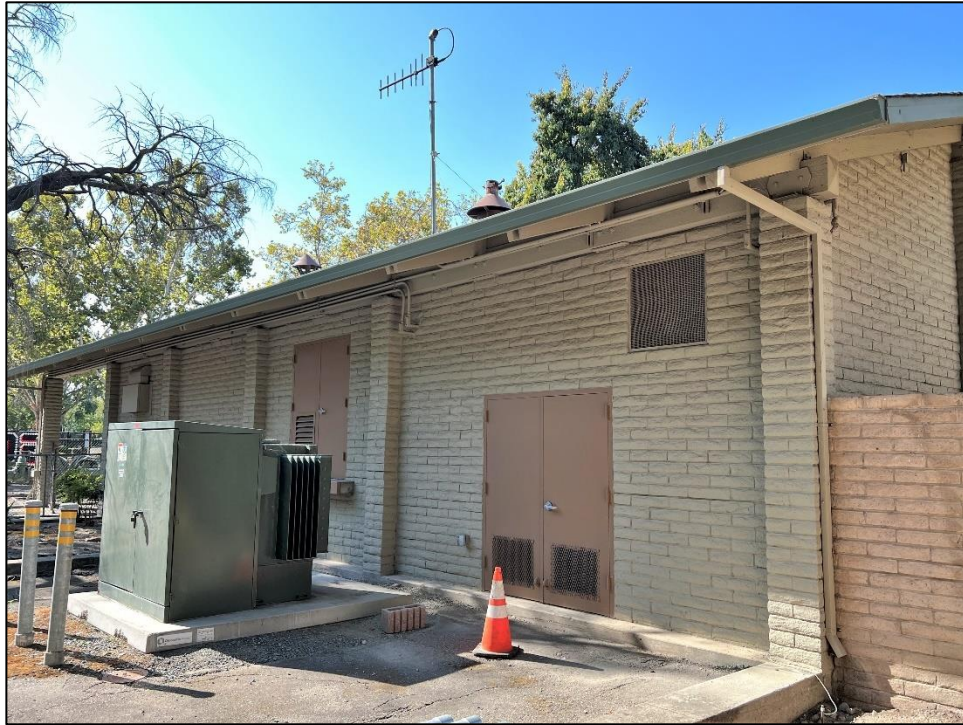
Photograph 6: Rear east side showing irregularly spaced pilasters; facing southwest, October 13, 2022.
