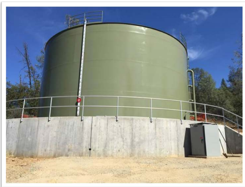
One of the many upgrades at the Lewiston Community Services District was the installation of this new water storage tank.
