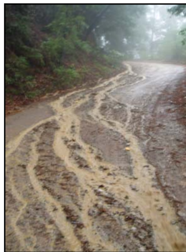
Erosion from rural roads in Santa Cruz County contributes significant quantities of sediment to impaired TMDL listed watersheds.
