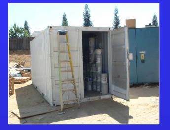
Store chemicals in watertight containers or in a completely enclosed structure
