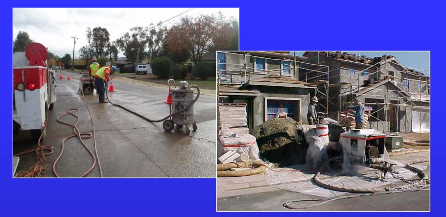
Contain and protect waste material from wind and rain at all times
