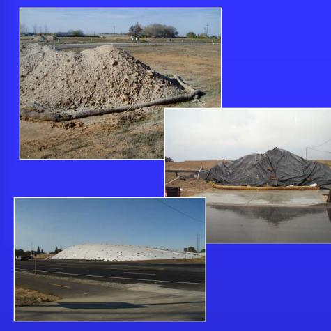
Cover and berm stockpiled construction material when not in use (soil, spoils, aggregate, fly-ash, stucco, hydrated lime, etc.)
