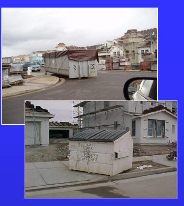
Prevent discharge from waste disposal containers to storm drains or receiving waters. Cover waste containers at the *end of every business day* and during rain events.
