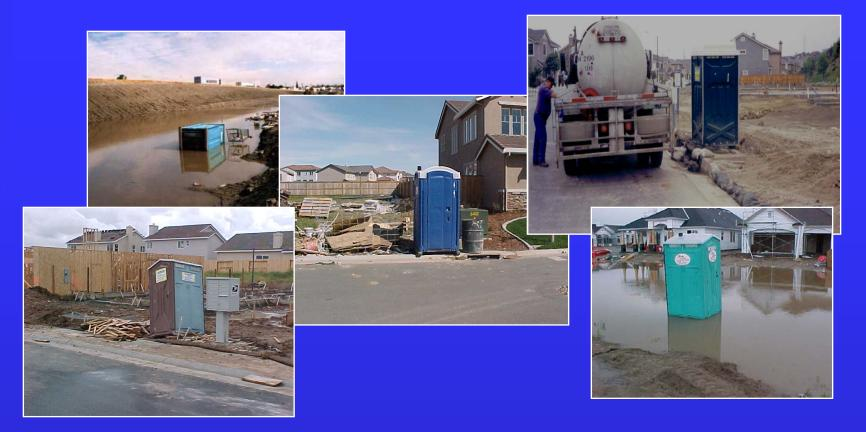
Contain "sanitation facilities" to prevent discharge to storm drains or receiving waters.
