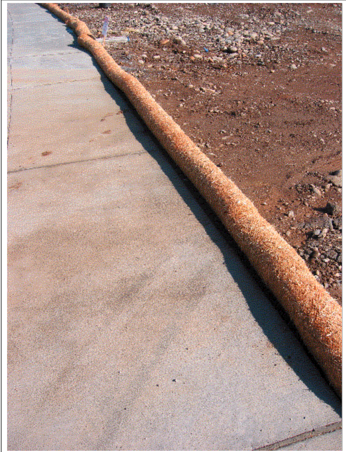
GRAND OAKS SUBDIVISION – CITY OF AUBURN EXAMPLE OF STRAW WATTLING FOR SEDIMENT AND EROSION CONTROL
