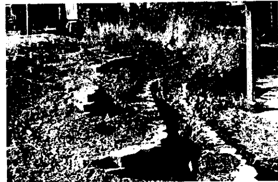
Extremely steep, eroding slopes like the one above need to be stabilized by incorporating structural means such as retaining walls or sturdy terraces. 12
