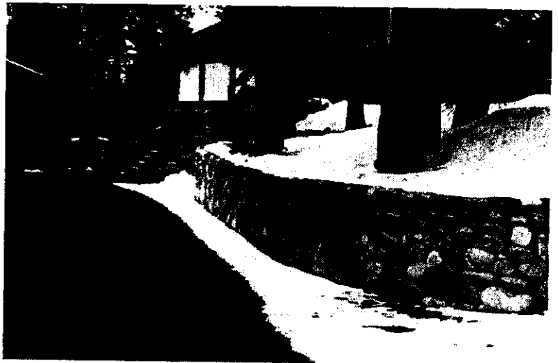
Above, a rock-faced retaining wall adjacent to a driveway.
