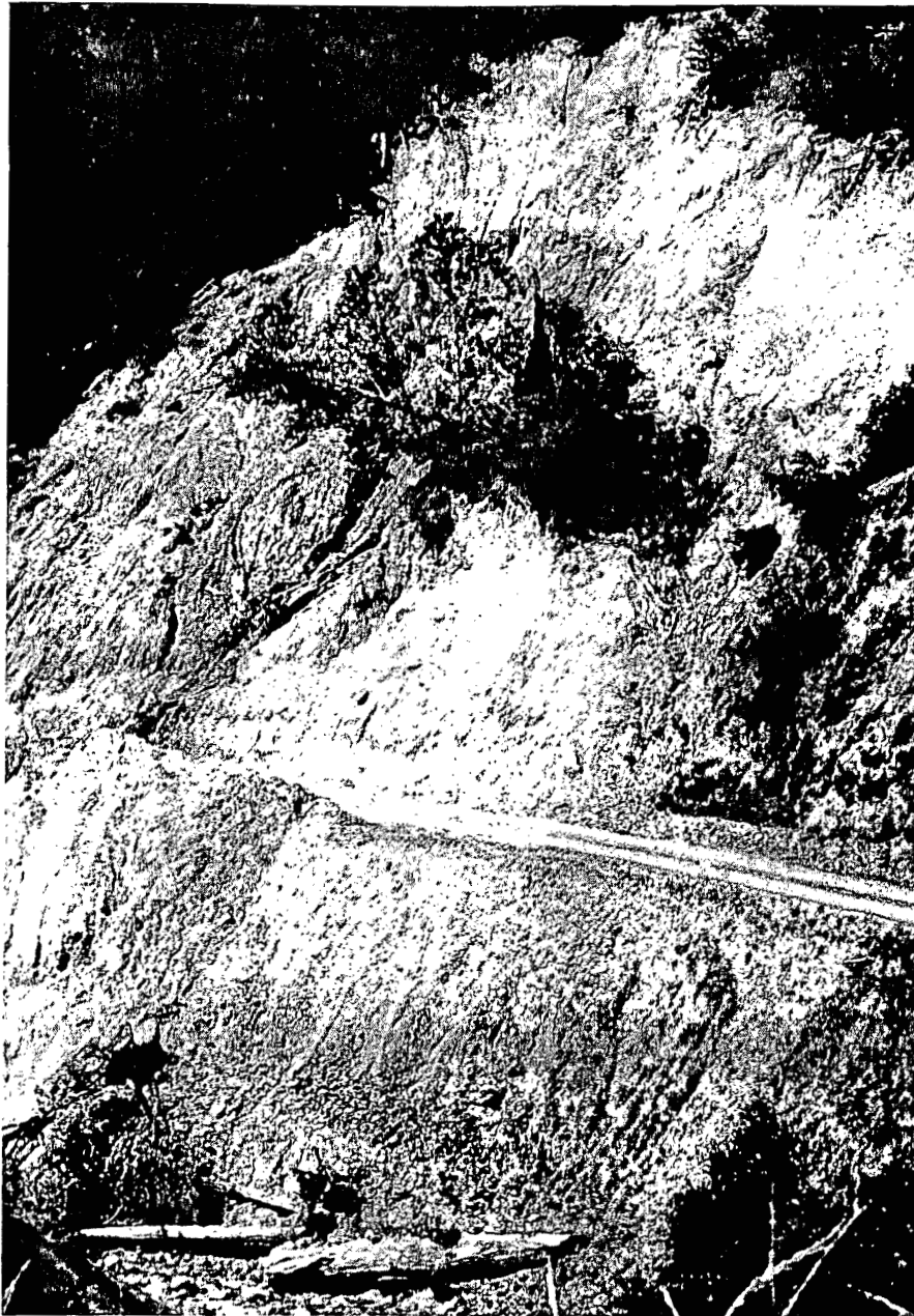
Fig. 4. Landslides and slope failures along roads and streams are major sources of erosion.
