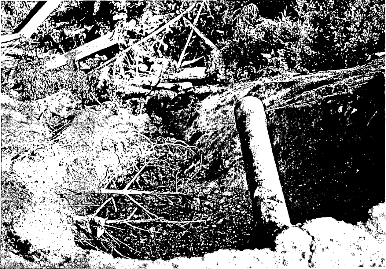
Fig. 2. Erosion caused by a culvert outlet with no energy dissipater.
