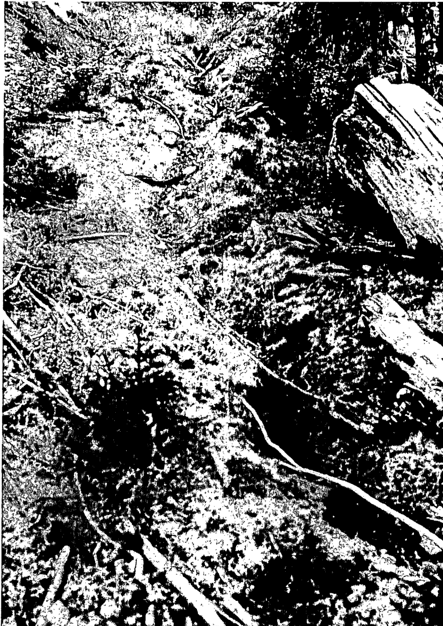
Fig. 7. The skidroads in the older logging areas generally had few, if any, waterbreaks. However, most of the skid roads have stabilized or have been revegetated with grasses and forbs.
