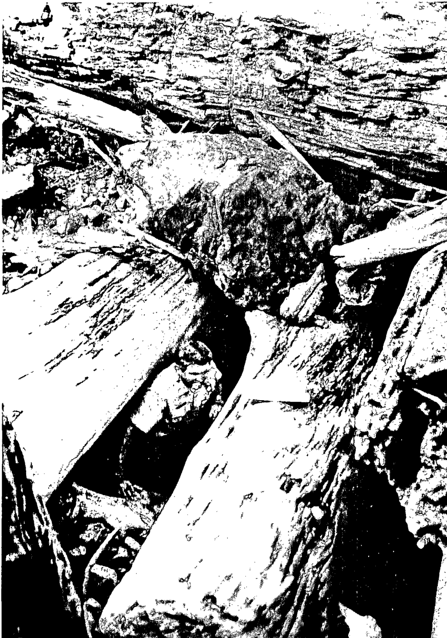
Fig. 3. An old log bridge which has collapsed and is causing stream blockages.
