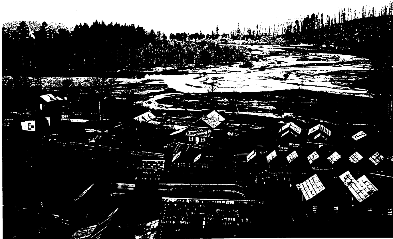
Figure 11 -- Riverside on Mad River near Blue Lake. View toward the west from Riverside before 1890 meander cutoff (taken between 1883 and 1890) at the confluence of the Mad River with the North Fork. Mad River flows from left to right. (Photo courtesy of Don Tuttle, Humboldt County Public Works Collection, Natural Resources Dept.).
