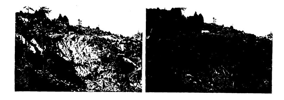
PHOTOS 2 and 3. (September and December, 1978): Log landing in the Miller Creek drainage on the C-line before and after rehabilitation by heavy equipment and manual labor crews. The outer part of the landing failed about 5 years ago and left a perched scarp of soil and organic debris above the stream. Heavy equipment removed the perched material, recontoured the slope, and manual labor crews then planted and wattled the slope (see text).
