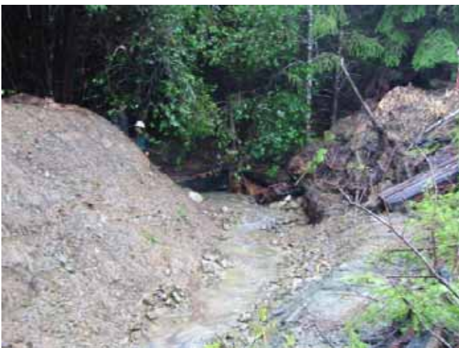
Figure 37. Legacy watercourse crossing removal.
