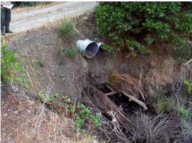
Figure 36. Watercourse crossing at high risk of failing.
