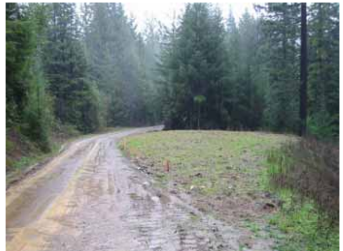
Figure 38. Reclaimed landing on mainline road.
