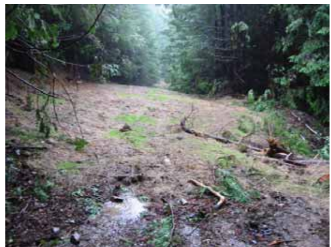
Figure 39. Abandoned road re-contoured to natural slope.
