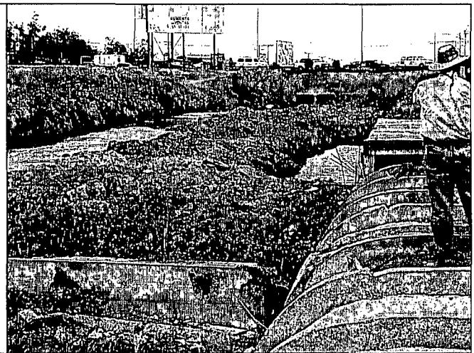
PHOTO NO. 32-NEW RIVER ENCASEMENT
