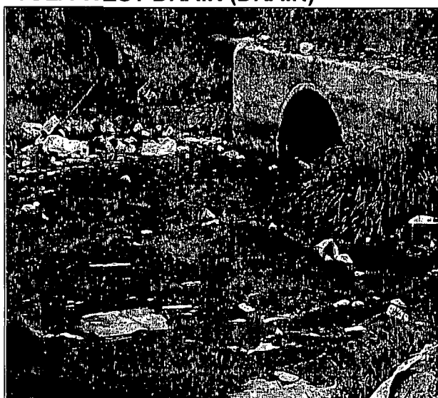
PHOTO NO. 1-TULA DRAIN
