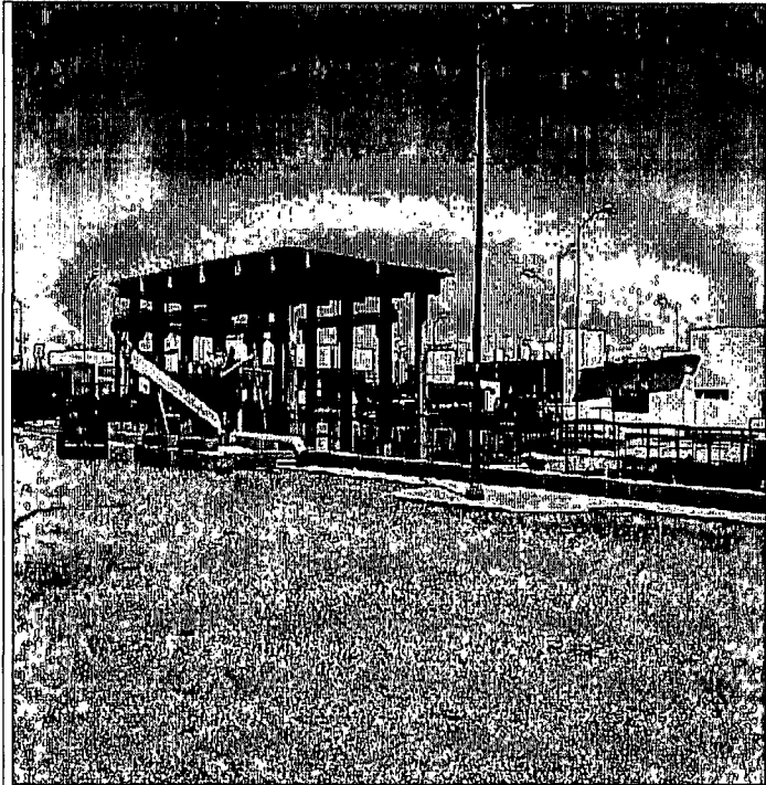
Photo No. 11 – Pump Station No. 4 Pump station No. 4 has been completed.
