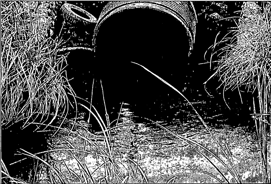
PHOTO NO. 28 - PRINCIPAL COLLECTOR
