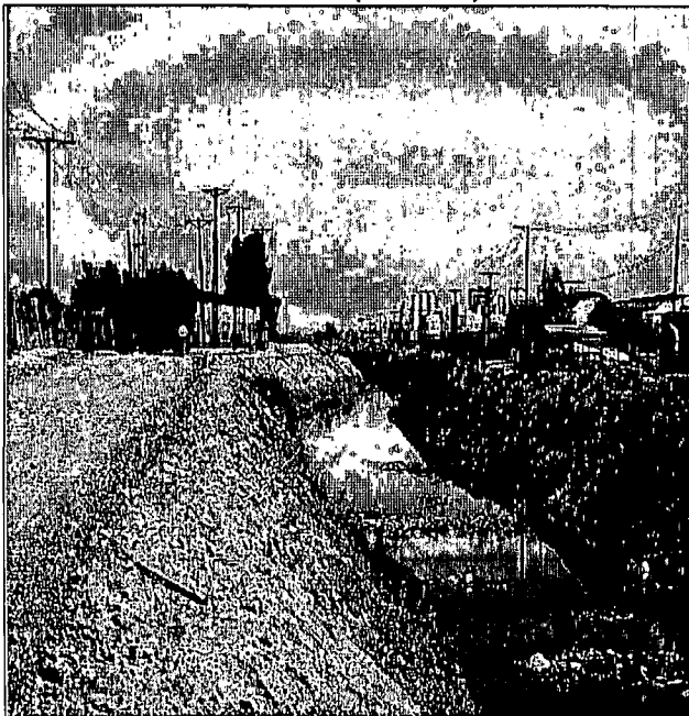
Photo No. 1 - Tula Drain
