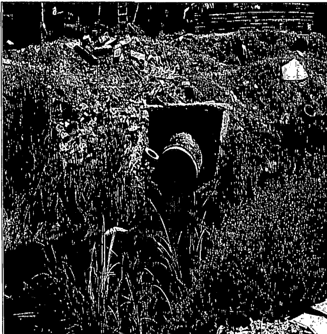
Photo No. 25- Principal Collector
