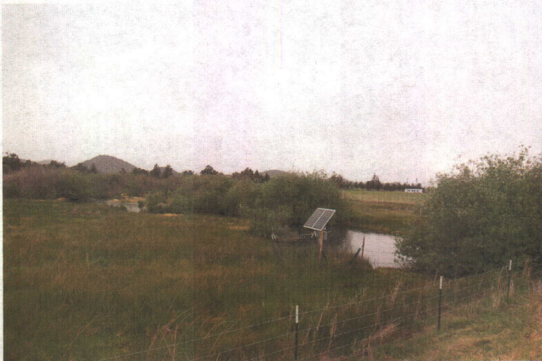
Photo 2: Diversion #241 Looking immediately downstream into Big Springs Creek. Date Taken: 4/16/2012
