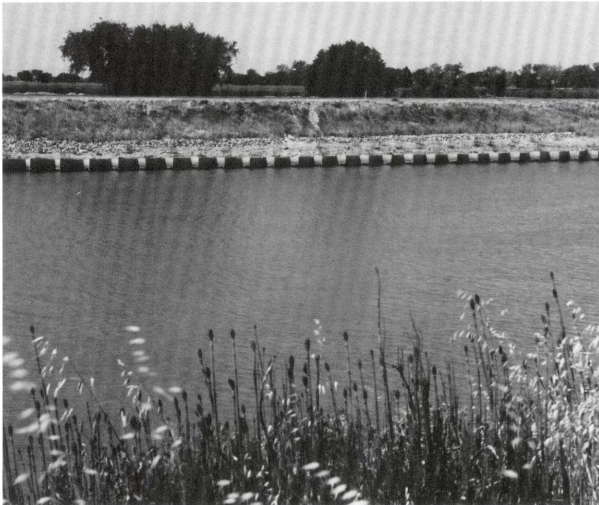
Experimental levee maintenance programs are being conducted at various locations in the Delta to determine better ways to protect the environment while maintaining proper safety for flood control. This photo shows a project to develop a berm that will provide for environmentally important shaded aquatic habitat.
