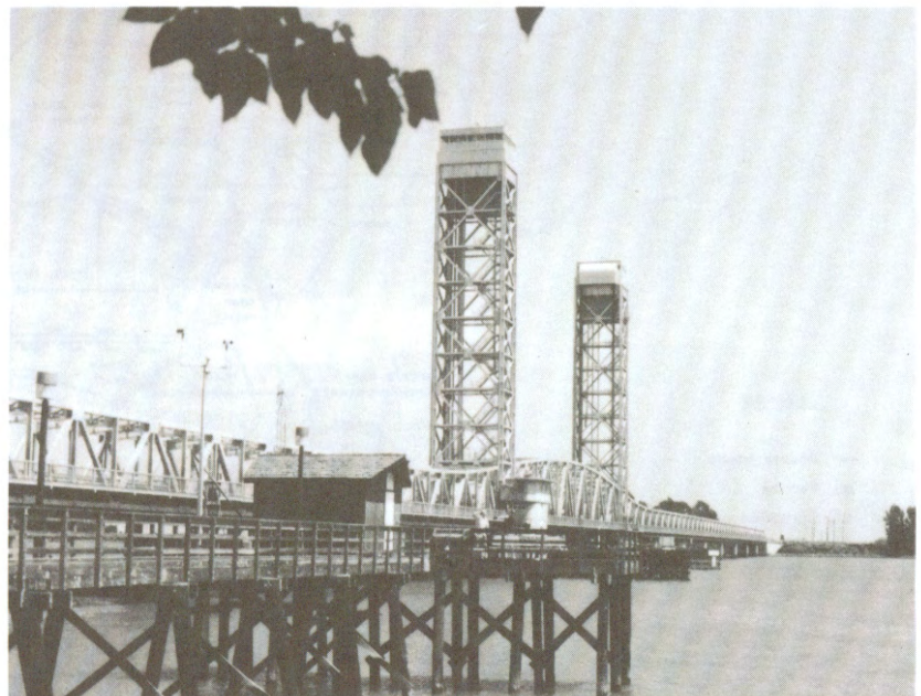
Rio Vista bridge on State Highway 12.
