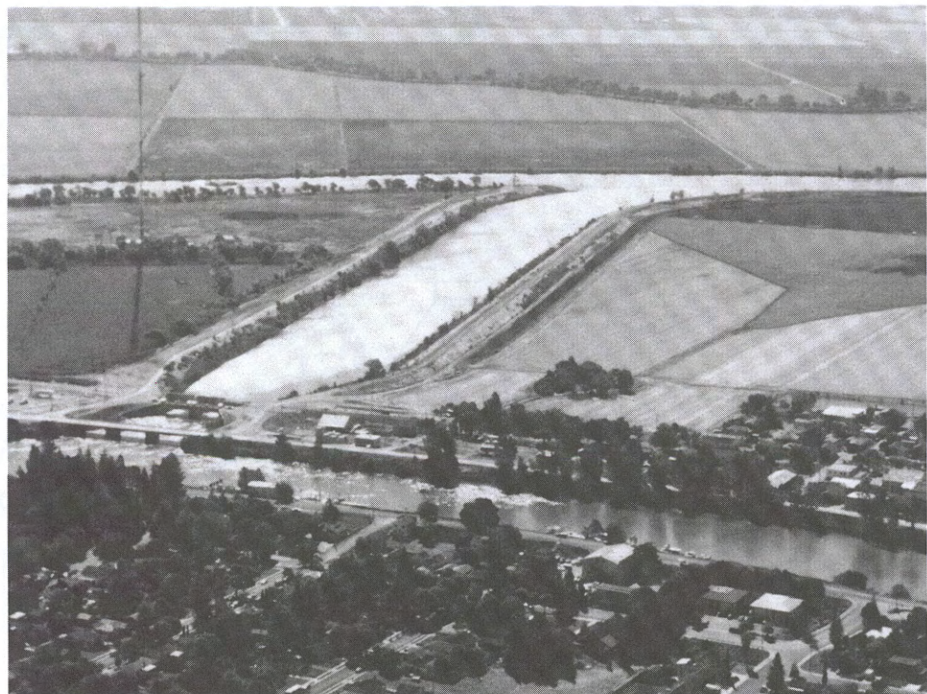
The Delta Cross Channel, constructed by the Bureau of Reclamation in 1951, connects the Sacramento River (foreground) with Snodgrass Slough and the Mokelumne River system.
