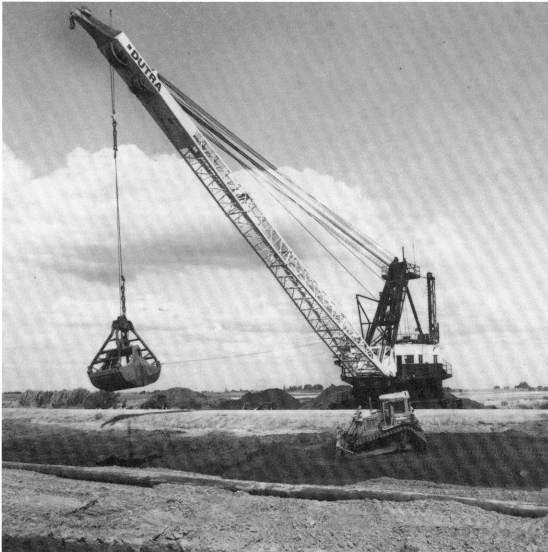
Levee rehabilitation on Twitchell Island.
