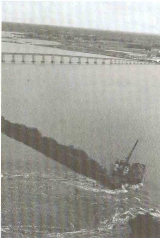
Levee break on Sherman Island in 1969.
