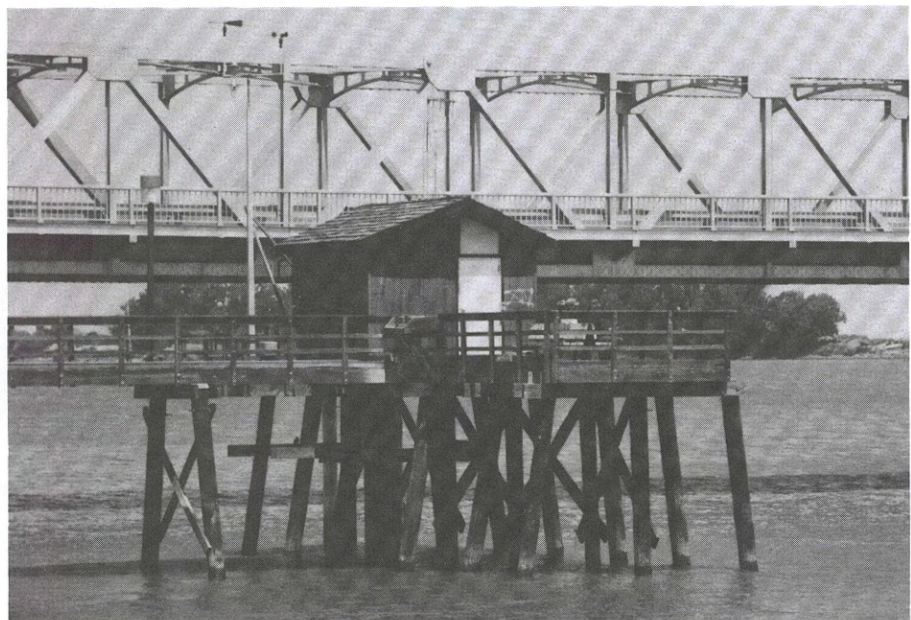
Fixed monitoring station at Rio Vista continuously monitors water level, salinity, temperature, dissolved oxygen, turbidity, and pH. It also measures wind speed and duration and solar radiation. It is one of over 35 stations in the Delta.
