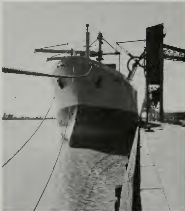
Deep-water channels through the Delta allow cargo to move on a large scale to and from the Ports of Stockton and Sacramento. The Port of Sacramento shipped a record tonnage exceeding 1.8 megatonnes (2 million tons) in the 1977-78 fiscal year.
