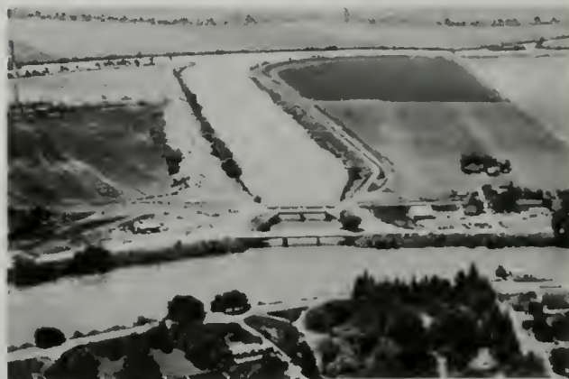
The Delta Cross Channel - the diversion upstream from Walnut Grove that routes Sacramento River water to the central Delta via the Mokelumne River.
