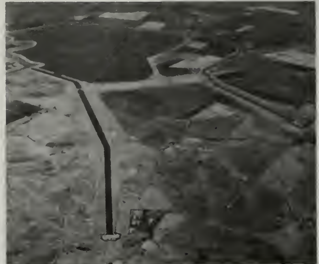
Clifton Court Forebay serves as the main Delta diversion point for the SWP. The Tracy Pumping Plant pumps water directly from Old River into the CVP Delta-Mendota Canal.
