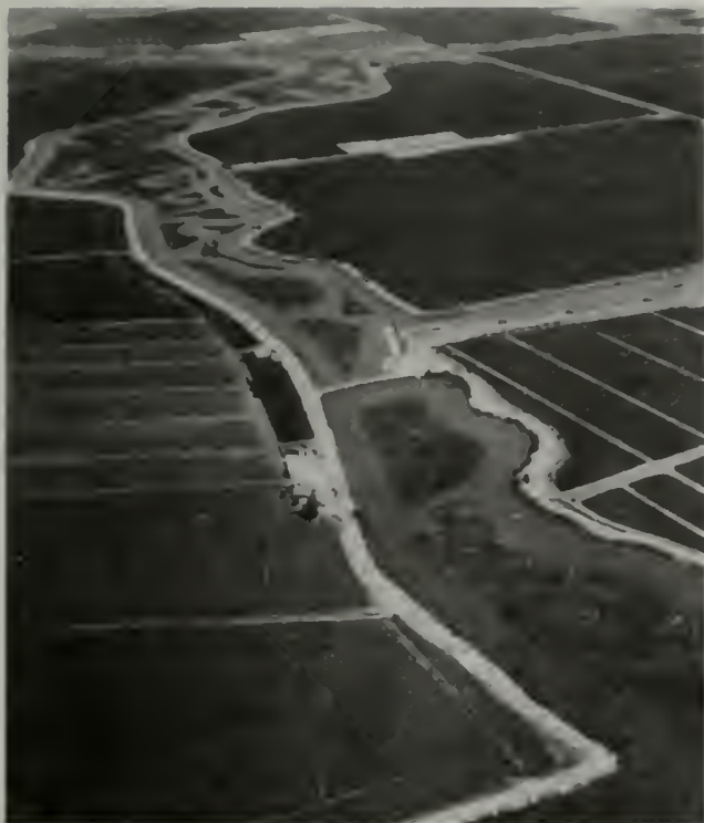
Disappointment Slough looking west near where the Peripheral Canal will cross. The first stage of the canal, which will be siphoned under the slough, will terminate just south of here. Water from the Peripheral Canal will be released into Disappointment Slough and other sloughs along the canal route to improve the water quality.
