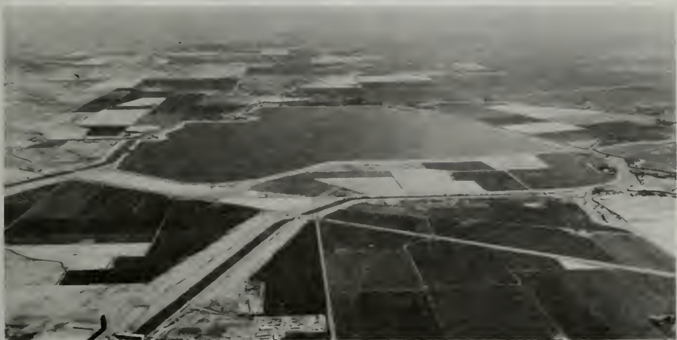
Clifton Court Forebay (center), which presently serves as the main diversion point for the SWP, will be terminus ad quem of the Peripheral Canal. As such, water regulated here will serve both the SWP Delta Pumping Plant (intake to the California Aqueduct, center left), and the CVP Tracy Pumping Plant, left foreground.
