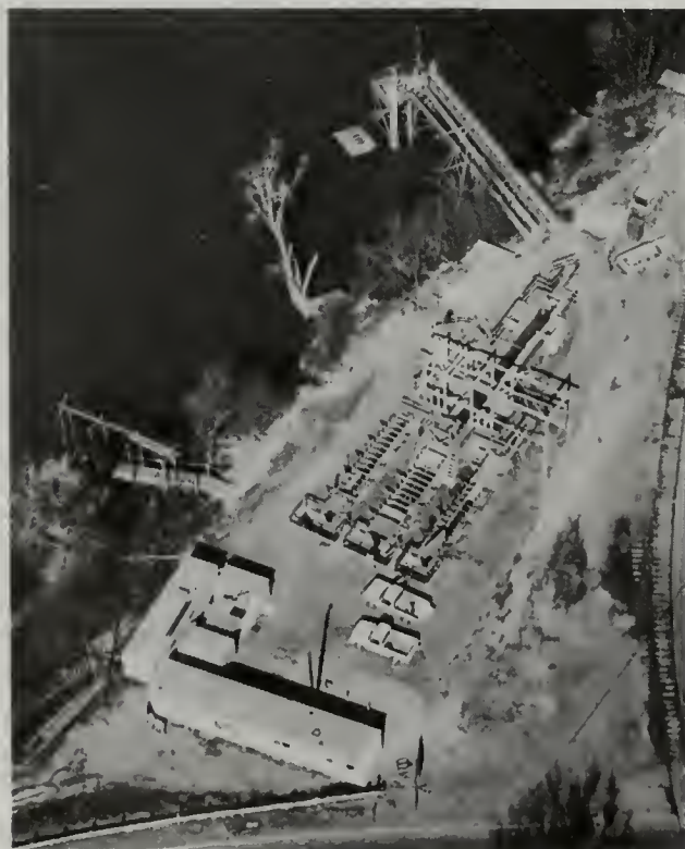
Fish screen test facility at town of Hood on Sacramento River. Biological and engineering tests are being conducted at this research and development facility to select the type of intake and fish screening system for the Peripheral Canal.
