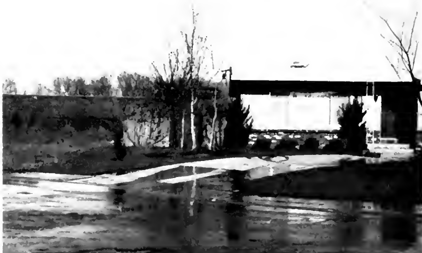
Figure 14. Seepage conditions along the Sacramento River near Chicory Bend in the South Sacramento area.
