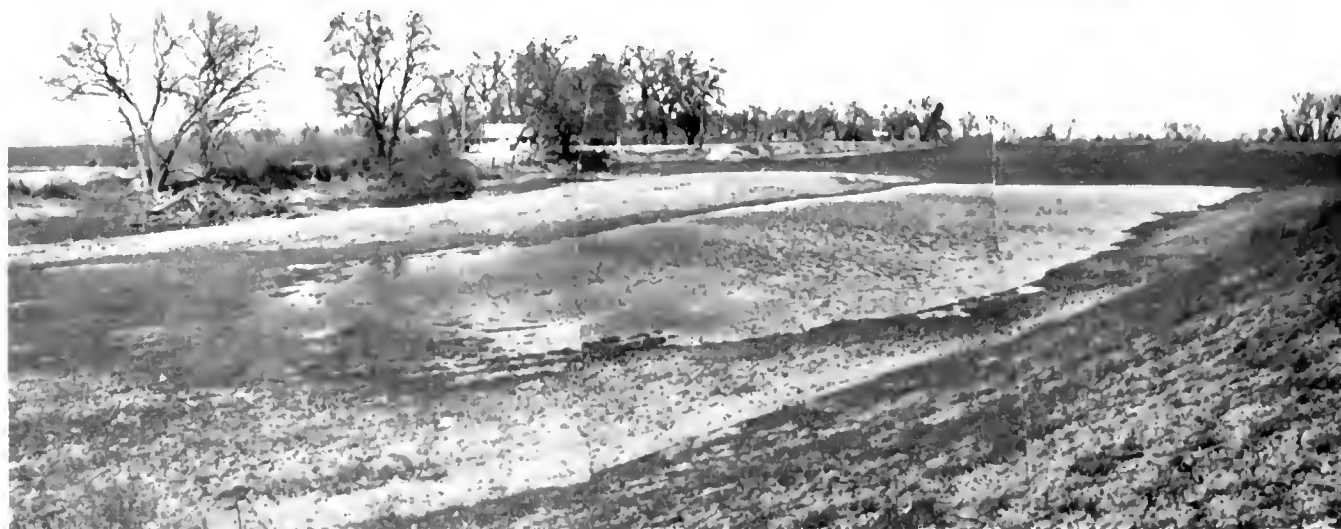
Figure 6. Ponded seepage between river levee and natural levee.
