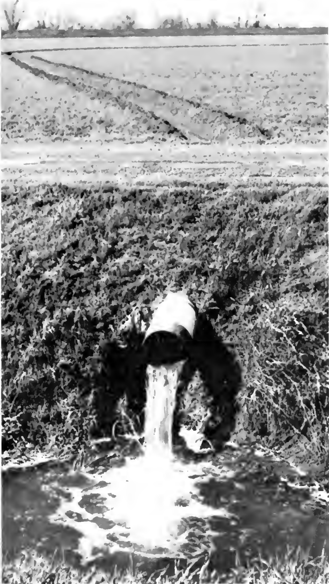
A 12-inch outfall pipe spilling seepage collected from field drain adjacent to the Sacramento River on the Van Ruiten ranch upstream from Kirkville. The flow at the outfall was estimated to be 0.25 cfs.
