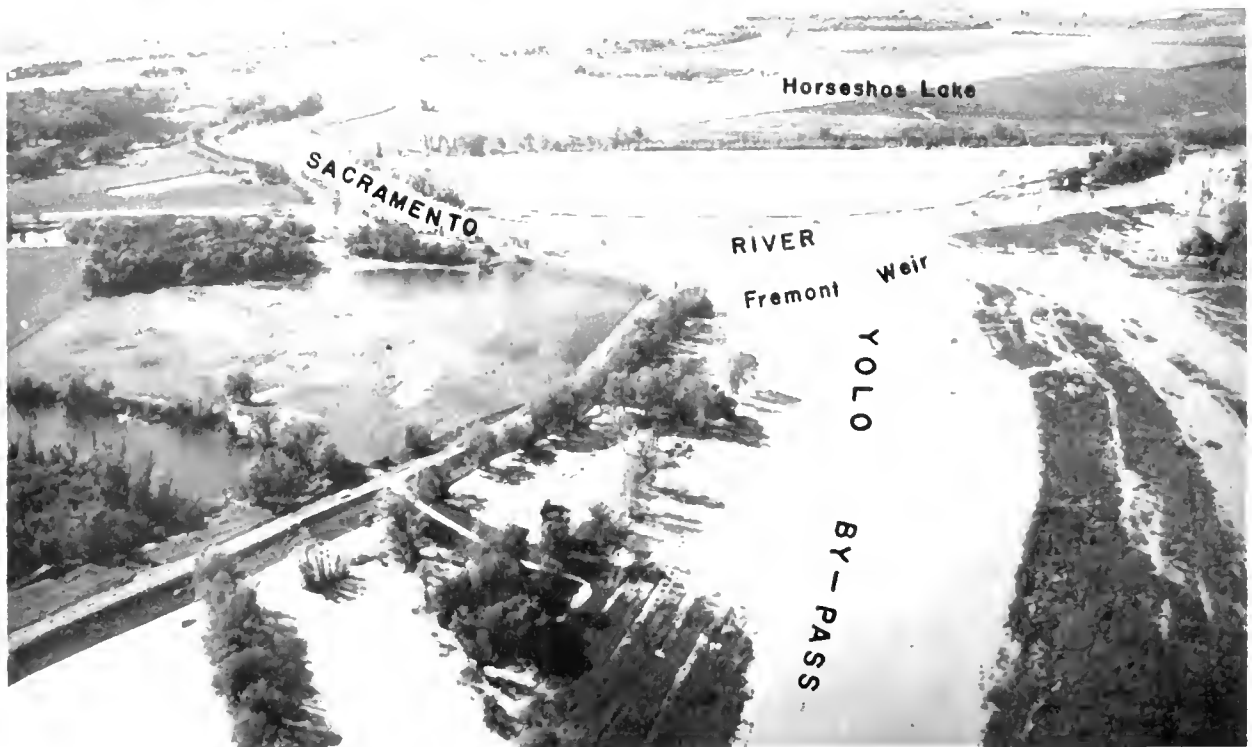
Figure 5. Tisdale and Fremont Weirs overflowing during the April 1963 seepage period
