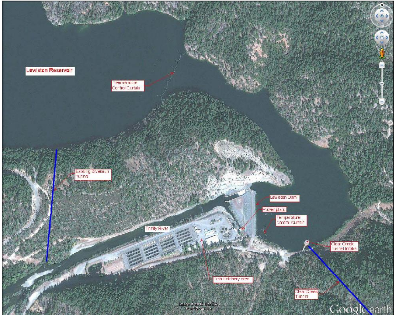
Figure 1. Lewiston Dam and Reservoir Facility and Structures.
