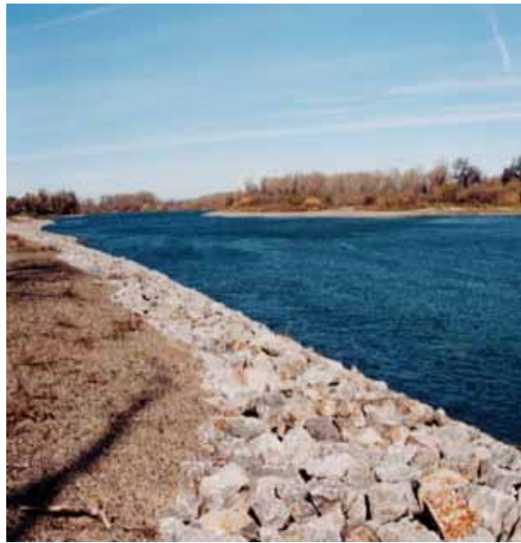
Typical Rock Revetment Along Sacramento River
