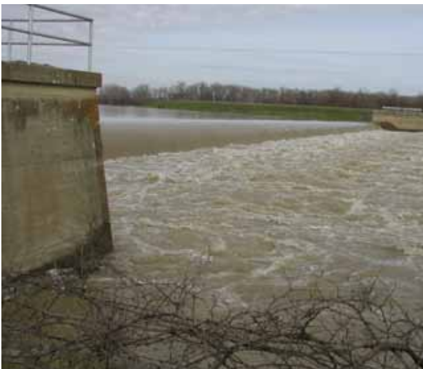
Floodflow over the Moulton Weir
