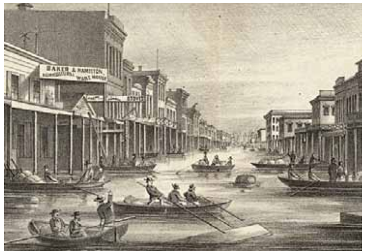
1862 Flooding in Sacramento
