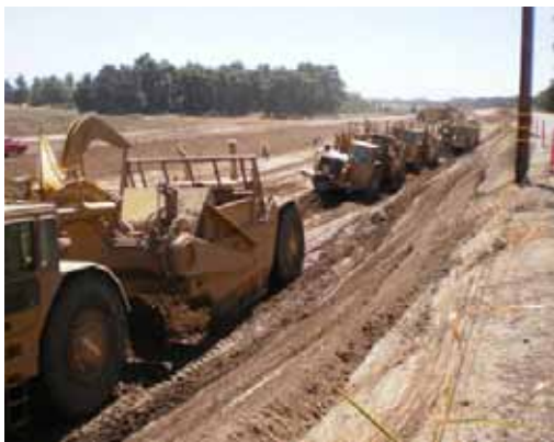
Levee Improvements in Natomas
