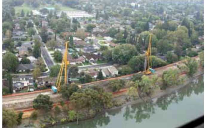
Geotechnical improvements to levees in the Pocket Area of Sacramento
