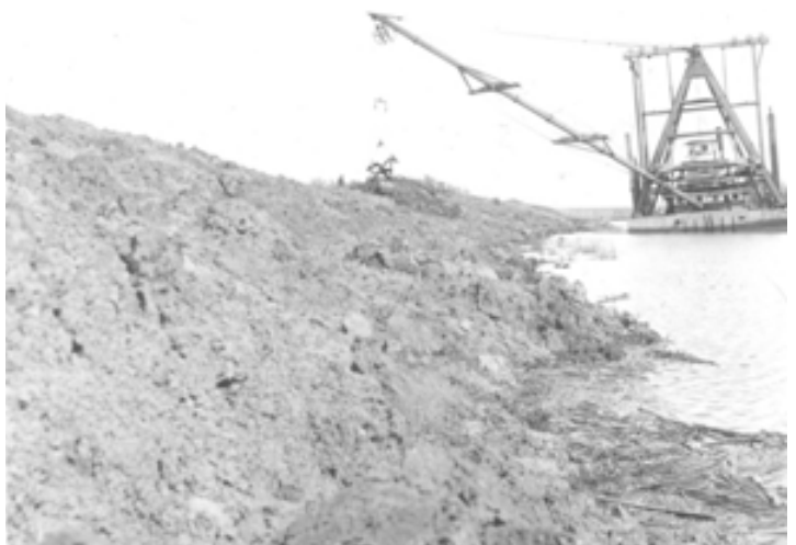
Construction of Yolo Bypass Levee
