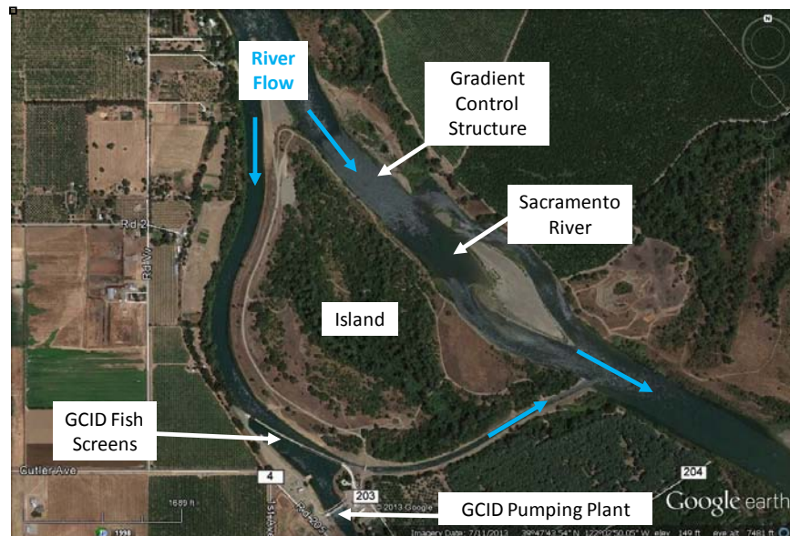
Figure 20. The GCID Hamilton City Pumping Plant and associated features of the Fish Screen Improvement Project.
