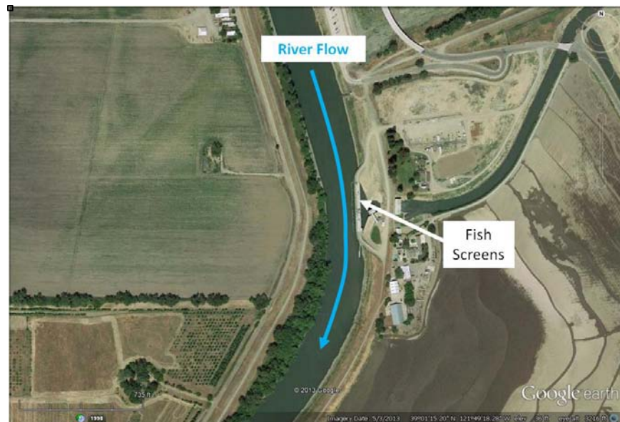
Figure 4. Aerial photograph of an example of an existing Sacramento River flat-plate fish screen located on an outside river bend to maintain high sweeping velocities.
