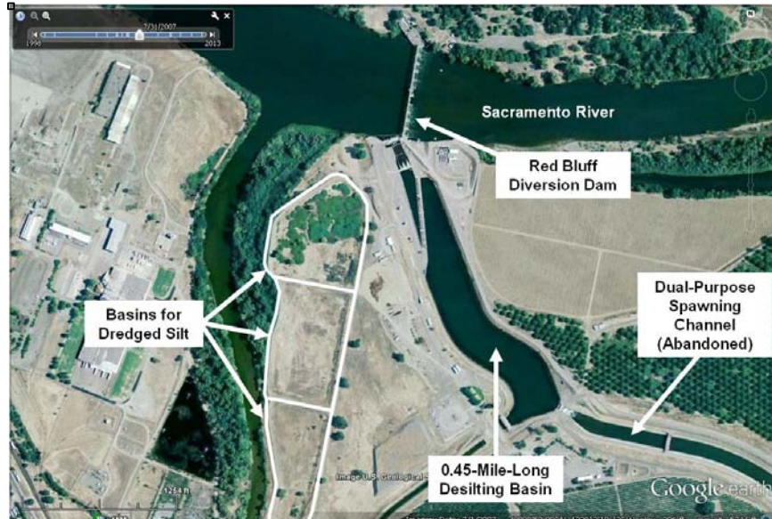
Figure 18. Aerial photograph of the Tehama-Colusa Canal headworks showing the 0.45-mile long desilting basin.
