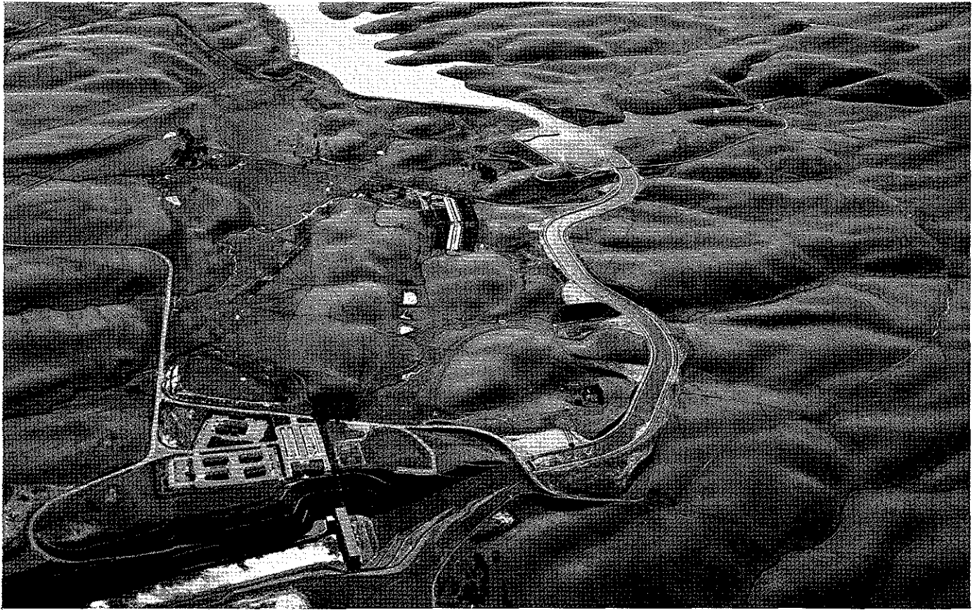
Department of Water Resources' Delta Pumping Plant, showing the California aqueduct and Bethany Reservoir.
