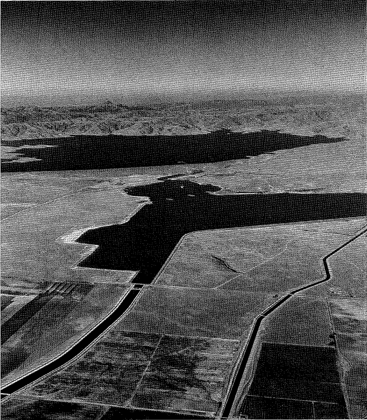
San Luis Dam and the O'Neill Forebay are part of both the Central Valley Project and the State Water Project. San Luis Reservoir stores water diverted from the Delta during the winter when irrigation demand is low. Water is then released later in the year to serve water contractors in the Central Valley and southern California. In addition to the reservoir, a portion of the California Aqueduct known as the San Luis Canal is jointly operated to serve both the Central Valley Project's San Luis service area and the State Water Project customers further south. (DWR photo)
