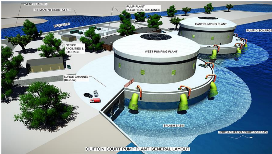
FIGURE 5: PROPOSED PUMPING FACILITIES AT CLIFTON COURT FOREBAY
