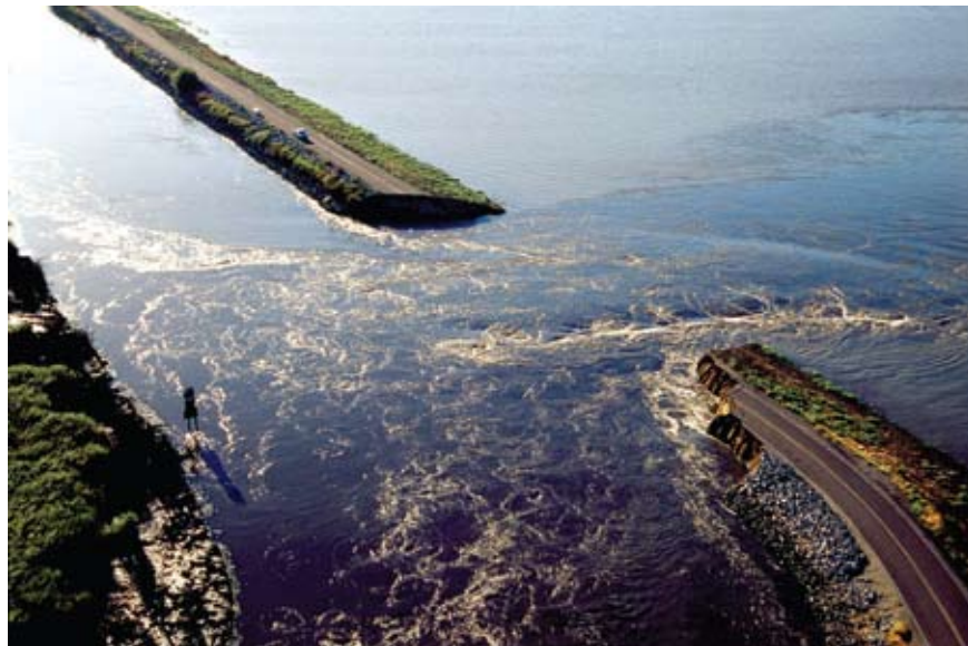
Figure 1.6. The Jones Tract levee failure and flooding of June 3, 2004. The levee was repaired and the Jones Tract restored at an estimated cost of $90 million. (Photo by: California Department of Water Resources)
