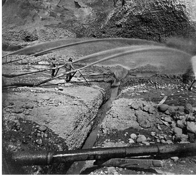
Figure 1.3. Hydraulic mining with high-pressure water hoses in the foothills of the Sierra Nevada. This method of placer mining was invented in California. (Photo by: California Department of Water Resources)
