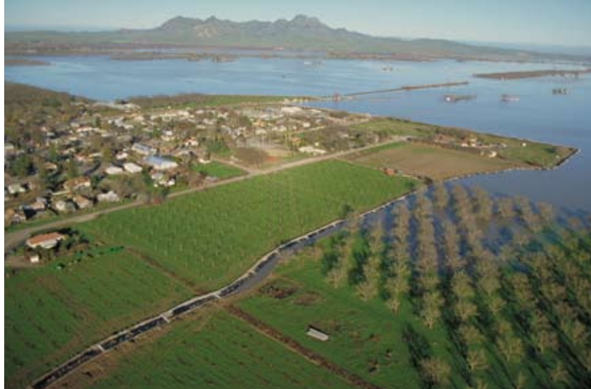
Figure I.2. Levee failures can result in extensive damage to homes and agricultural fields. Flooding also imperils our water supply. (Photo by: California Department of Water Resources)
