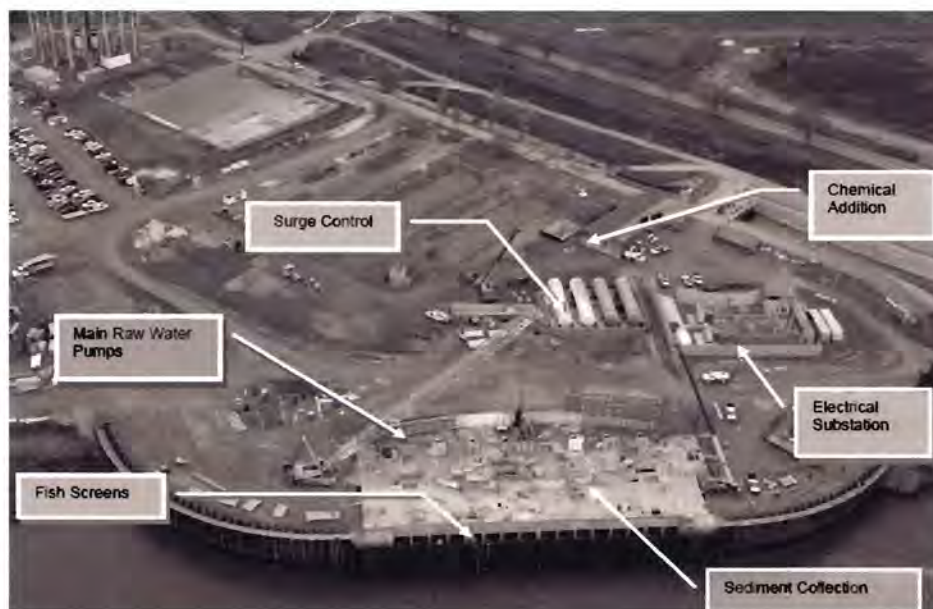
Figure 5 - Major Intake Systems Locations Shown on an Aerial Construction Photograph of Intake Site
