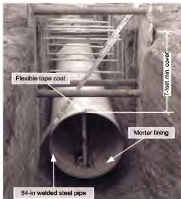
Figure 7 - Typical Trench Section
