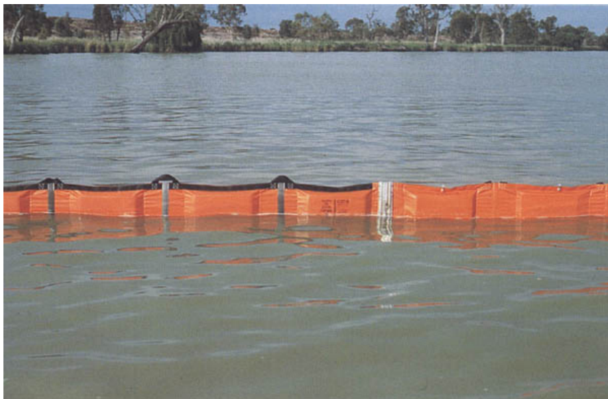
Figure 2.2G Use of a barrier or boom to keep surface scums of algae and cyanobacteria away from water offtake structures (Photograph courtesy of Peter Baker, Australian Water Quality Centre)
