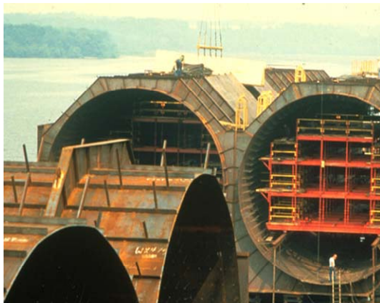
Figure 11-6 Fort McHenry Tunnel, Baltimore
