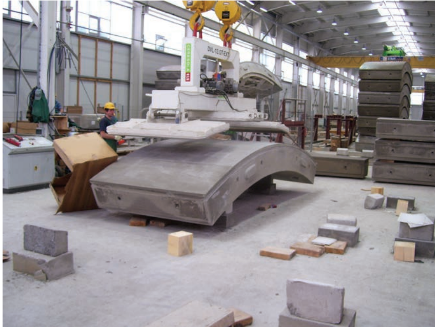
Figure 10-7 Precast Segments for One-Pass Lining, Forms Stripped
