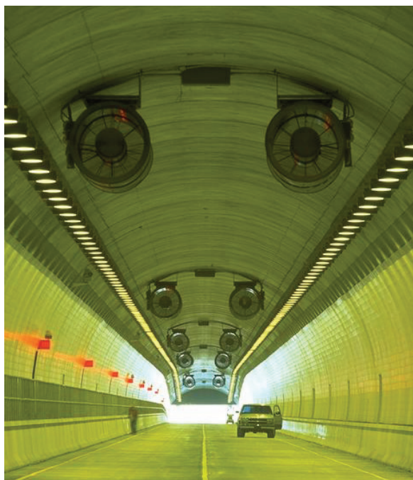
Figure 10-1 Cumberland Gap Tunnel
