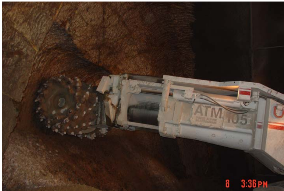
Figure 9-12 Road Header SEM Excavation in Medium Hard, Jointed Rock (Devil's Slide Tunnels, California)
