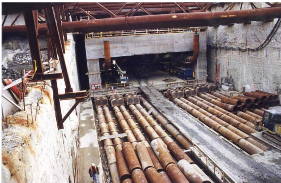
Figure 12-9 Progressive Installation of Packer Sections and Connecting Diaphragm Plates
