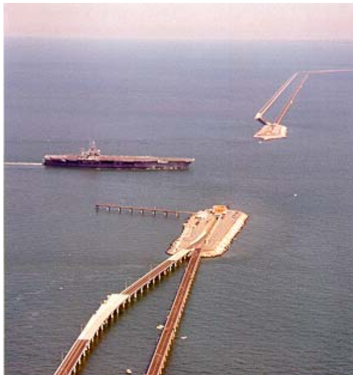
Figure 11-2 Chesapeake Bay Bridge-Tunnel
