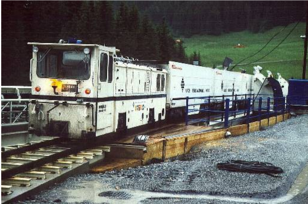
Figure 14-4 Muck Train Dumping at Portal
