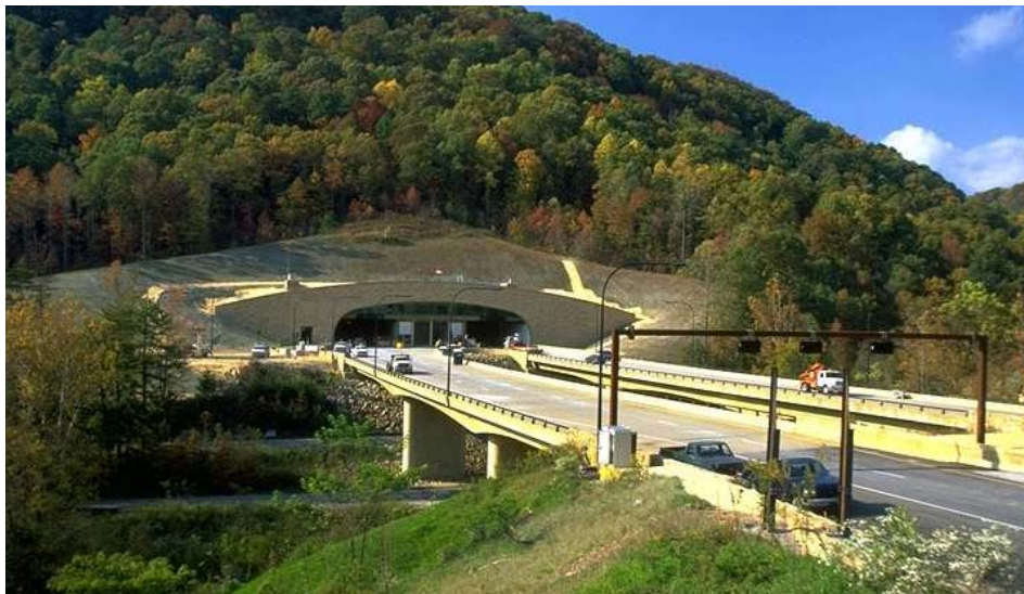
Figure 2-8 Portal Structure for Cumberland Gap Tunnel
