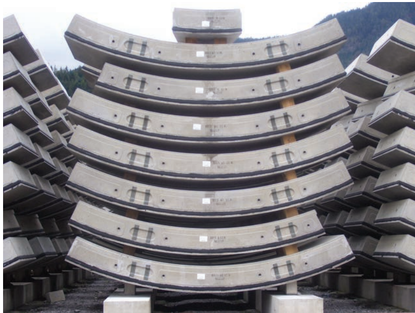
Figure 10-8 Stacked Precast Segments for One-Pass Lining
