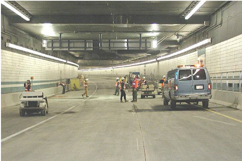
Figure 12-1 Completed I-90 Tunnels
