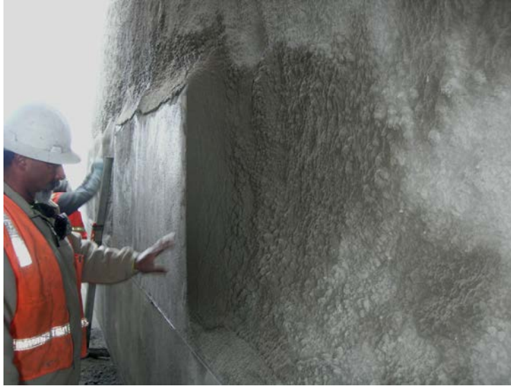
Figure 16-13 Shotcrete Finishing, Shawmut Jct. Boston
