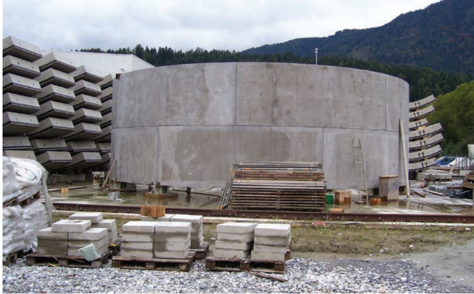
Figure 10-13 Mock-up of Precast Segment Rings
