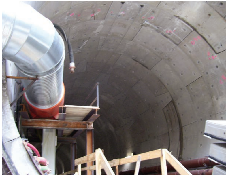
Figure 10-2 Precast Segmental Lining
