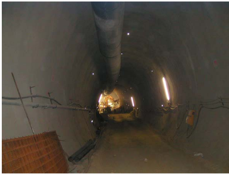
Figure 9-22 Deformation Monitoring Cross Section Points (Light Rail Bochum, Germany)
