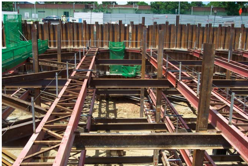
Figure 5-4 Sheet Pile Walls with Multi Level-Bracing
