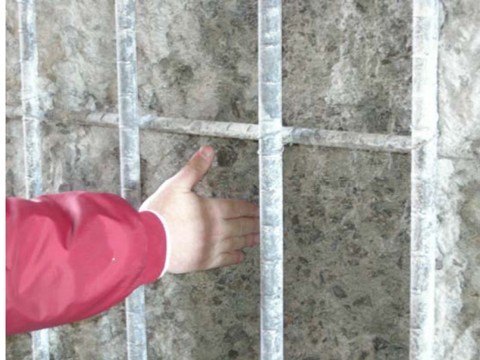
Figure 16-7 Substrate after Hydro-demolition, Shawmut Jct. Boston
