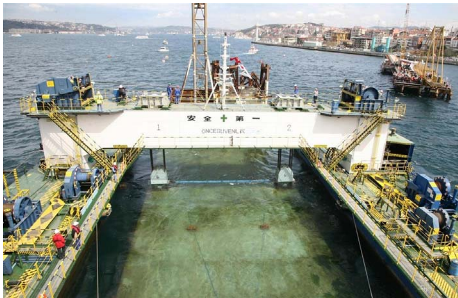
Figure 11-15 A Tunnel Element is Being Placed.
