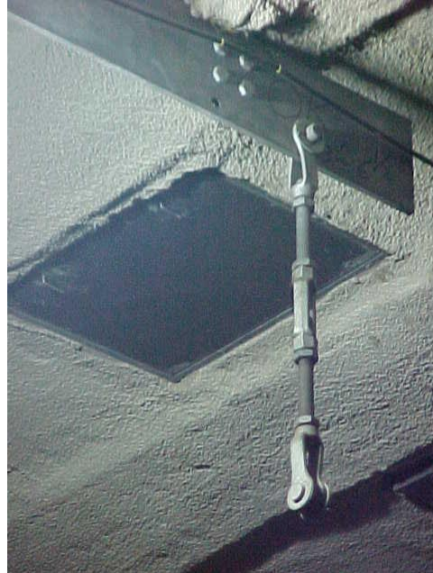
Figure 16-22 Typical Replacement Hanger Hardware
