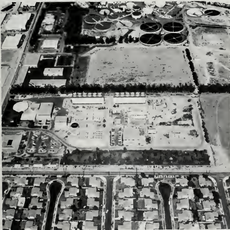
Water Factory 21 in Orange County. Operation of this plant, together with the primary and secondary treatment of municipal waste water at the plant appearing at top, involve most of the treatment processes in use today. Treated water produced by advanced treatment and desalted water are blended with water from deep wells and then injected underground to form a barrier to sea water intruding into the ground water in the region.
