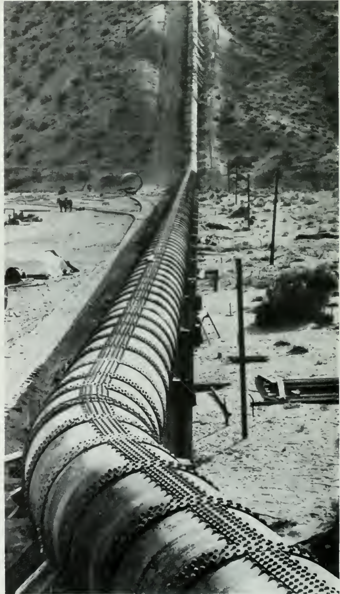
Water transported by the Los Angeles Aqueduct moves through an inverted siphon across Jawbone Canyon, about 100 miles from the terminus of the system.
