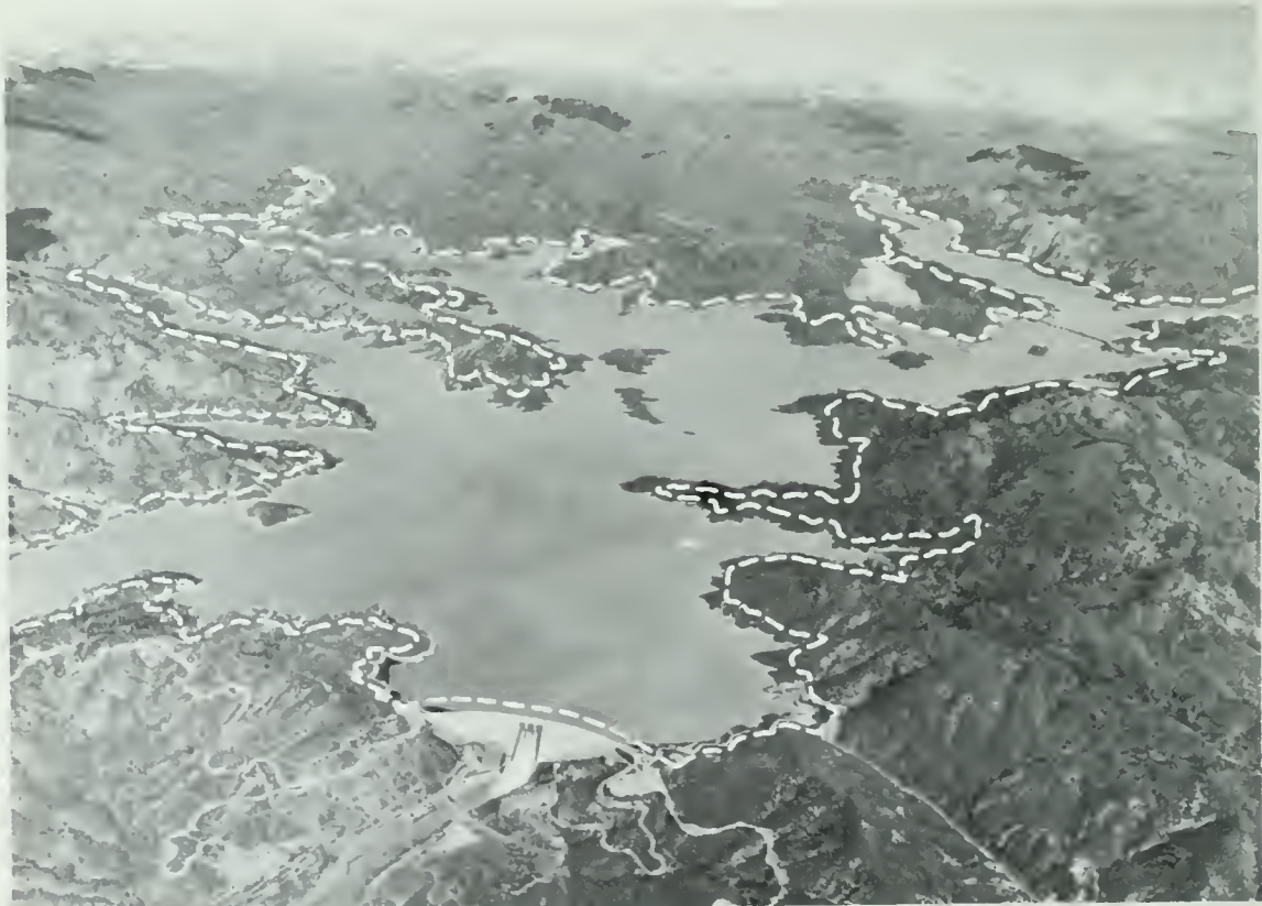
Shasta Dam and Reservoir of the Central Valley Project, showing the outline of the proposed enlargement. Raising the present height of the dam by another 200 feet would create a 14-million-acre-foot reservoir and increase the dependable water supply by about 1.4 million acre-feet per year.
