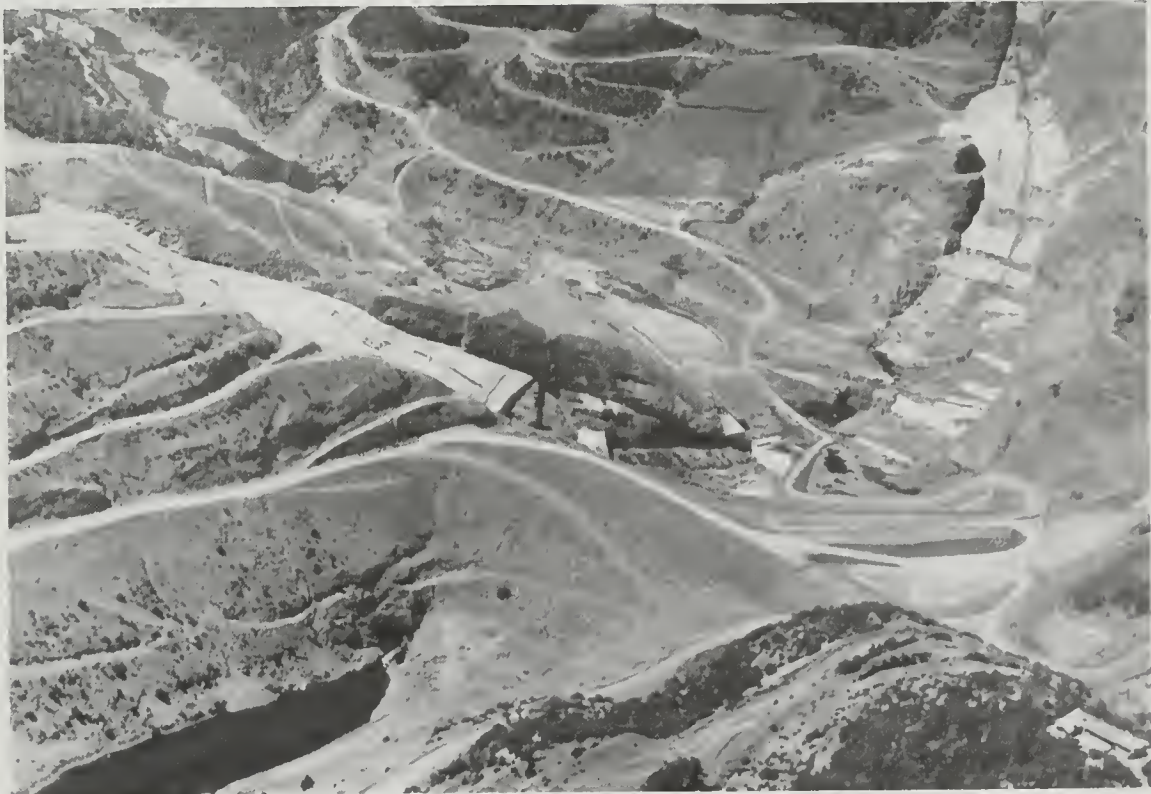
Auburn Dam site on the North Fork American River. Downstream view shows the present status of construction. A 200-foot-high upstream cofferdam is situated in the foreground, with the dam's keyway or "notch" in the canyon visible just above. Work on the dam has been suspended, pending redesign to meet higher seismic criteria and reauthorization by Congress.
