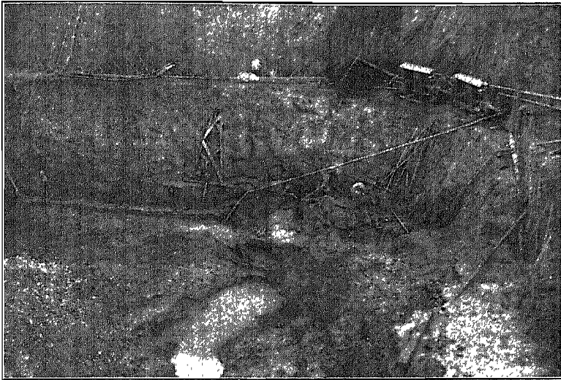
FIG. 145. Open excavation in soft silt at site of Bonneville Dam, Ore., after consolidation by the vacuum method.
