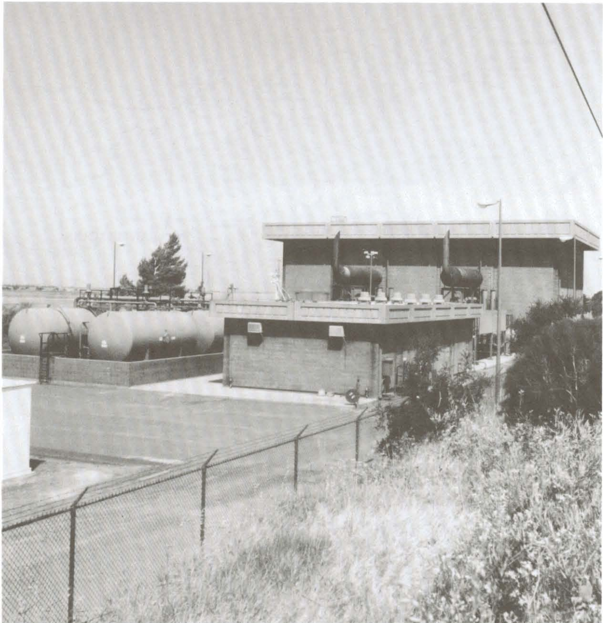
One of Pacific Gas and Electric Company's natural gas facilities on Brannan Island.
