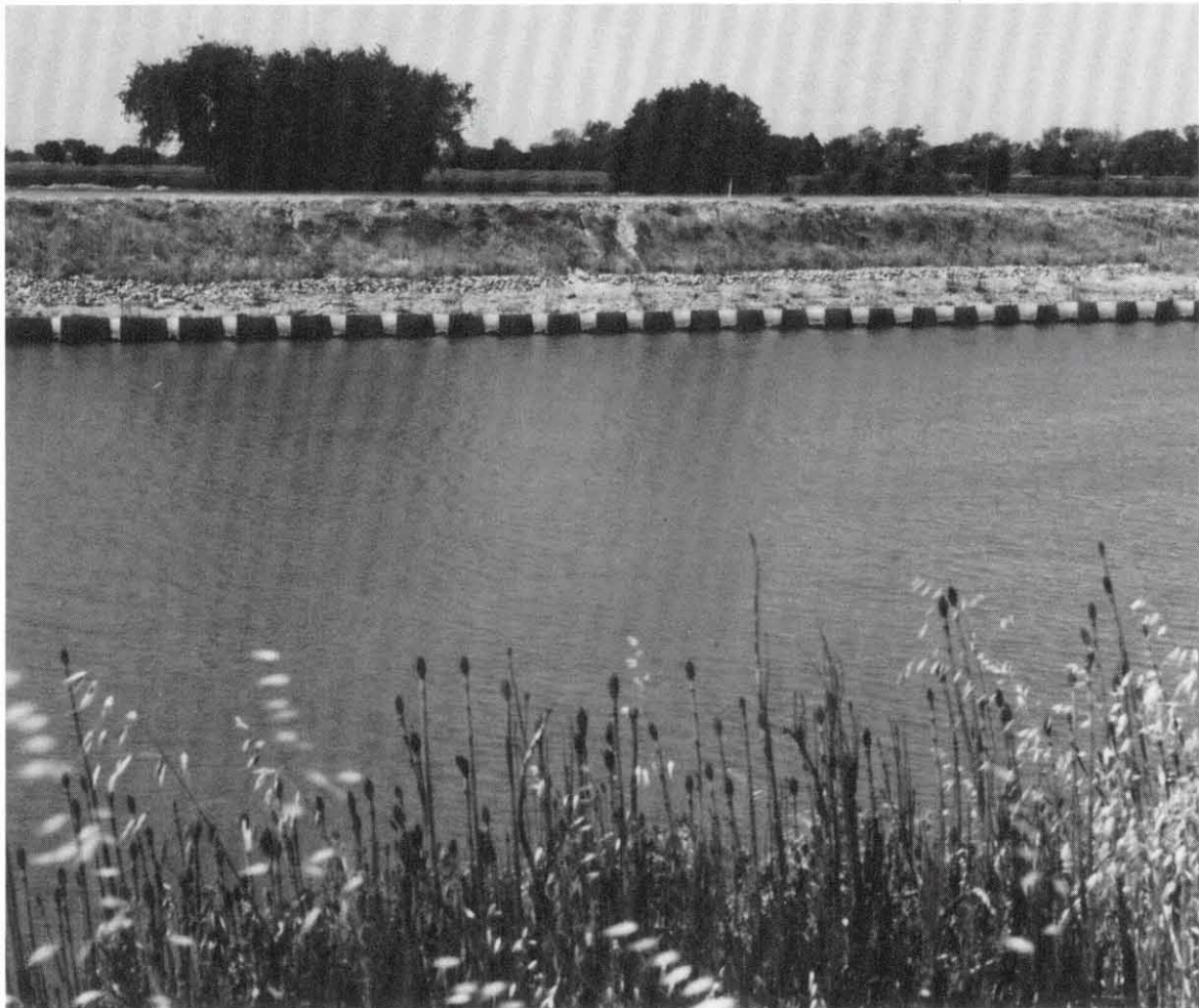
Experimental levee maintenance programs are being conducted at various locations in the Delta to determine better ways to protect the environment while maintaining proper safety for flood control. This photo shows a project to develop a berm that will provide for environmentally important shaded aquatic habitat.
