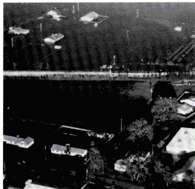
1986 flooding of the town of Thornton adjacent to the South Fork Mokelumne River.
