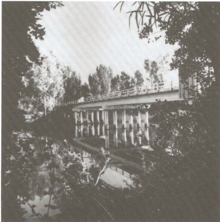
View of a bridge on a local road in the Delta.
