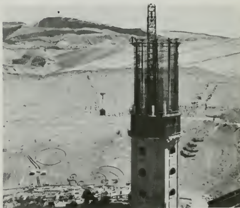
Figure 395. Concrete Placement—High Intake Tower
