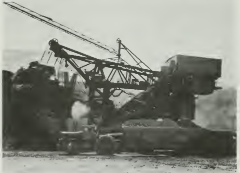
Figure 234. Wheel Excavator Cutting on 50-Foot-High Face
