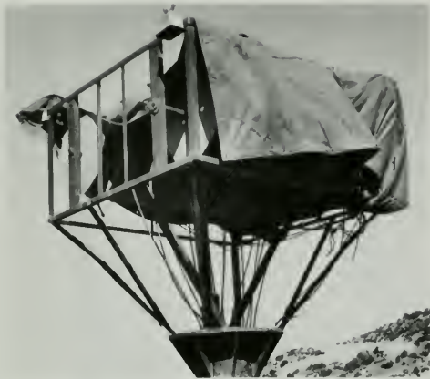
Figure 256. Instolltion of Piezometer Tubing
