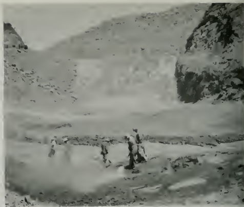
Figure 326. Air-Water Jet Cleanup of Foundation
