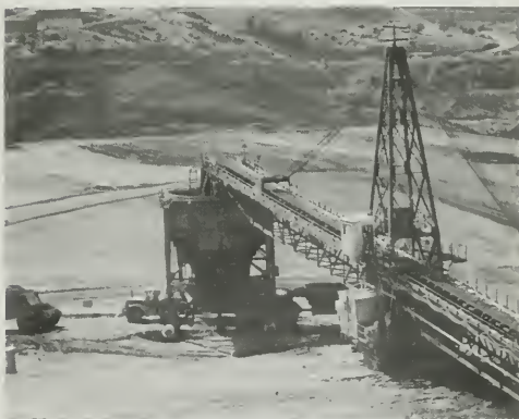
Figure 113. Truck-Loading Hopper
