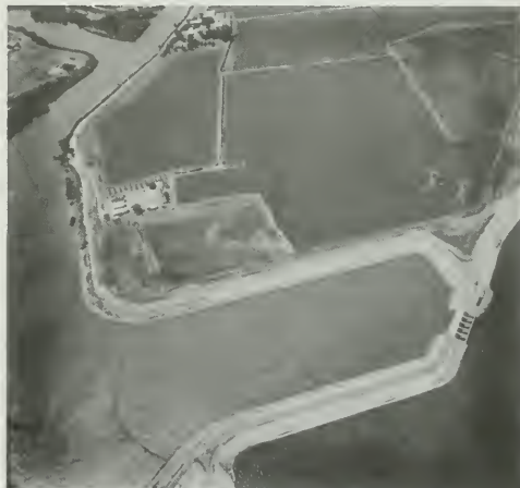
Figure 178. Control Structure and Inlet Channel Connection to West Canal and Old River (in background)
