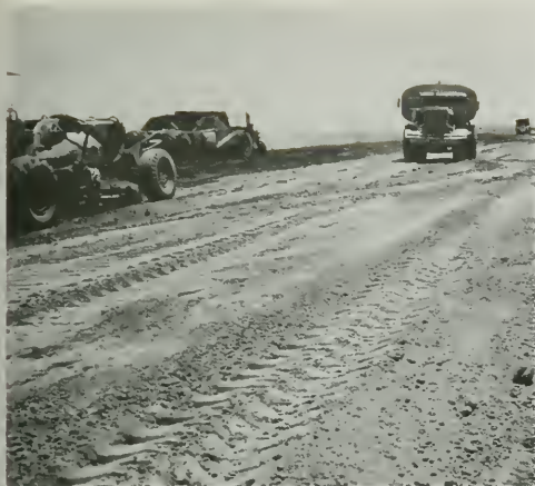
Figure 154. Afterbay Dam Construction
