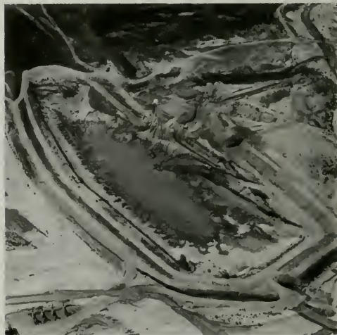
Figure 381. Foundation Exploration Trench
