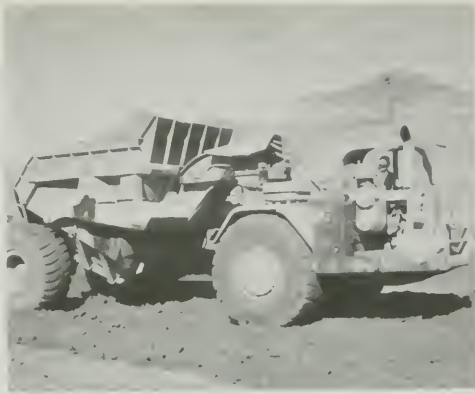
Figure 328. Rear-Dump Rock Wagon Used for Embankment Hauling
