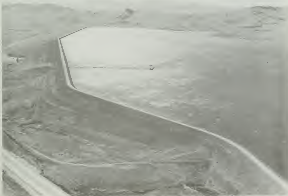
Figure 228. Aerial View—San Luis Dam and Reservoir
