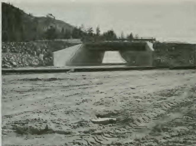
Figure 54. Spillway Approach and Log Boom
