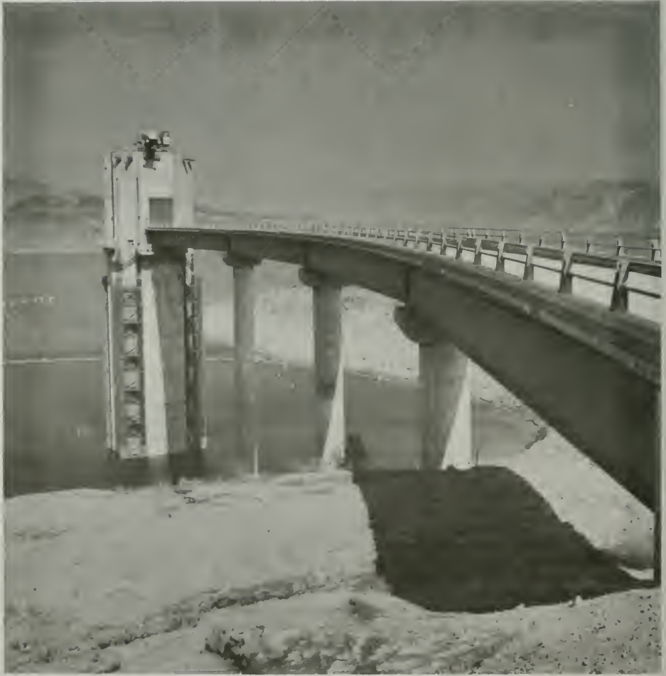
Figure 354. High Intake Tower and Access Bridge
