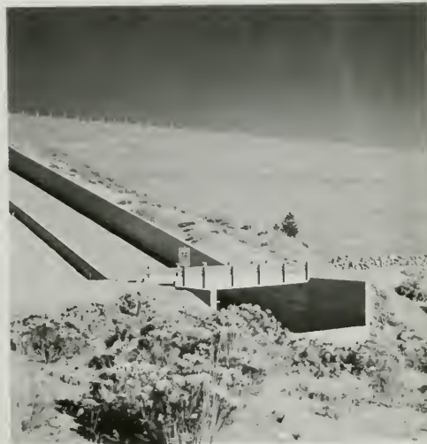
Figure 25. Spillway Flip Bucket
