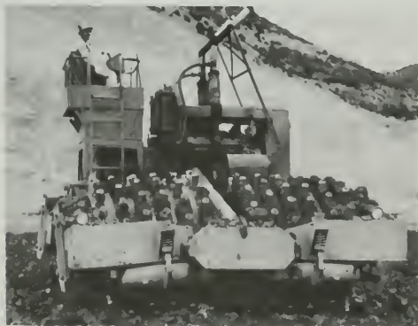
Figure 272. Compacting Zone 1 Material
