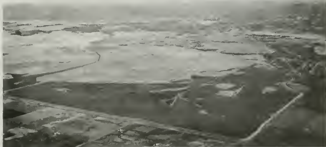
Figure 132. Aerial View—Thermalito Afterbay
