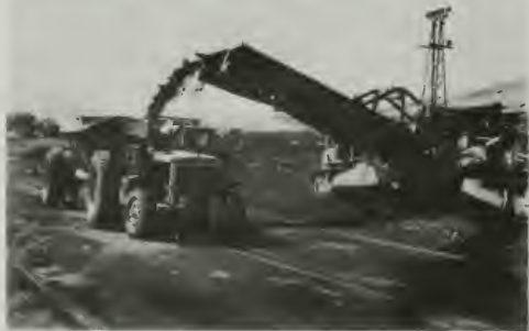
Figure 291. Excavation in Clay Borrow Area
