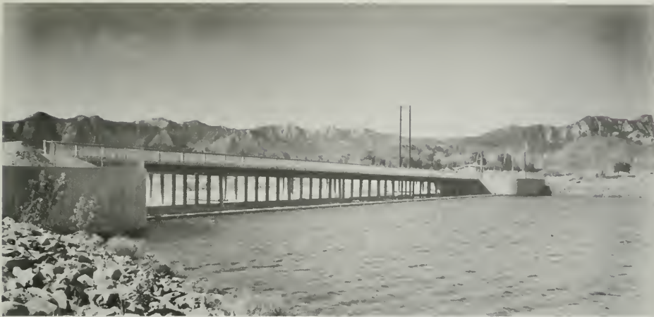
Figure 362. Castaic Lagoon Control Structure
