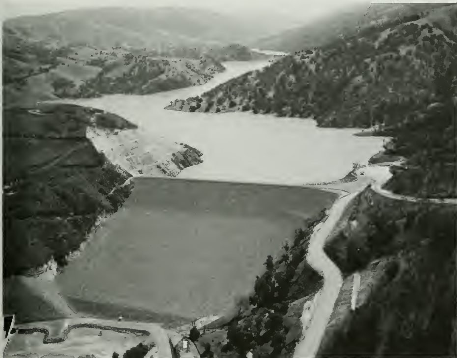
Figure 203. Aerial View—Del Valle Dam and Lake Del Valle
