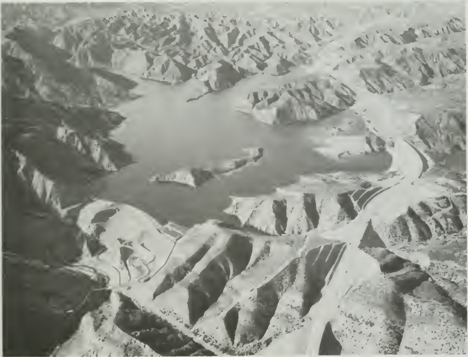
Figure 301. Aerial View—Pyramid Dam and Lake
