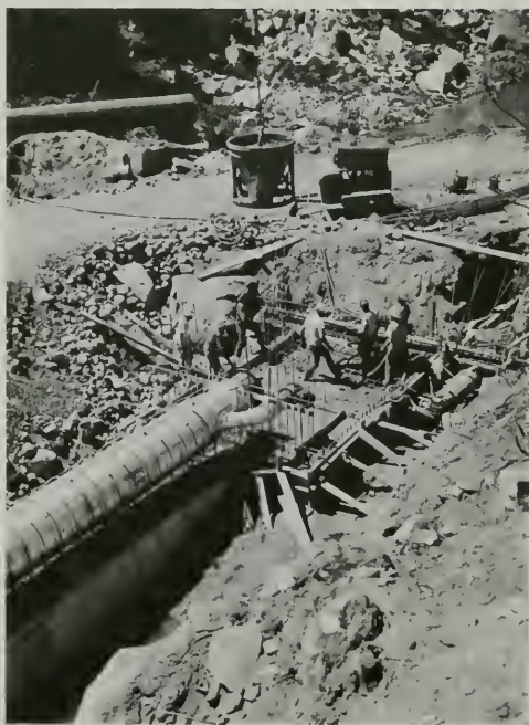
Figure 37. Outlet Works Control Structure
