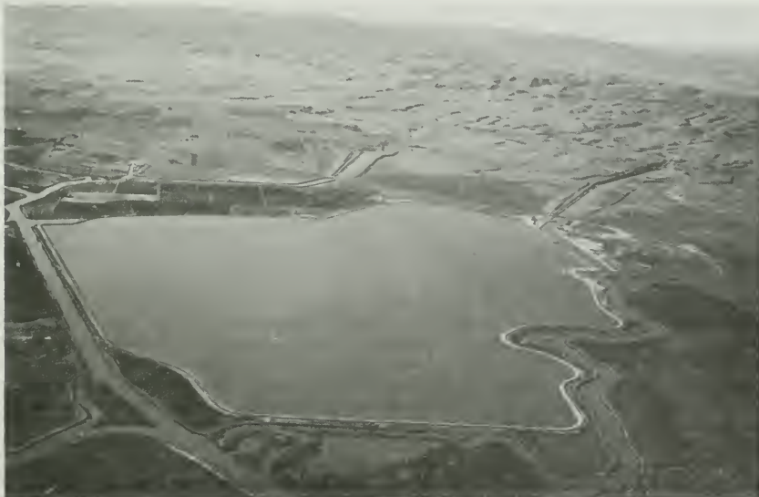
Figure 173. Aerial View—Clifton Court Forebay
