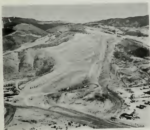
Figure 400. Spillway Stilling Basin and Chute Excavation
