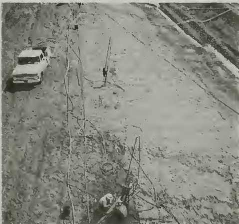
Figure 152. Grouting Foundation at Forebay Main Dam
