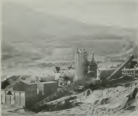
Figure 390. Soil-Cement Batch Plant
