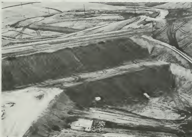
Figure 201. Bethony Forebay Dam Construction
