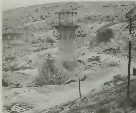
Figure 397. Low Intake Tower
