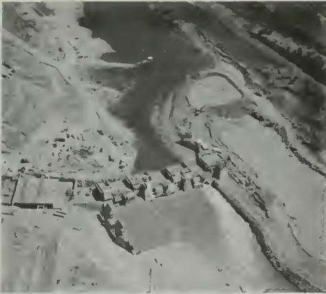
Figure 128. Cofferdam Closure
