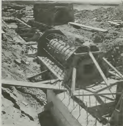
Figure 166. Pacific Gas and Electric Lateral Outlet Conduit
