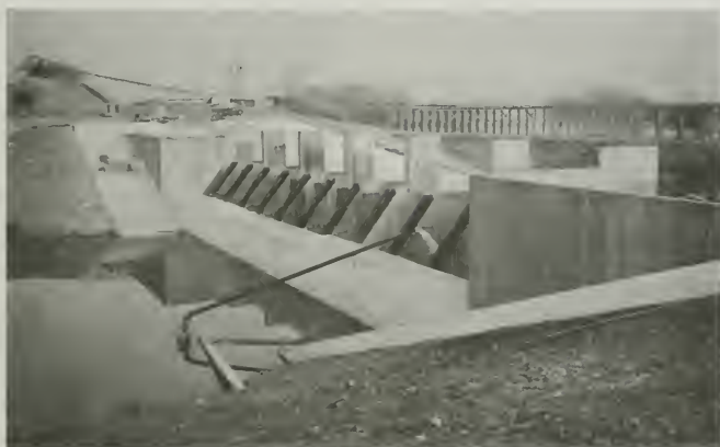
Figure 171. River Outlet—Fish Barrier Weir
