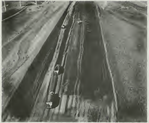
Figure 233. Placing and Compacting Embankment—San Luis Dam
