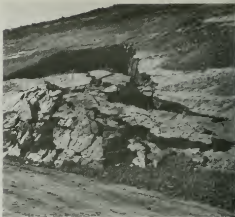
Figure 157. Slide at Left Side of Power Canal
