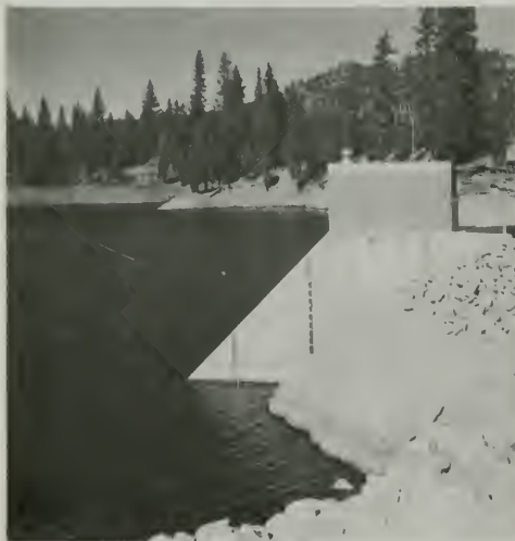
Figure 50. Control House at Dam Crest
