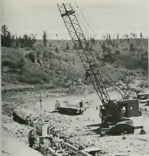
Figure 23. Outlet Works Concrete Placement
