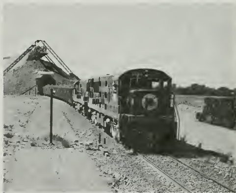
Figure 105. Pervious Loading Station
