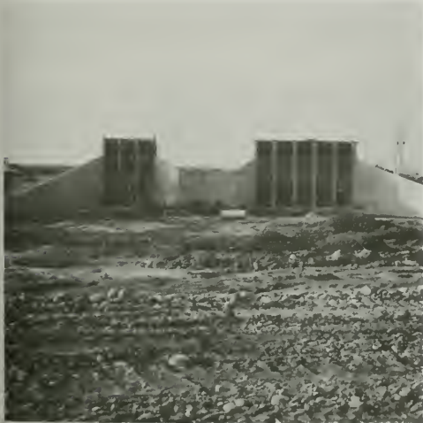
Figure 165. Western Canal and Richvale Canal Outlets—Upstream View
