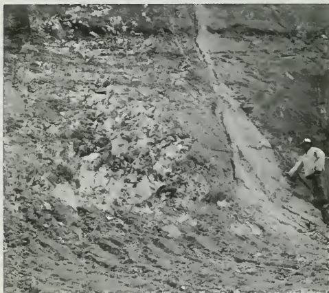
Figure 249. Fault Uncovered During Excavation
