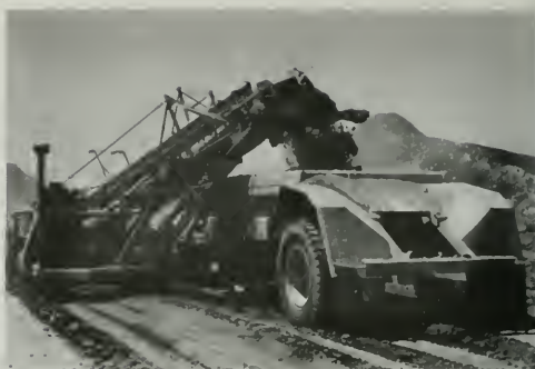
Figure 292. Excavation in Lake Borrow Area
