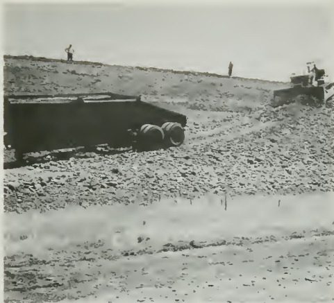
Figure 155. Placement of Zone 4A—Afterbay Dam
