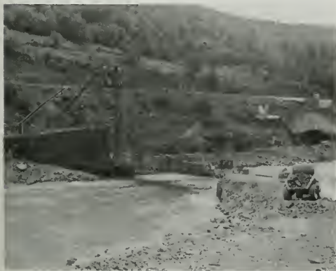
Figure 93. Diversion Tunnel No. 1 Intake Portal After Backfilling
