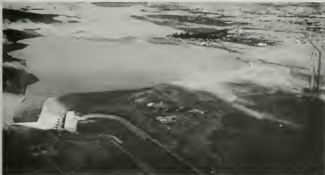
Figure 131. Aerial View—Thermalito Forebay
