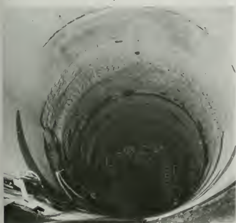
Figure 117. Wedge Seat Removal in Diversion Tunnels
