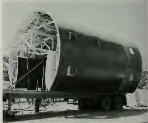
Figure 225. Tunnel Crown Placement Forms
