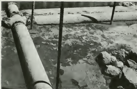
Figure 263. Perforated Drain Pipes in Spillway Chute
