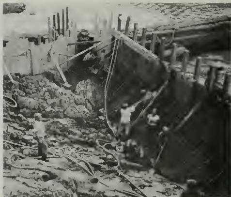
Figure 97. Wood Forms—Core Block
