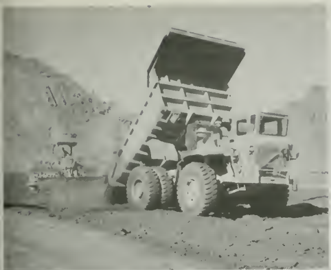
Figure 327. Dump Truck Used for Embankment Material Hauling
