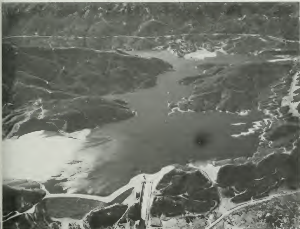
Figure 246. Aerial View—Cedar Springs Dam and Silverwood Lake
