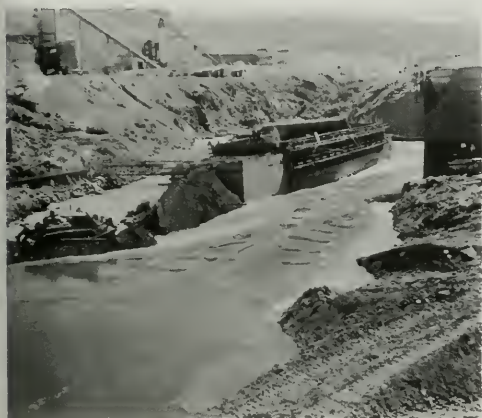
Figure 95. Stage 2 Diversion Earth Dike
