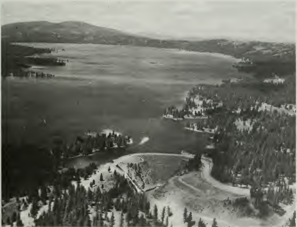
Figure 41. Aerial View—Grizzly Valley Dam and Lake Davis
