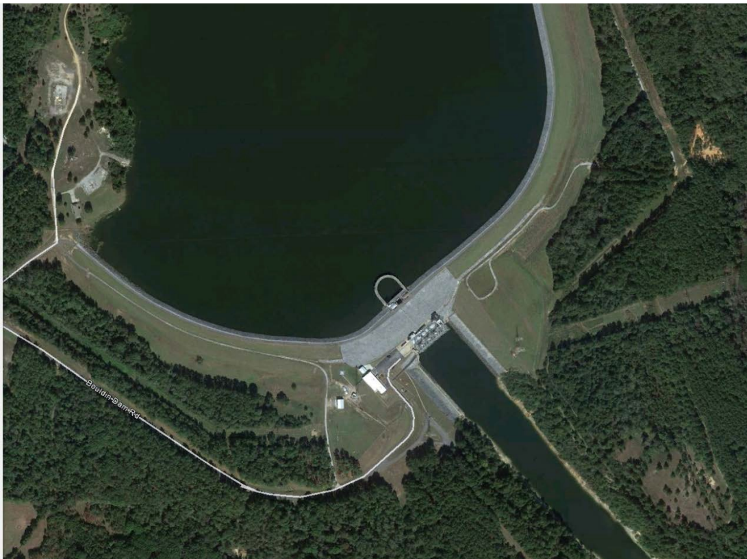
Figure 1.—Walter Bouldin Dam, intake, powerhouse, and tailrace canal (Google Earth, November 1, 2014).
