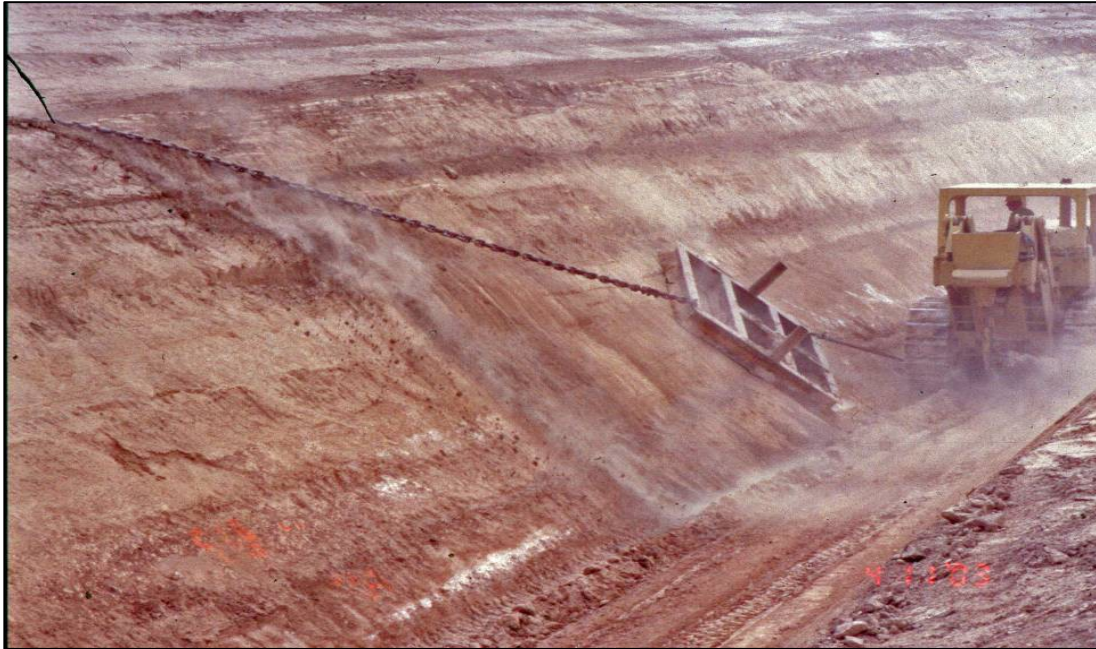
Figure 4.—Smoothing geotextile subgrade with metal frame, Olmitos-Garcias No. 2 Dam.
