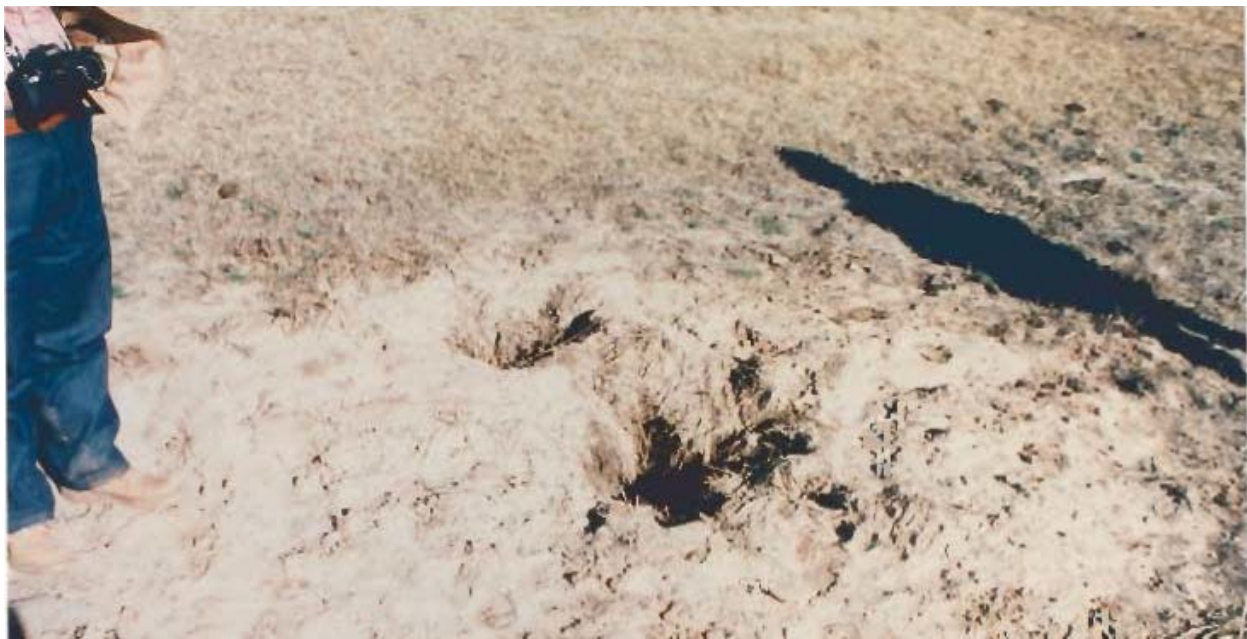
Figure 6.—Tunnel outlet downstream from Sta. 5+50, March 8, 1988.
