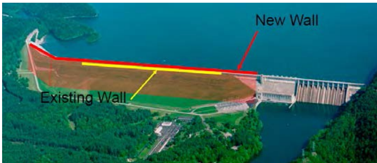
Figure 2.—Overall view of the dam showing extent of the existing and new cutoff walls.
