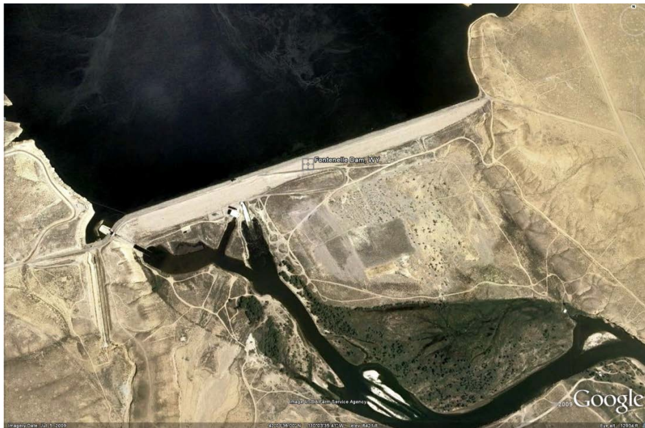
Figure 1.—Fontenelle Dam (Google Earth, July 5, 2009).
