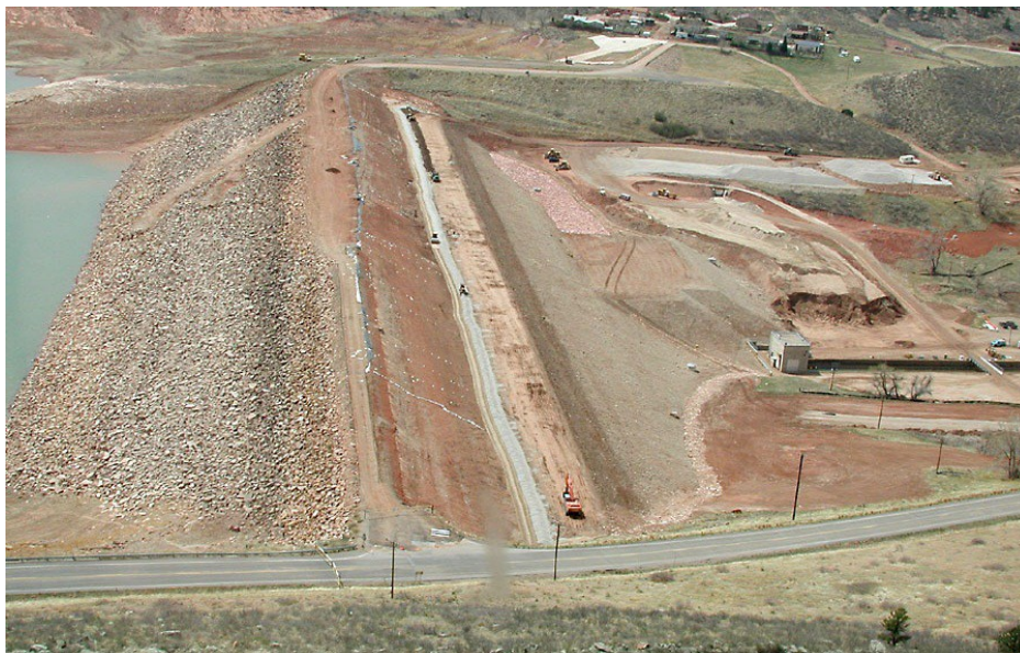
Figure 7.—Construction of downstream filter and berm at Horsetooth Dam.
