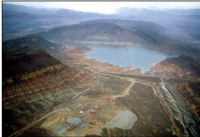
Figure 2.—The breach of the dike is located on the right limb of a large anticline where the rock outcrop extends beneath the dam in an upstream- downstream orientation.
