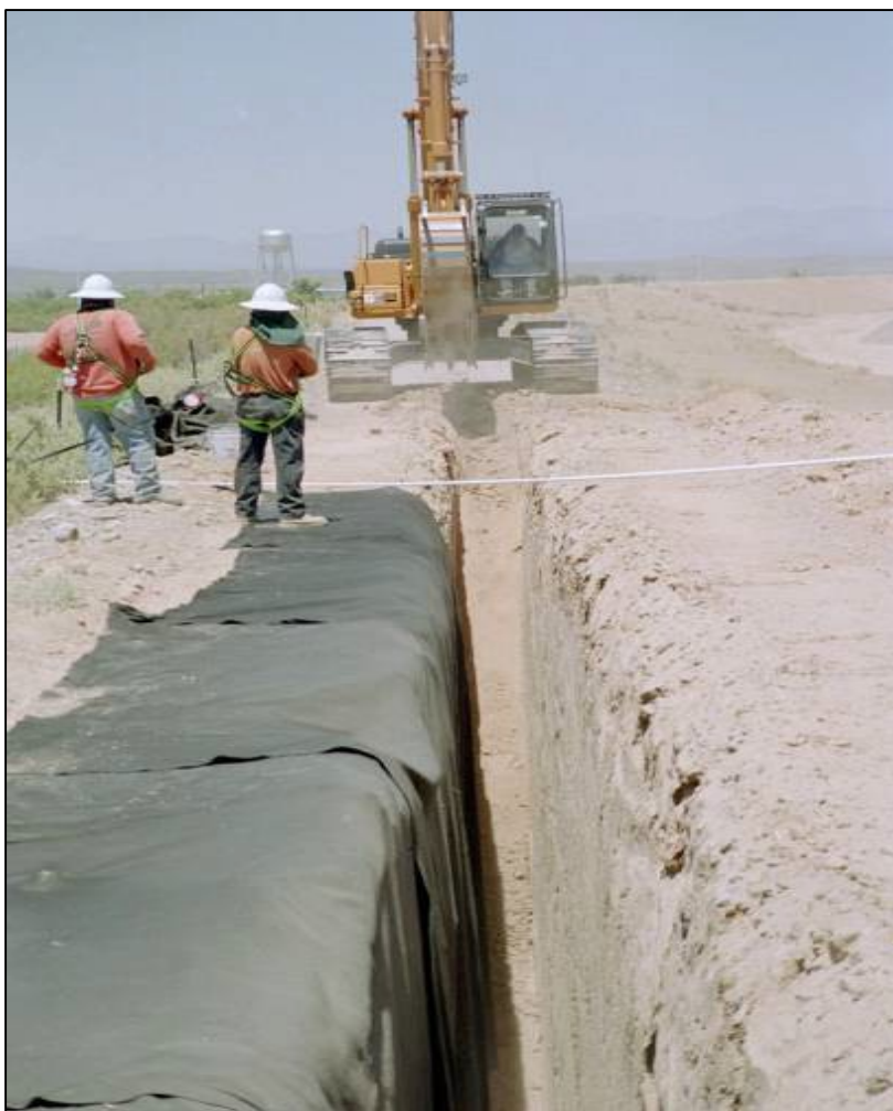
Figure 3.—Trenching and operation, Florence Dam.
