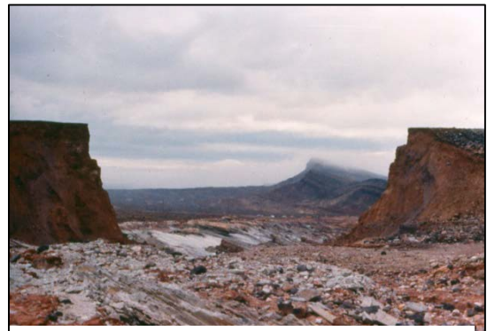
Figure 1b.—Breach through Quail Creek Dike.
