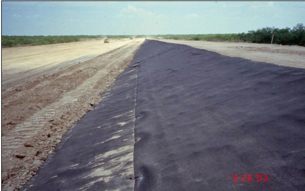
Figure 6.—Fill placement against geotextile, Olmitos-Garcias No. 2 Dam.
