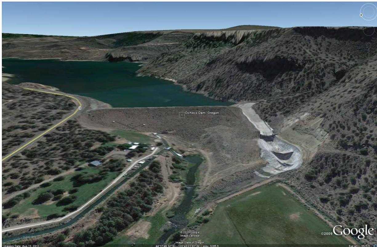
Figure 1.—Oblique view of Ochoco Dam, Oregon.
