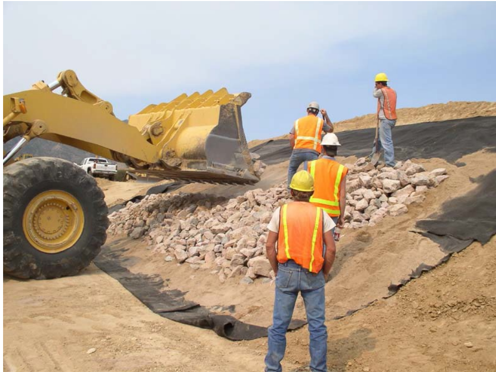
Figure 7.—Constructing the mockup.
