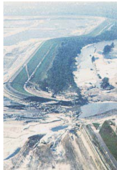
Figure 5.—Same area after breach.
