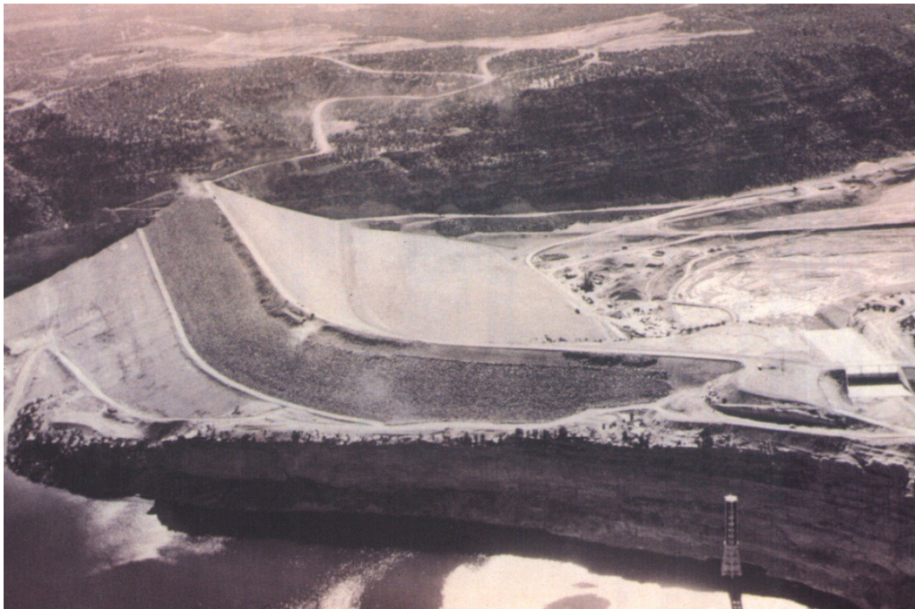
Figure 2.—Right abutment of Navajo Dam, looking downstream.
