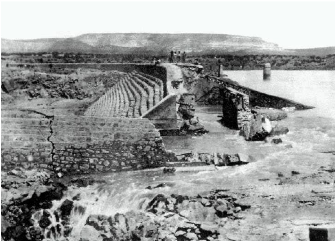
Figure 2.—Black Rock Dam near failure, 1909; spillway is in the foreground.
