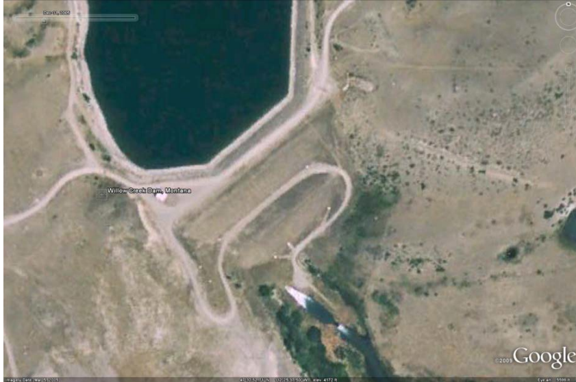
Figure 2.—Willow Creek Dam after 1996 and 2000 repairs (Google Earth, December 31, 2005).
