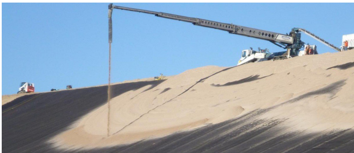
Figure 10.—Telebelt used from dam crest to protect geo-net composite.
