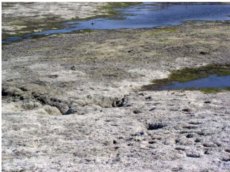
Figure 9.—Sinkholes in reservoir bottom.
