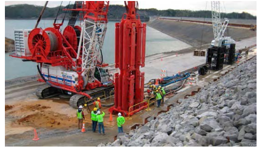
Figure 9.—View of hydromill construction.
