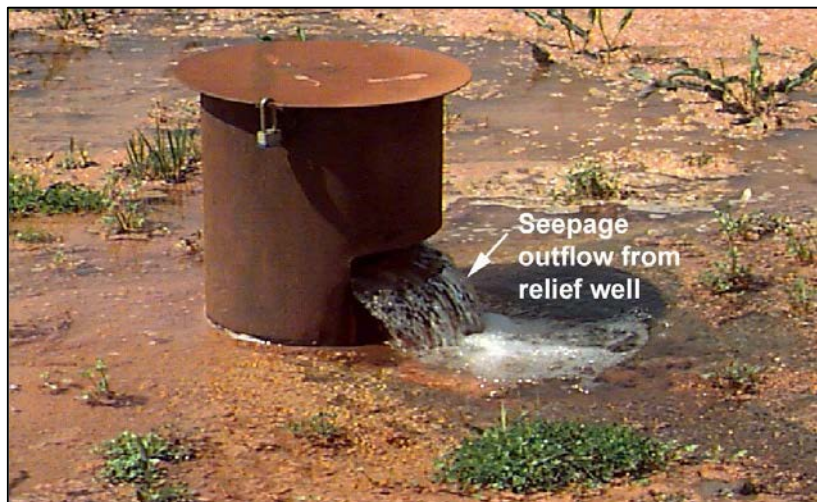
Figure 7-9.—Relief well seepage outflow. Although relief wells are not typically installed for the primary purpose of seepage water monitoring, their outflow can be collected, measured, and evaluated similar to open piezometers or observation wells.
