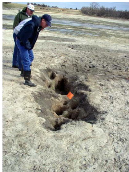
Figure 10.—Large sinkhole in reservoir.
