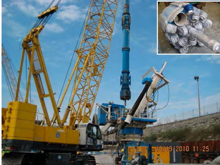
Figure 12.—Secant pile wall construction with reverse circulation drill.
