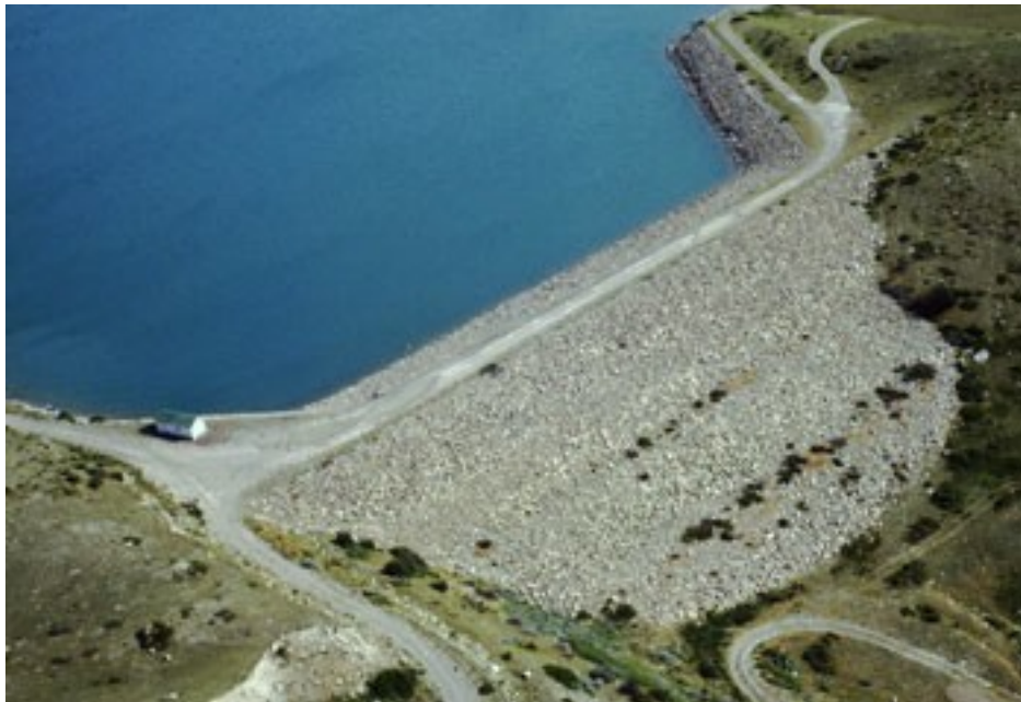
Figure 1.—Photograph of the Willow Creek Dam and gate house (Reclamation).
