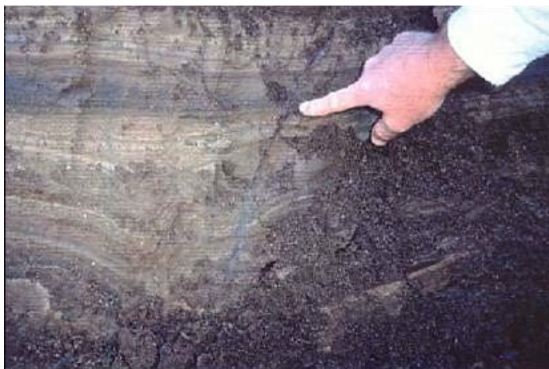
Figure 3-3.—Suspected hydraulic fracture at Ochoco Dam near the intake tower that was subsequently filled with reservoir sediments.
