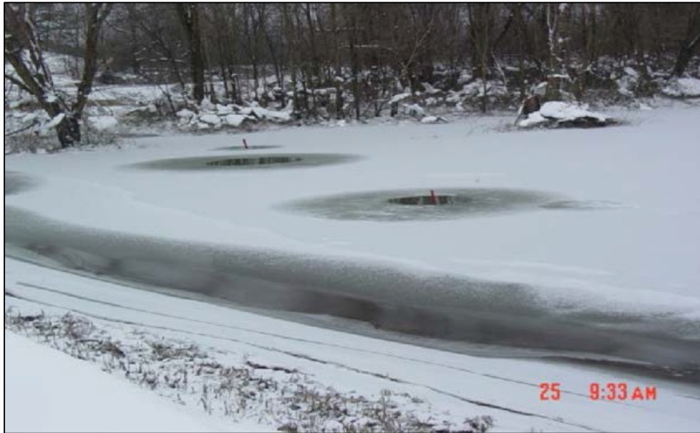
Figure 6-11.—Seepage water discharge locations (flagged with red markers) are more evident during the winter due to water temperature differences.
