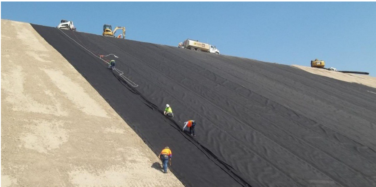
Figure 9.—Typical installation of geo-net composite on downstream face of embankment.
