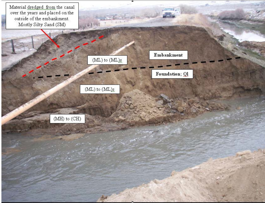
Figure 7.—Downstream view of the Truckee Canal breach. Dashed, black line is the approximate contact between the canal embankment and in-place lakebed deposits (Q1) composed primarily of silt with sand (ML)s and elastic silt (ML) with minor sandy lenses. Center-left is an abandoned Sierra Pacific Power gas pipeline.
