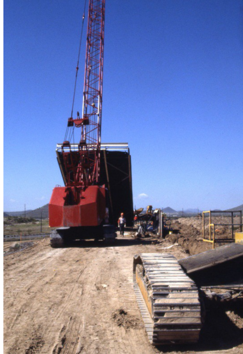
Figure 8.—Transport of geomembrane panel by crane using steel frame.
