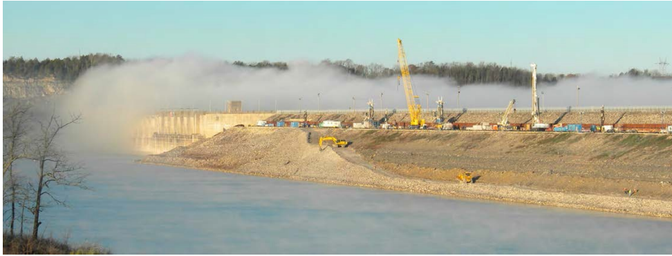
Figure 6.—View of working platform on upstream slope.
