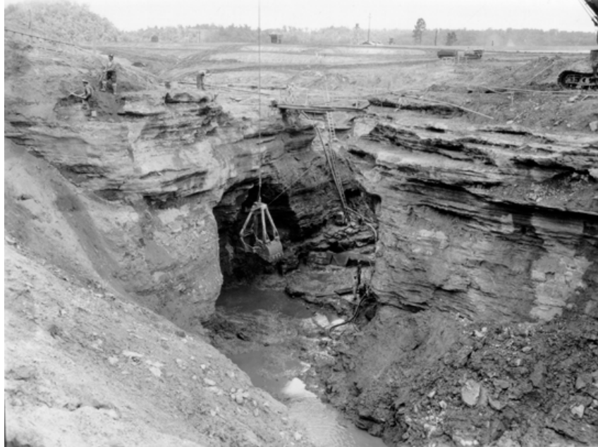
Figure 3.—View of solution feature in cutoff trench excavation.
