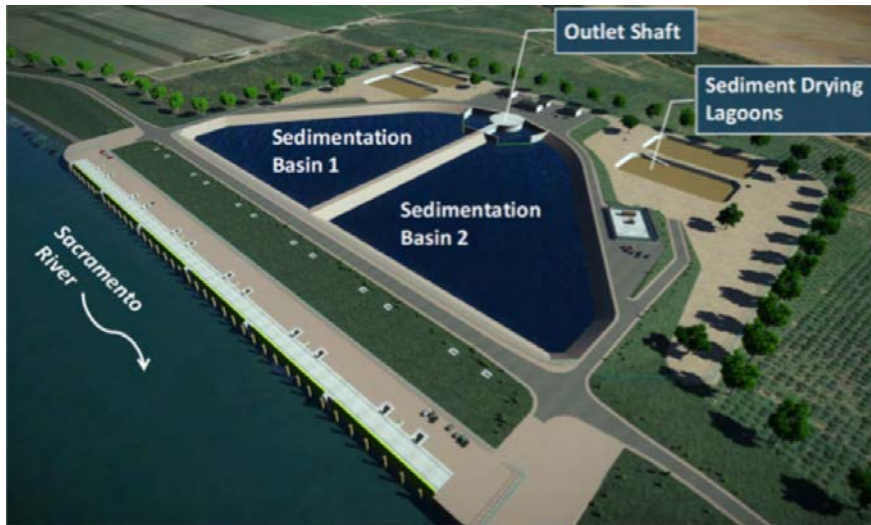
Figure 4: Sacramento River intakes
