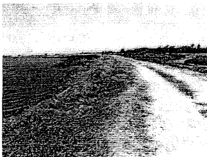
Low freeboard, easily overtopped Delta levee
