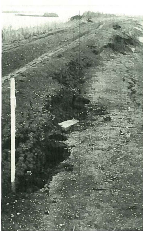
Cracks occurring on the levees of a low-lying island.
