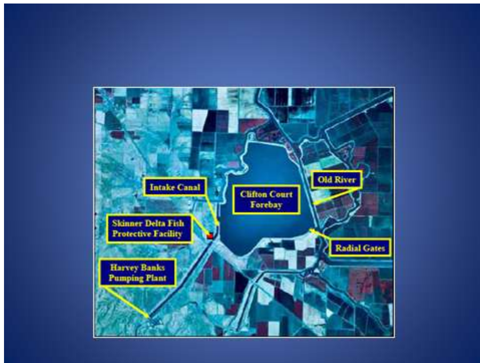
Figure 9-18. Clifton Court Forebay.
