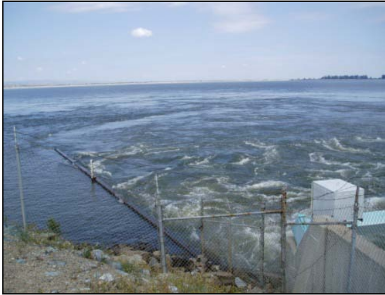
Figure 54. Clifton Court Forebay showing turbulence behind the radial gates. Photo by Dave Vogel.
