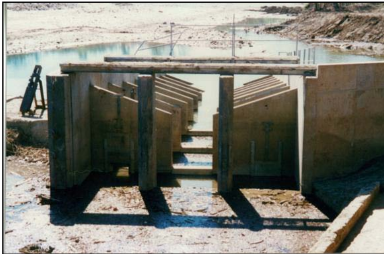
Figure 15. New fish ladder constructed on Butte Creek. Photo by Dave Vogel.
