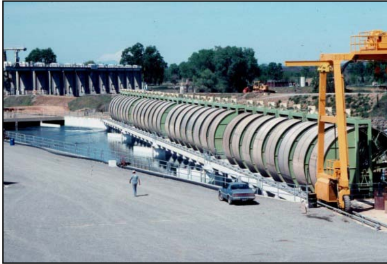
Figure 36. State-of-the-art angled rotary drum screens installed at the headworks to the Tehama-Colusa Canal and Corning Canal at RBDD in 1990. Photo by Dave Vogel.
