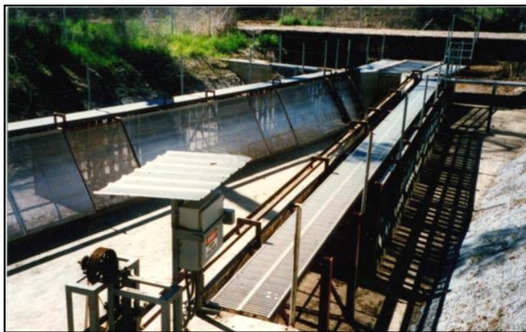
Figure 27. New fish screens constructed on Butte Creek. Photo by Dave Vogel.
