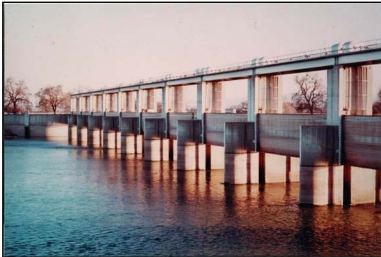
Figure 12. Red Bluff Diversion Dam with all 11 dam gates raised to provide unimpeded upstream and downstream fish passage. Photo by Dave Vogel.
