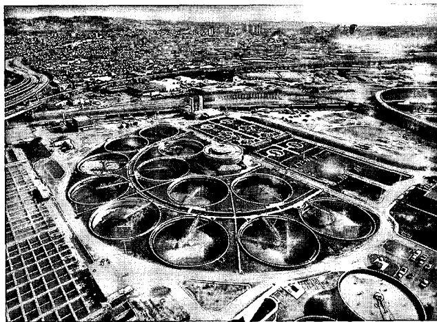
More than 50 municipal wastewater treatment plants, like this one operated by the East Bay Municipal Utility District, discharge to the estuary a combined daily average of 855 million gallons of treated effluent. (Photo: courtesy, EBMUD)
