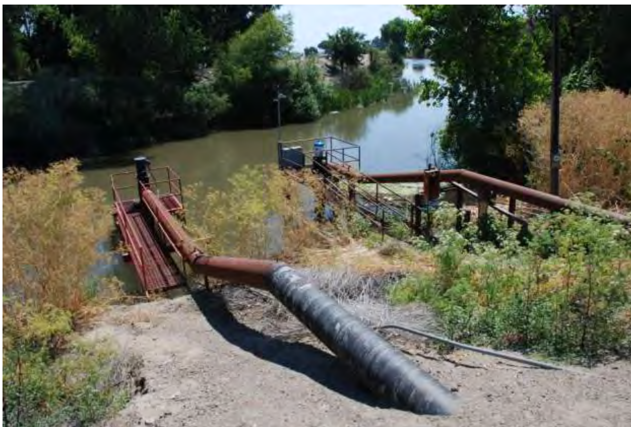
Photo 2. Typical Pump Diversions
