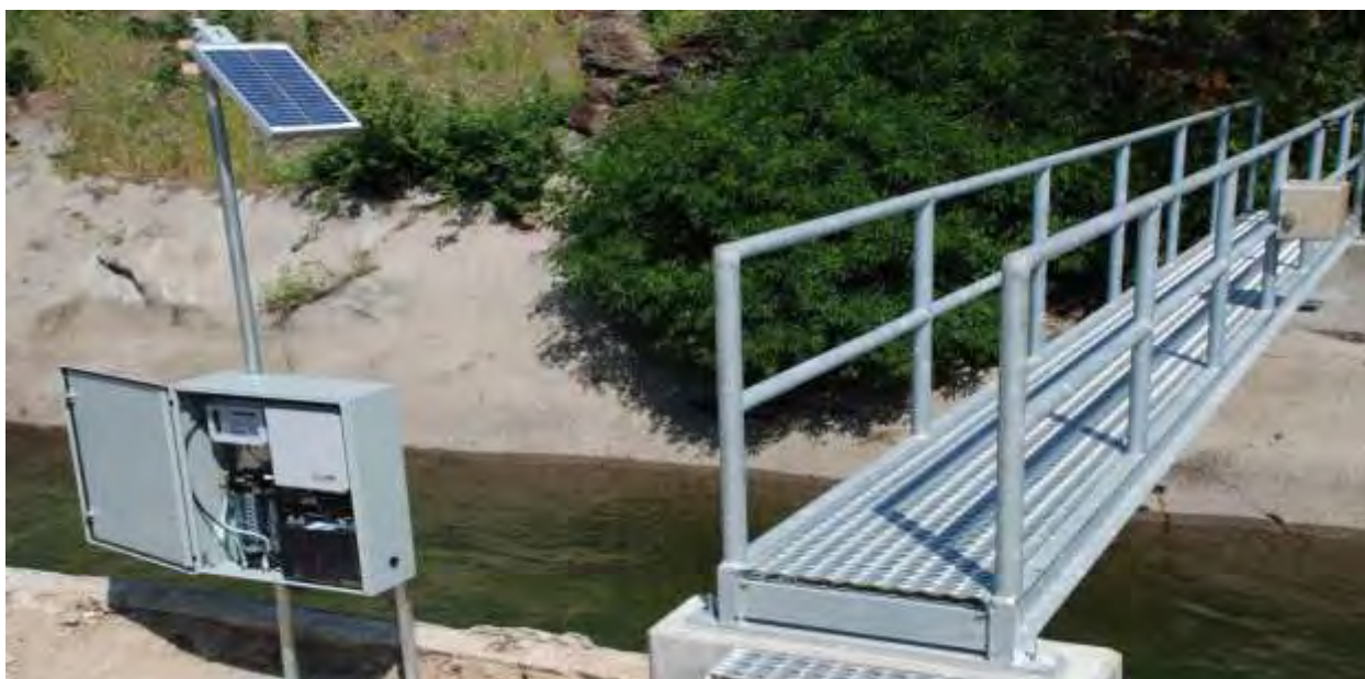
Photo 5. Typical Gaging Station and Measuring Bridge Over Irrigation Canal
