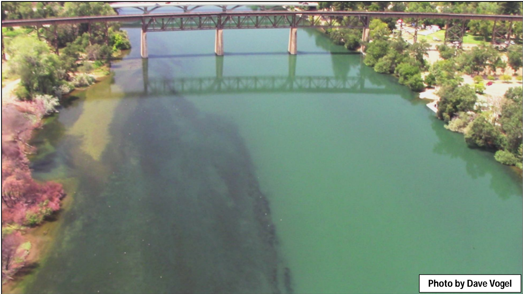
Sacramento River looking upstream from ACID Dam
