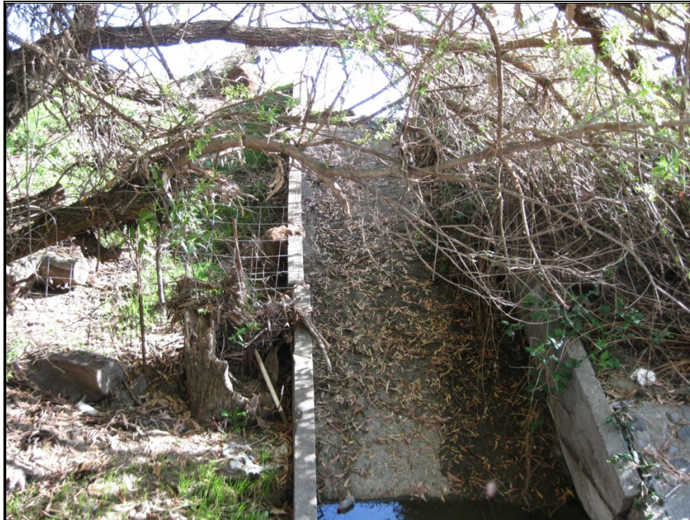
Photo 2 - View of upstream reservoir (D032167) spillway
