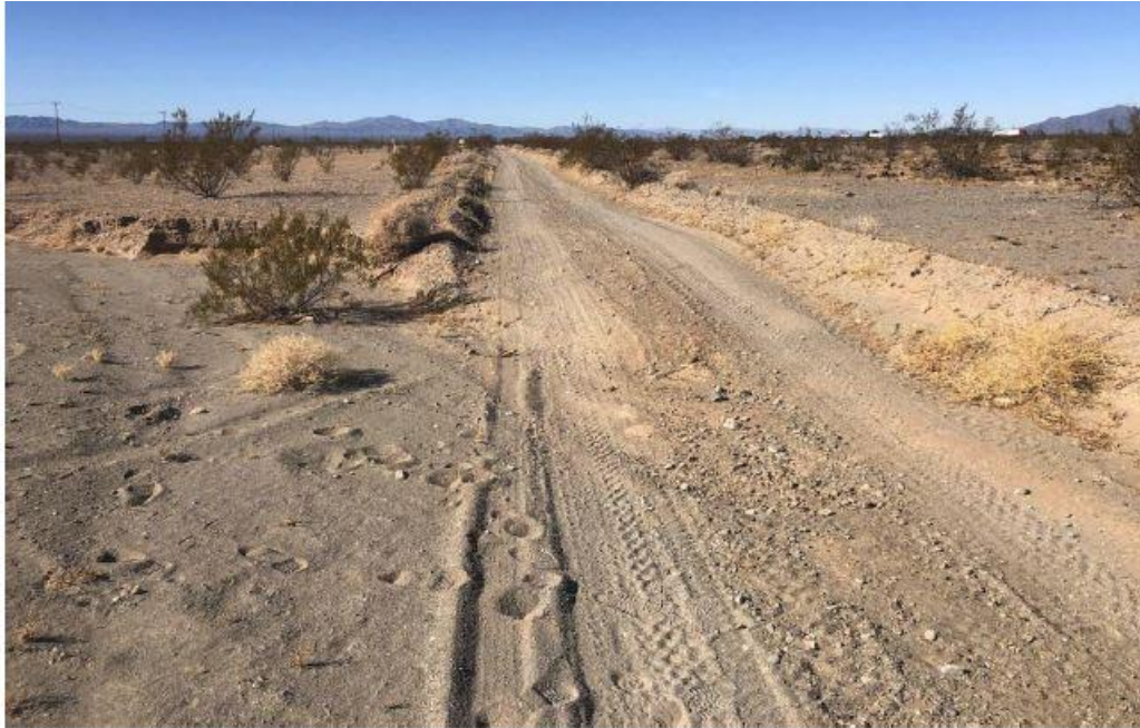
Photograph 3: Representative drainage crossing a dirt road in the Project area (Rincon Consultants, Inc. 2021b 8 ).
