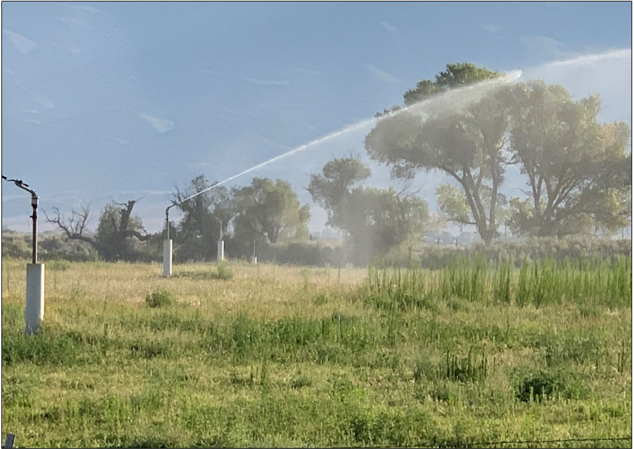
Figure 7.2- BAWA is considering installing on its Department-acquired land a fixed in-ground sprinkler irrigation system to irrigate improved pastureland. This photograph is of a property adjacent to the BAWA wastewater treatment plants showing a similar irrigation system planned for BAWA land.
