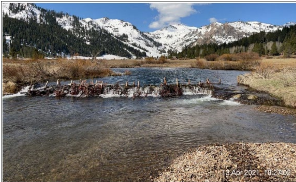
Figure 5.3 - Artificial beaver dam slowing and dispersing water so sediment can settle, and erosion is decreased
