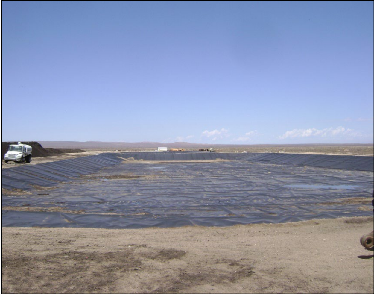
Figure 8.6 - Photo location no. 4, view of one of the onsite lined surface impoundments. All runoff from the site is directed to the surface impoundments for evaporation.
