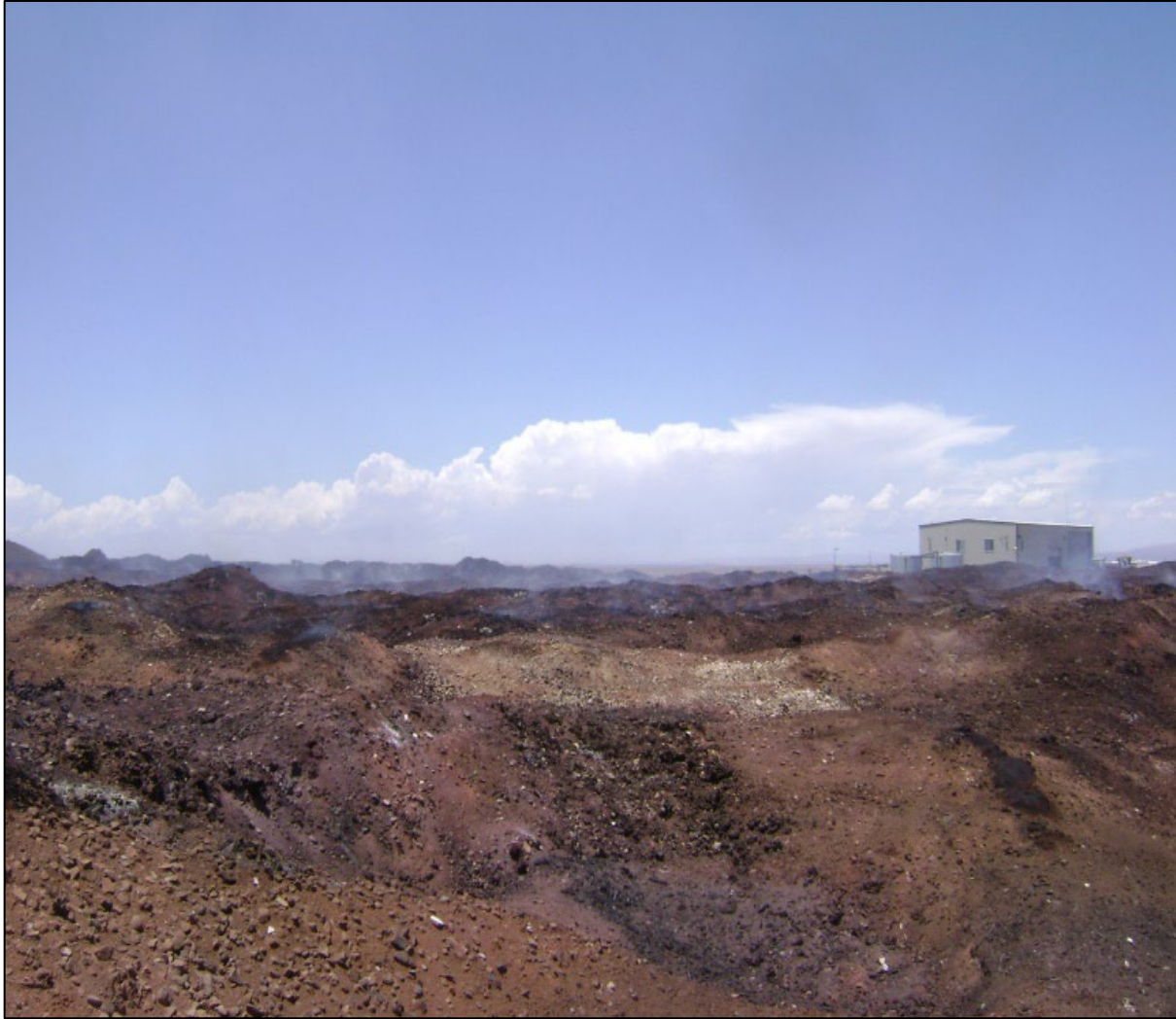
Figure 8.4 - Photo location no. 1, view of smoldering material in the northeastern portion of the site. The material was oxidized from the heat of the fire and excessive internal temperatures of the material.
