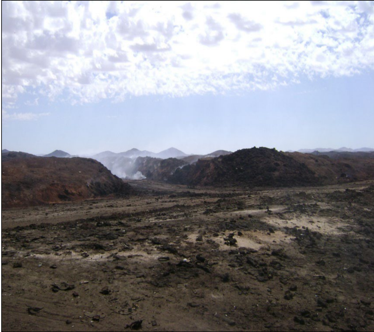
Figure 8.3 - Photo location no. 2, view of smoldering material along the western portion of the site. The windrows are more apparent in this portion of the site, though the heights vary due to heavy equipment frequently turning and tilling the piles.
