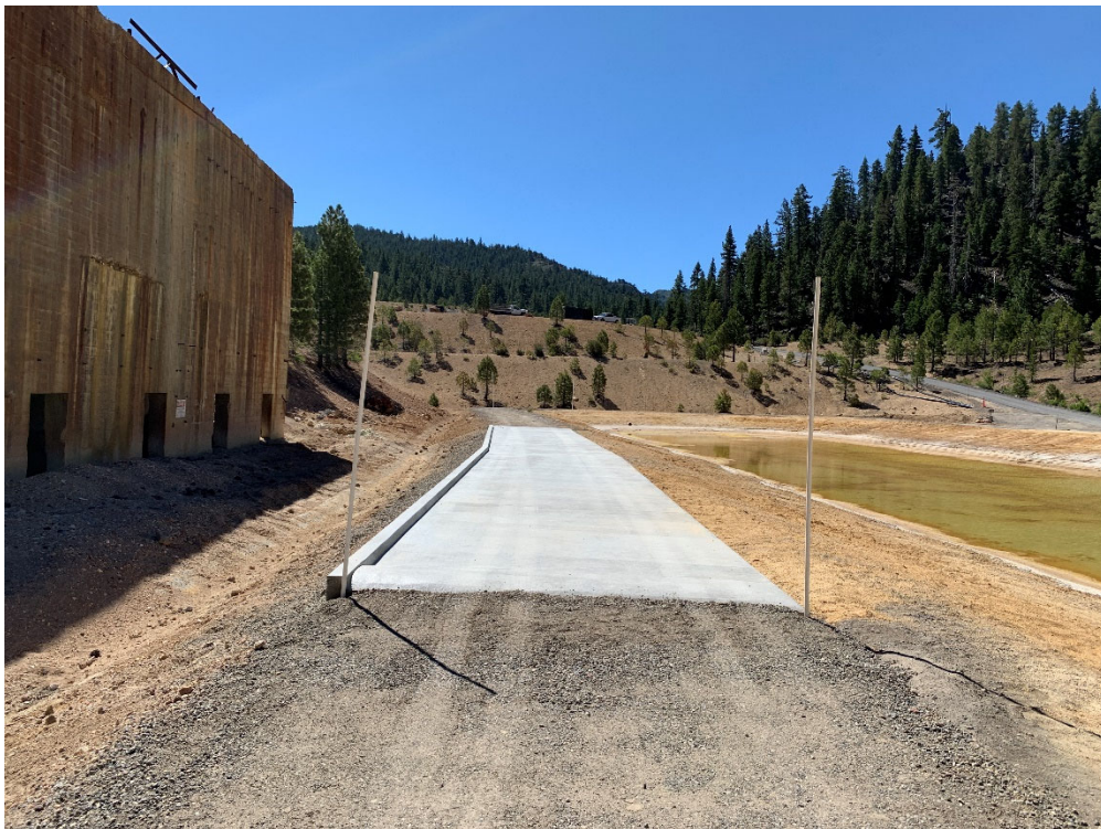
Photo 6 – June 29, 2022, Concrete pad constructed at Pond 3 for winter/spring treatment activities.
