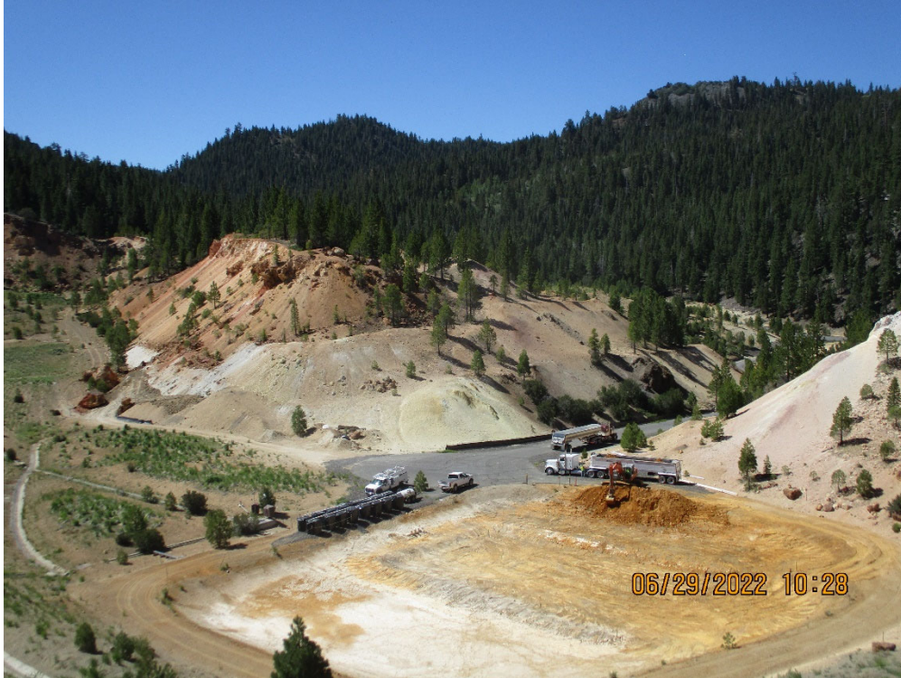
Photo 1 – June 29, 2022, Sludge stockpile and disposal activities at the pit clarifier.
