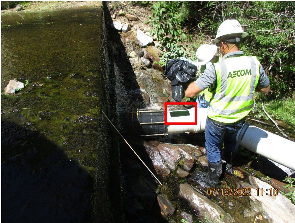
Photo 3 – June 13, 2022, Access port for video inspection of the Channel Underdrain (CUD).
