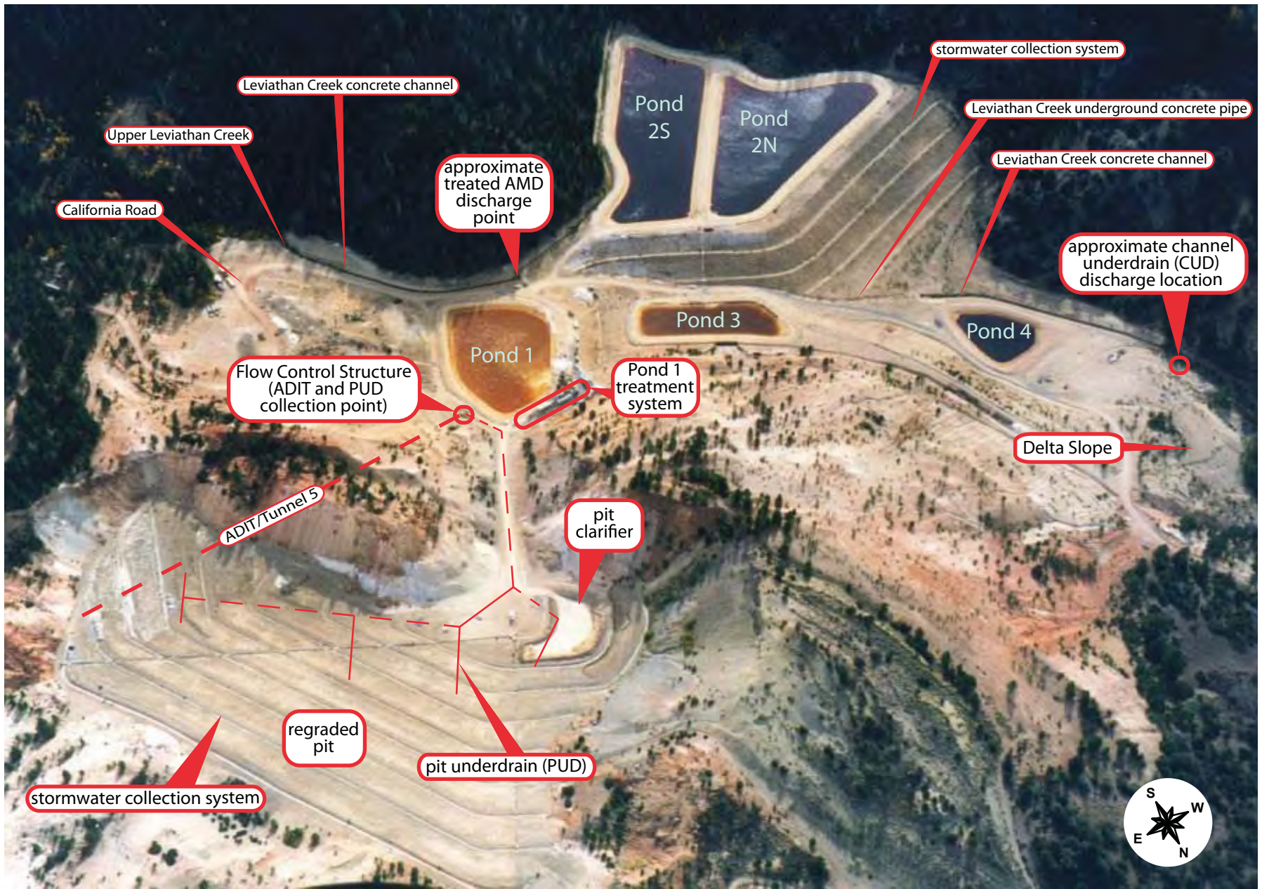
FIGURE 3 LAHONTAN WATER BOARD AMD CAPTURE AND TREATMENT SYSTEM
